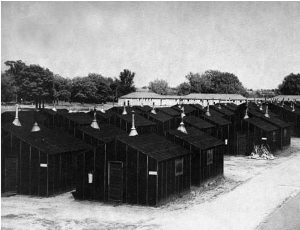
Temporary barracks known as the Turkey Farm
