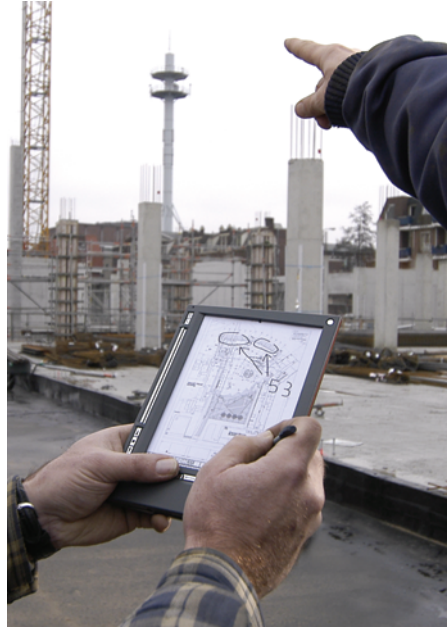
Figure 2.19. With eReaders, forms can be input with a significant advantage in size, weight and cost (compared to a laptop).
