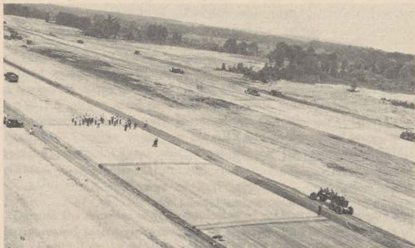
Figure 7. Army engineer troops placing T-17 membrane on soil surface of an airfield runway in Vietnam.
