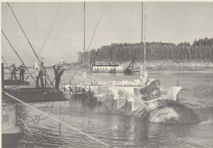
Figure 11. Salvaging a 356-ton tank of liquid chlorine from the Mississippi mud.
