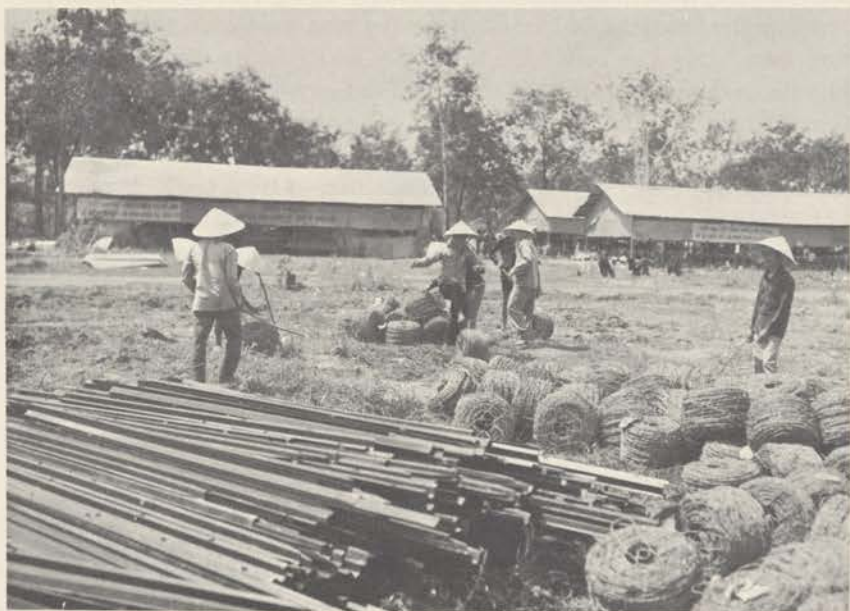
Figure 1. Wire and steel posts for protective fencing around a strategic hamlet, Vietnam.
