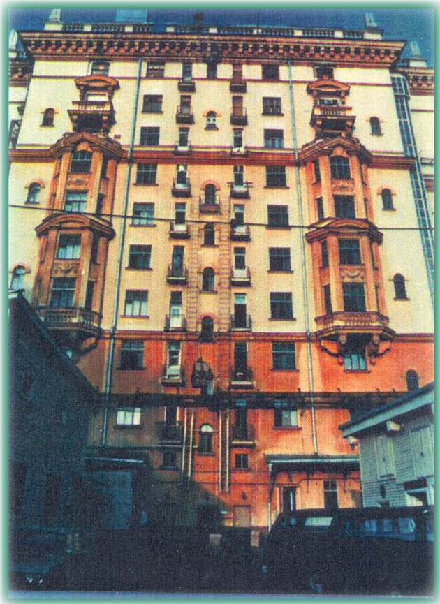
Fig. 1. U.S. embassy in Moscow. Equipment was lifted in and out of this building, possibly from the roof, since the Soviets had shut down the elevator.
