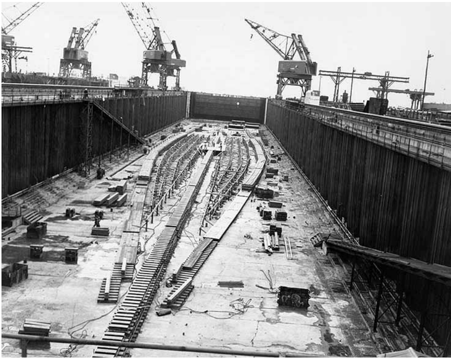
Keel plate laid for USS United States (CVA-58) at the Newport News Shipbuilding and Dry Dock Company shipyard, Newport News, Virginia, 18 April 1949. Five days later, on 23 April, Secretary of Defense Johnson cancelled the carrier.
