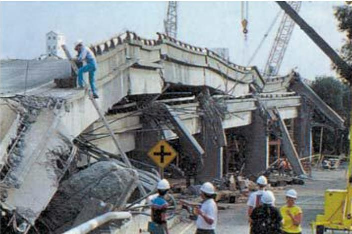
The Cypress Freeway structure in Oakland was built in the 1950s, before the use of modern seismic safety standards. Part of the structure standing on soft mud collapsed in the magnitude 6.9 Loma Prieta earthquake in 1989. Adjacent parts of the structure that were built on firmer ground remained standing.
