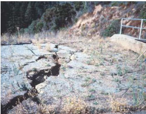
Cracks in the top of this earthen dam were caused by the 1989 magnitude 6.9 Loma Prieta earthquake.
