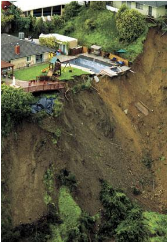
The hillside beneath a home gave way following the magnitude 6.7 Northridge earthquake in 1994.
