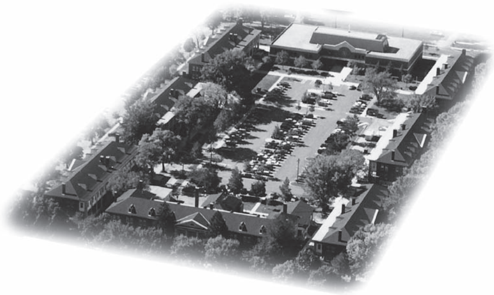
DAU's New Fort Belvoir, Virginia, Campus
