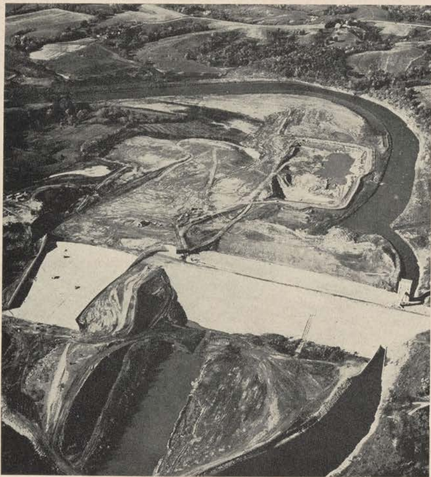
Figure 17. Aerial view of Coralville Dam work.
