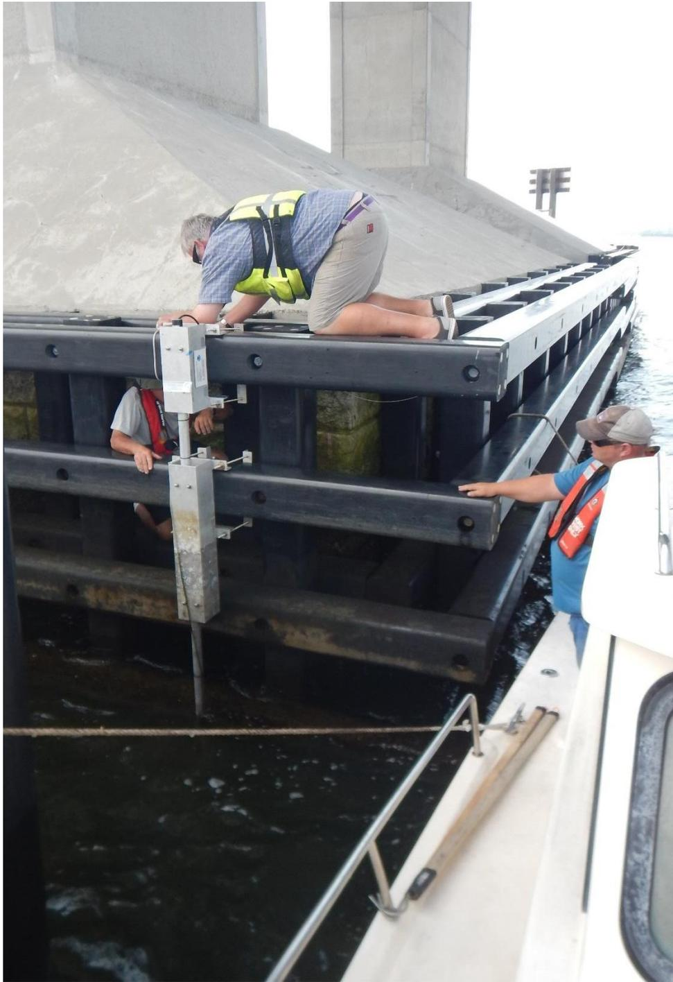
**Figure 3-4.** Horizontal crib mount being installed. ADCP is held at the bottom of the pole, below the surface.
