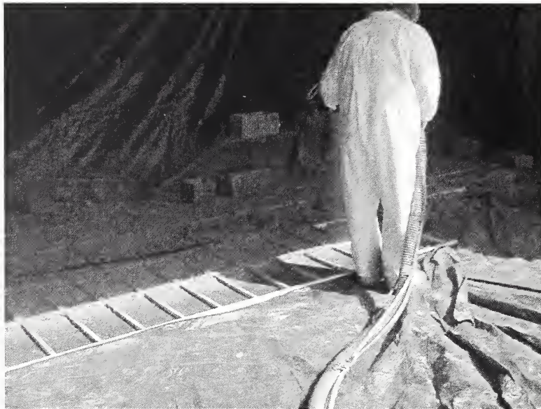
Figure 7–5. Spraying steel plates with BLAZE-SHIELD DC/F.
