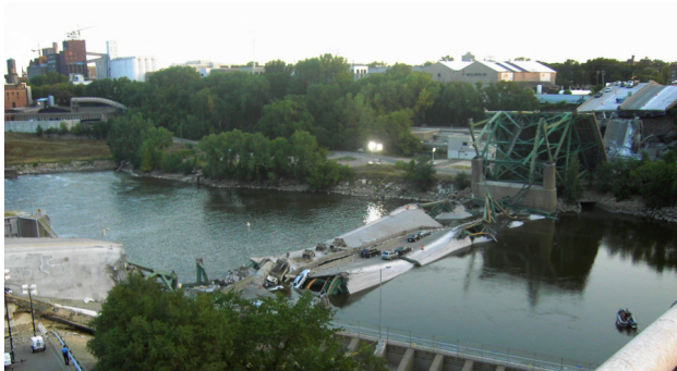
Figure 10. The I-35W Mississippi River Bridge collapsed in 2007 as a result of a design flaw. It carried appx. 140,000 vehicles per day. Source: Mike Wills, Flickr
