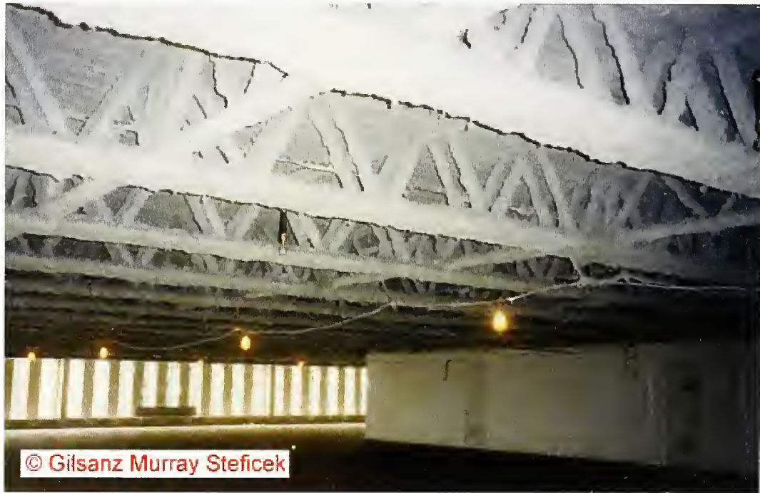
Figure 1–8. Photograph of insulated WTC trusses.
