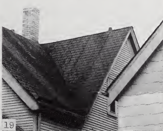
FIGURES 14 to 19.— Mineral-surfaced, asphalt-prepared roll roofings.
