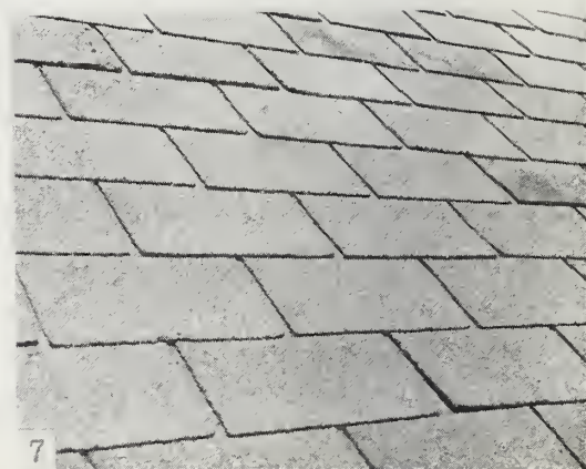
FIGURES 2 to 7.— Asphalt shingles (individual shingles applied by the American method).
