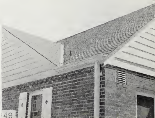
FIGURES 44 to 49.— Metal roof, flashings, and valleys
