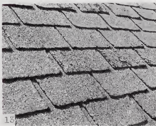
FIGURES 8 to 13.—Asphalt shingles (individual shingles applied by the American method).
