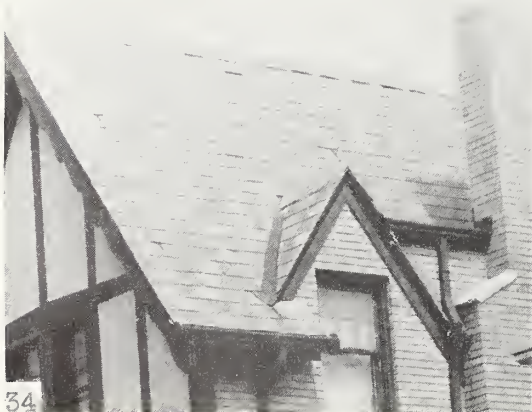
FIGURES 32 to 37.—Cement-asbestos shingles and slate.
