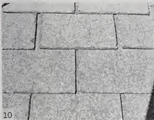
FIGURES 8 to 13.—Asphalt shingles (individual shingles applied by the American method).
