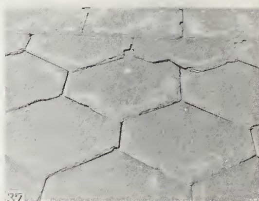
FIGURES 32 to 37.—Cement-asbestos shingles and slate.
