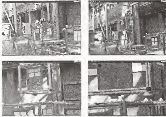
Figure 6. Robotized crane assembling a module.
