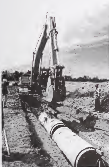
b) Laying Pipe with PipeMan
