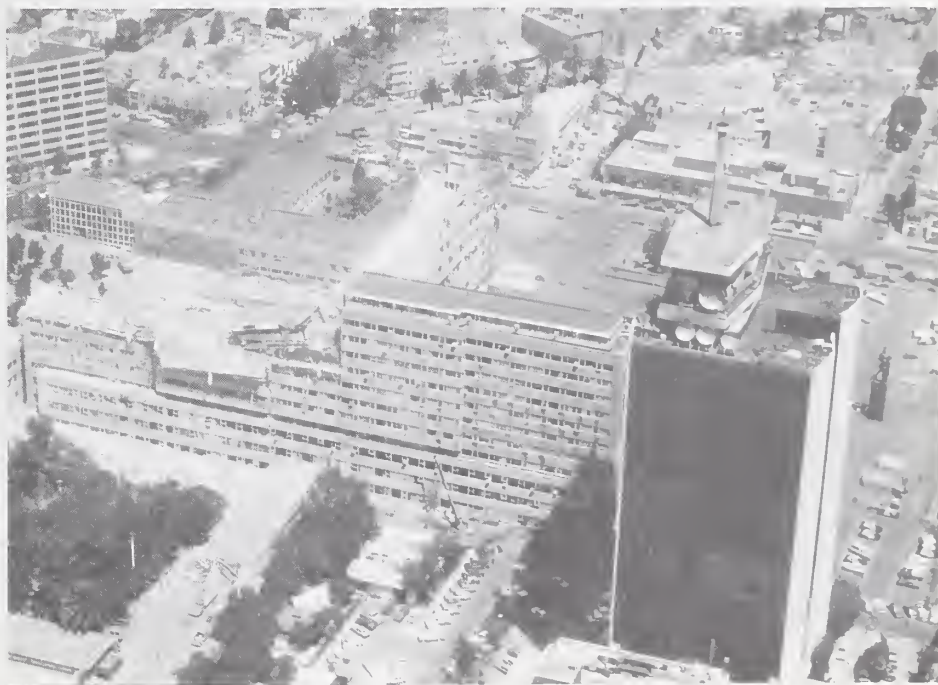
(b) Aerial view looking southwest.
