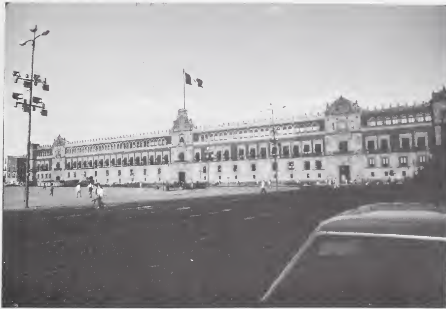
Figure 5.70. Colonial stone masonry structures (National Palace and Cathedral) have short natural periods of vibration and performed well in the earthquake.
