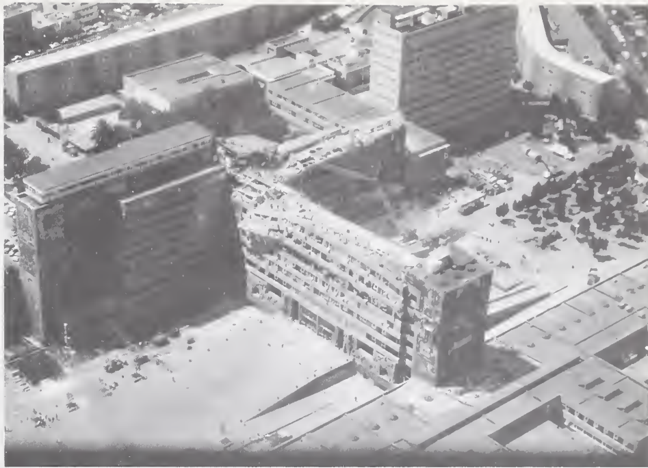
(a) Aerial view looking north.
