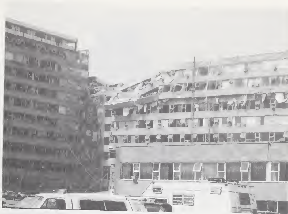
(a) East side of SCT Building.
