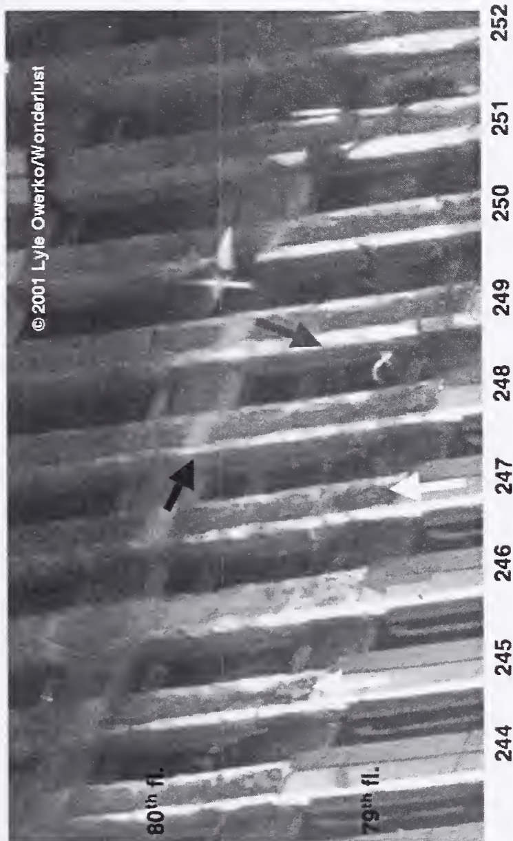
Figure 2-34. Image of missing sprayed fire-resistant material on flanges of exterior columns of N face of WTC 2. Sprayed fire-resistant material has come off, revealing red Tnemec paint of the column (red arrows). This image also shows how the outer web regions have been partially or completely denuded of sprayed fire-resistant material. Damage is evidenced by shading by sunlight - compare green (undamaged sprayed fire-resistant material) and white (damaged sprayed fire-resistant material) arrows. Blue arrow indicates same type of white coated area of sprayed fire-resistant material as previous figure that adhered when material above and below was dislodged.
