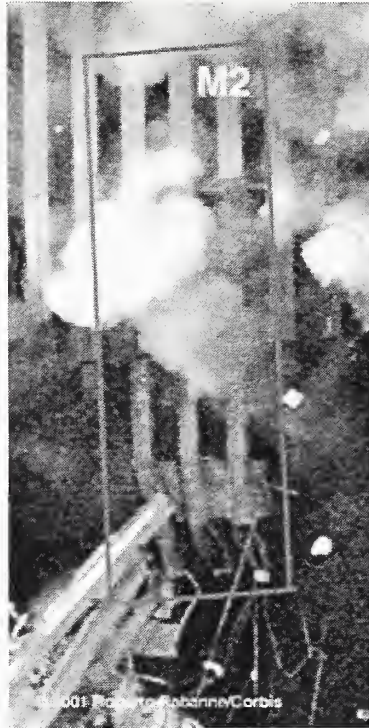
Figure 2–17. Close-up of pre-collapse condition of panel M-2 (A130: 96-99).
