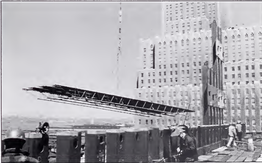
Figure 1-6. a) Construction photograph of a composite floor truss.
