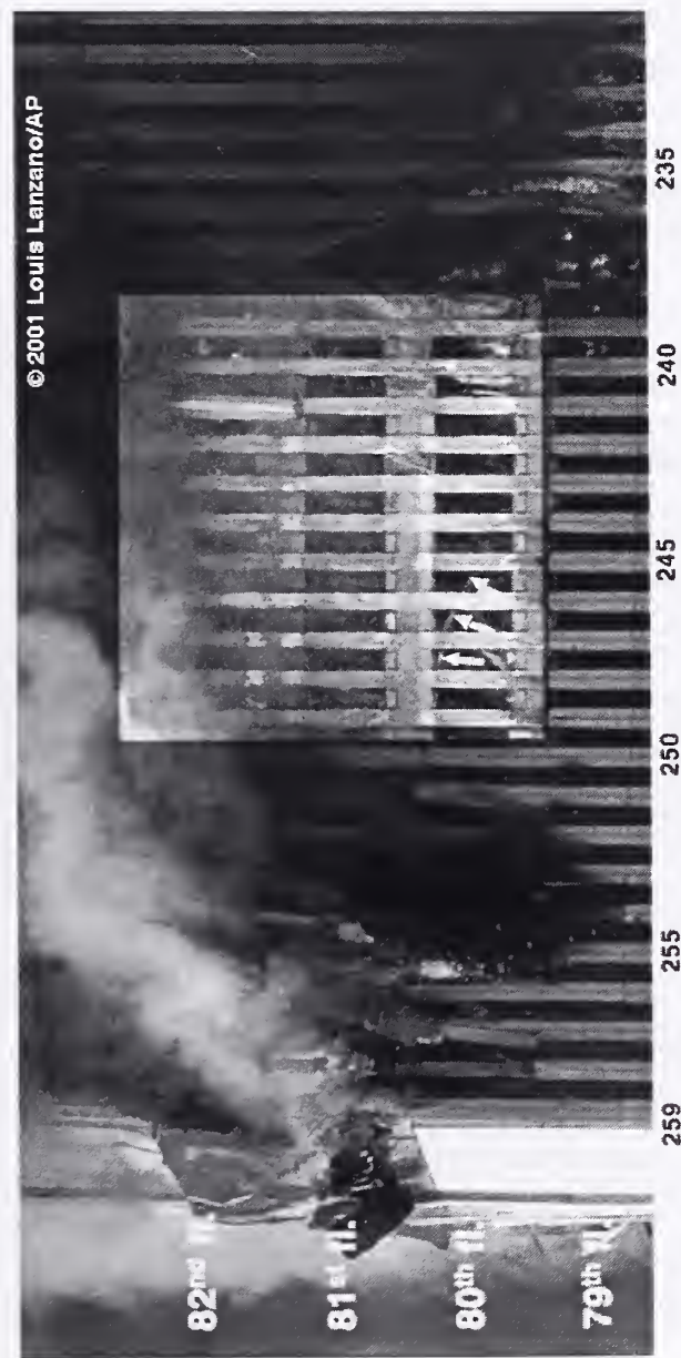
Figure 2-42. Image of dropped floor on north face of WTC 2. The slab of the 81st floor has dropped into the office space of the 80th floor.
