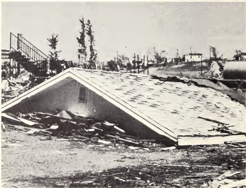
Carport roof of a large motel in Lubbock, Texas, was lifted completely from its supports, moved approximately 40 feet, and set down intact by a tornado. The remainder of this motel was demolished.
