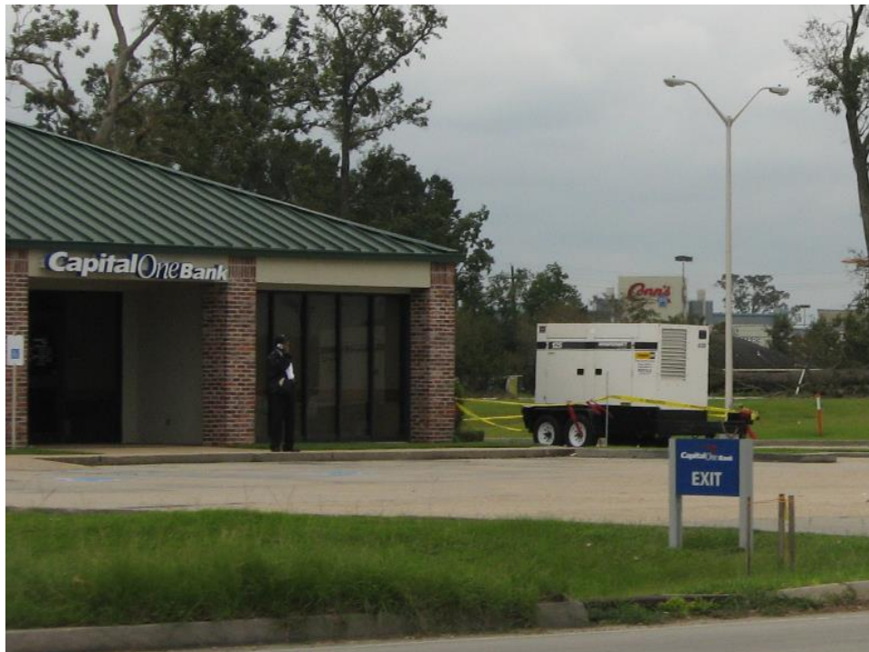
Figure 9. A mobile diesel generator powering a bank office south of Baton Rouge, LA after Hurricane Gustav.
