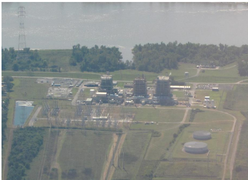
Figure 7. Little Gypsy power plant in Laplace, LA. This power plant is primarily fueled by natural gas, but it also accepts oil as fuel. Oil storage tanks are seen on the bottom right corner of this photograph.
