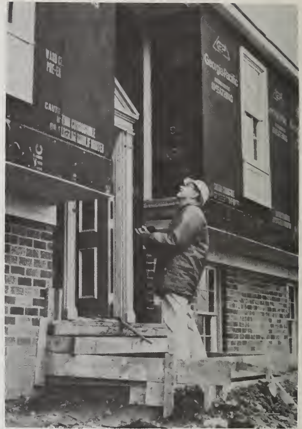
CBT technical data provides a basis for building code provisions.
