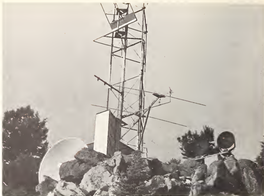
Mountain-top transmitting location for studies of fading characteristics in wide-band transmission systems. Receivers are located at a distance of 70 miles on the plains within the line-of-sight. Problems of space telecommunications have led to a need for more data on long line-of-sight transmission paths (page 128).
