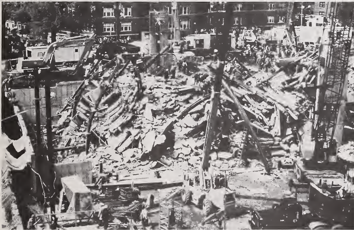
The failure of a key component of the system for lifting concrete floor slabs was the most probable cause of the L'Ambiance Plaza building collapse on April 23, 1987.
