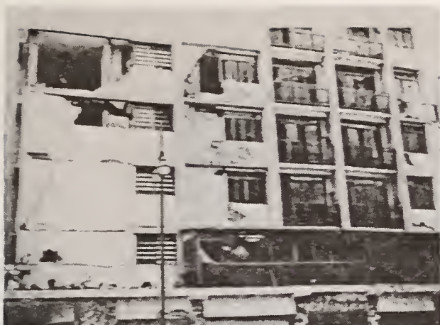
Fig. 10—Damage to brittle hollow clay tile infill in Caracas, 1967
