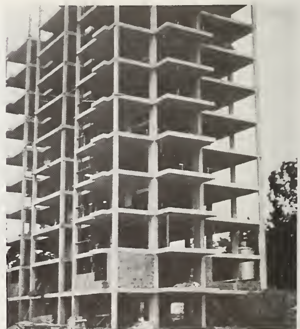
Fig. 9—Typical skeleton of a multi-story building in Caracas, Venezuela
