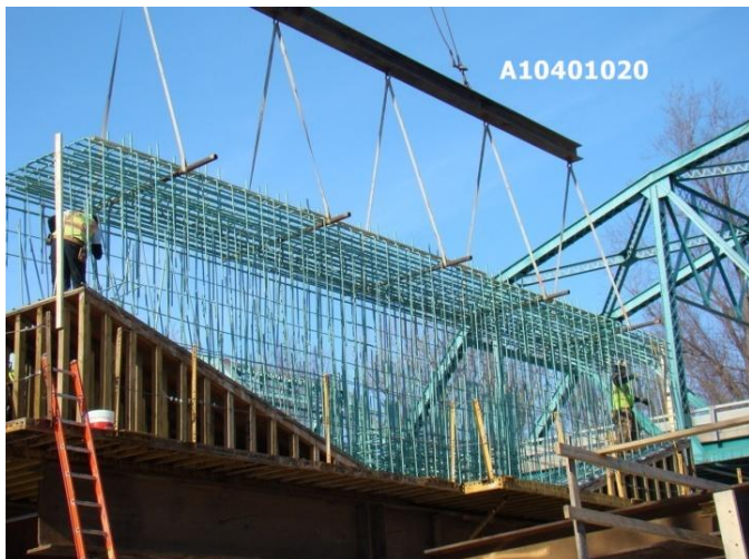
Figure B.9 Individual Elements: A1040 Cap Beams (Sub-Elements: A10401020 Reinforcement)
