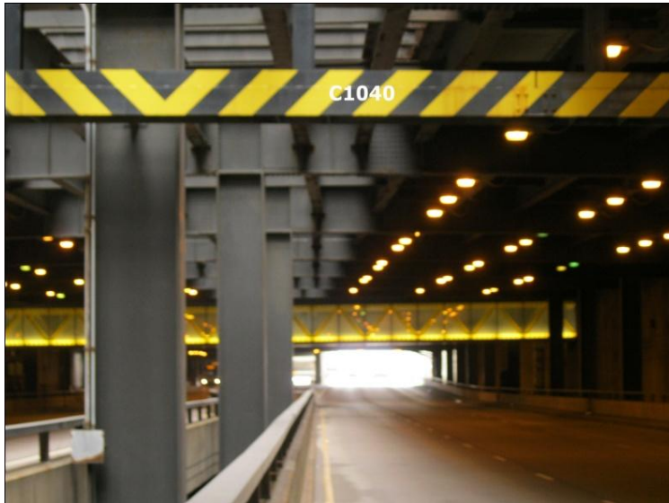
Figure B.37 Individual Elements: C1040 Sacrificial Beams
