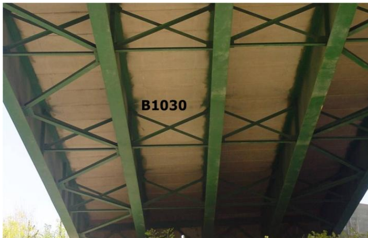
Figure B.23 Individual Elements: B1030 Bracings
