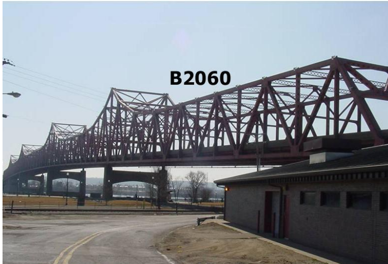
Figure B.30 Individual Elements: B2060 Truss Members
