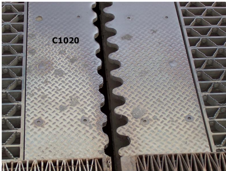
Figure B.35 Individual Elements: C1020 Expansion Joints
