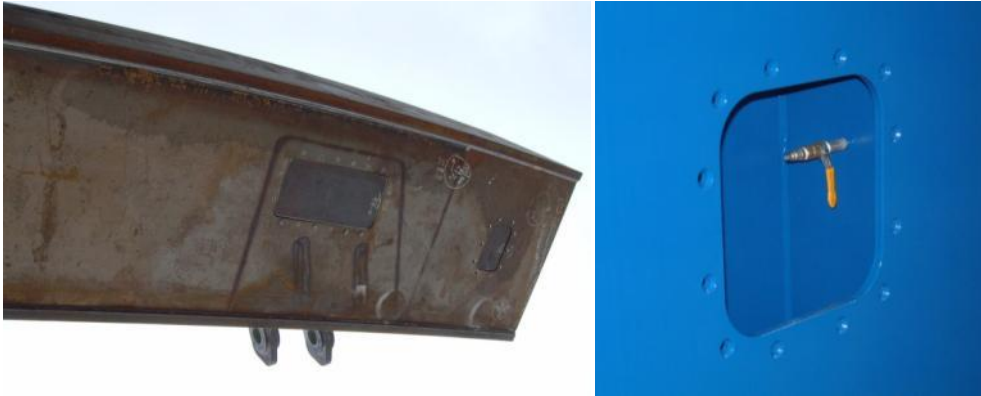
Figure C.7 Access Opening to the Arch Rib
