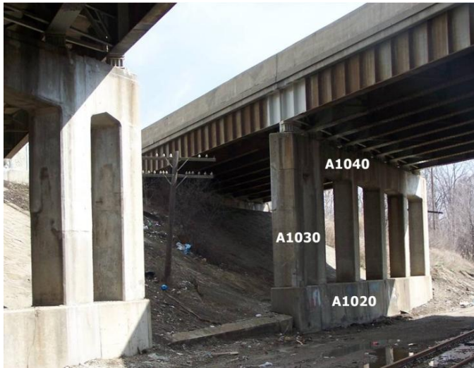
Figure B.8 Individual Elements: A1020 Walls, A1030 Columns, A1040 Cap Beams
