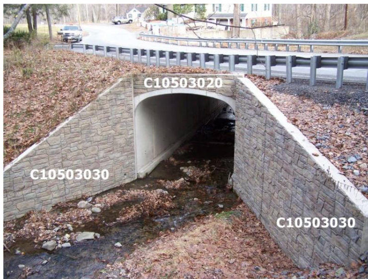
Figure B.39 Individual Elements: C1050 Drainage Systems (Sub-Elements C105030 Buried Drains (C10503020 Head Walls, C10503030 End Walls))
