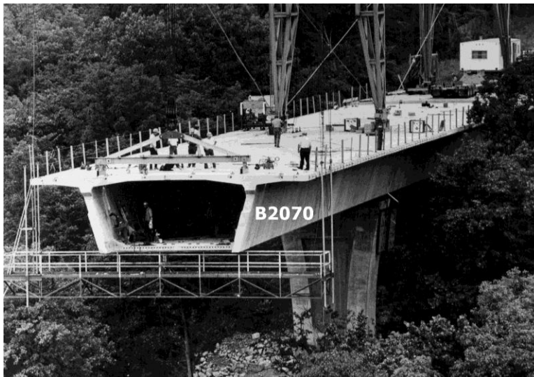
Figure B.31 Individual Elements: B2070 Segmental Box Girders
