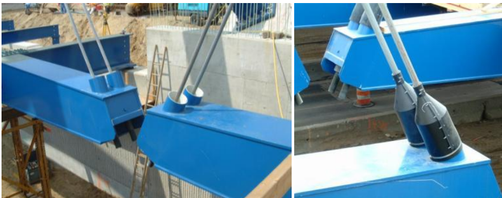
Figure C.8 Hanger Assembly and Neoprene Transition Boots
