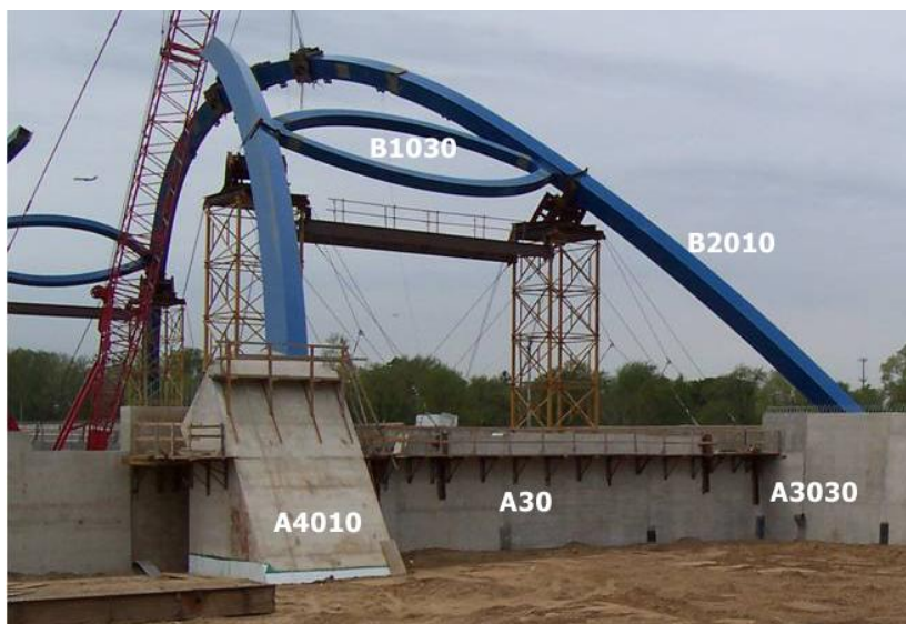
Figure B.17 Group Elements: A40 Other Supports (Individual Elements: A4010 Thrust Blocks)
