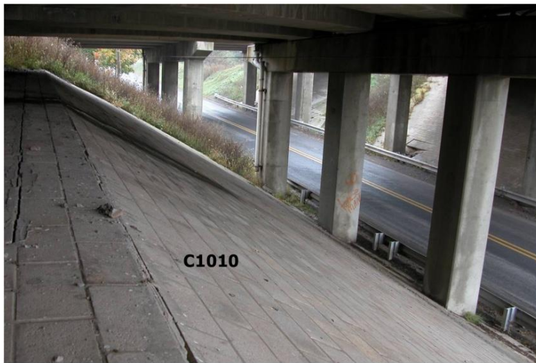
Figure B.34 Group Elements: C10 Structure Protection (Individual Elements:C1010 Slope Walls)
