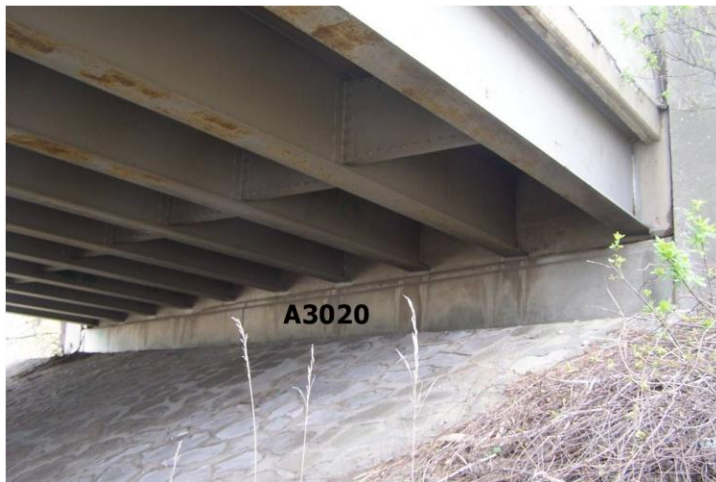
Figure B.15 Individual Elements: A3020 Stems
