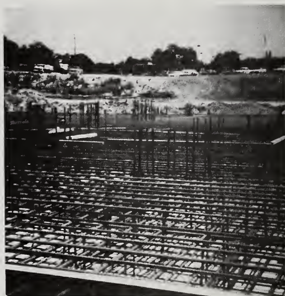
CHECKING THE SPACING AND NUMBER OF BARS COULD BE A PROBLEM
