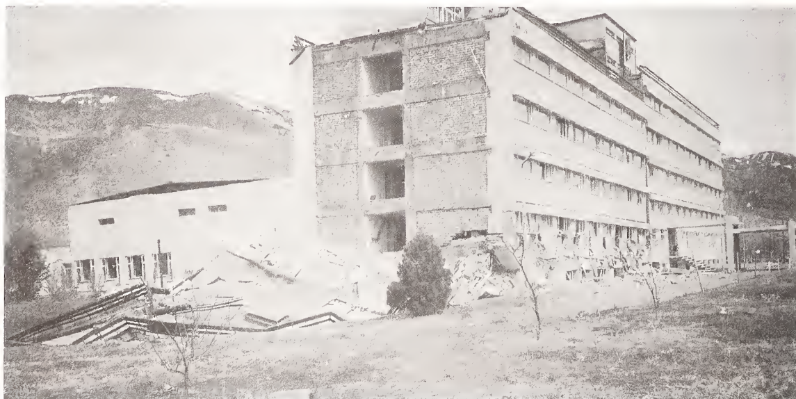
Figure 8. The Military Hospital—lost one wing, lost a story of one of the two middle wings and sustained heavy damage to the remaining two wings.
