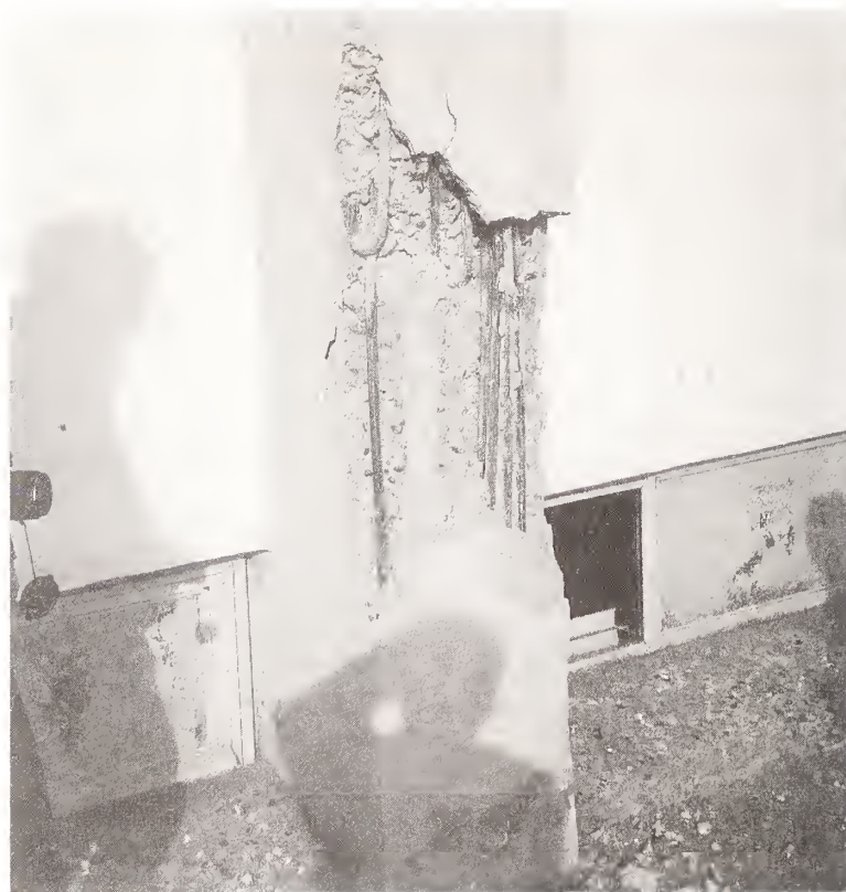
Figure 7. An external column of Unsan flour mill exhibiting short column and deficient detailing lack of shear reinforcement.
