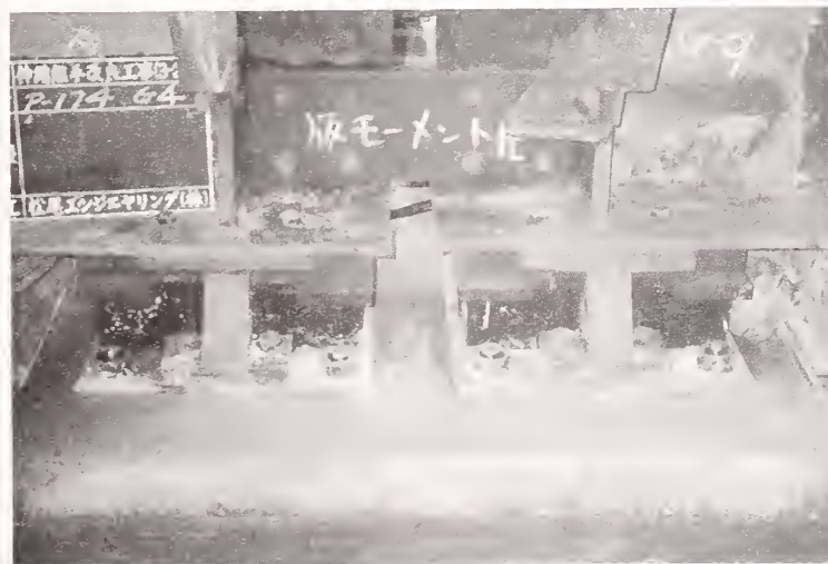
Photo 4 Deck Connection of Existing Bridge
