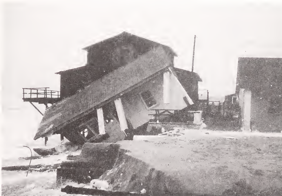
Figure 2. Example of severe storm-induced erosion and structural damage
