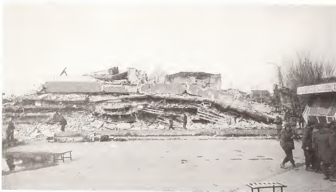
Figure 3. Typically pancaked building in Erzincan.
