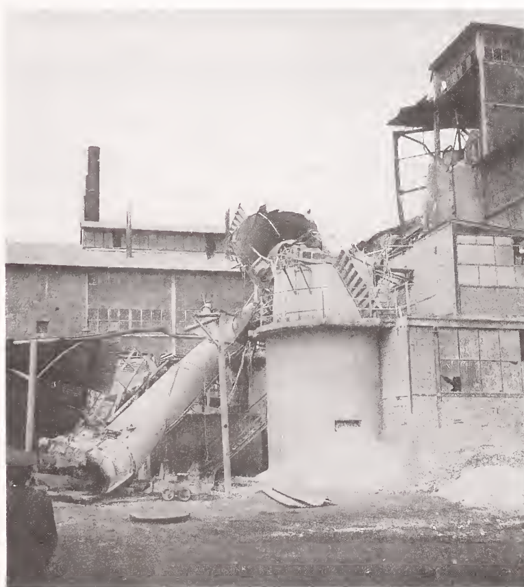
Figure 10. Collapsed stack of the calcination unit of the sugar refinery.
