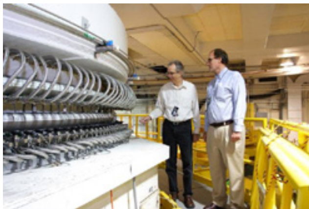
FIGURE 2: Tony Norbedo and Paul Brand inspecting headers of the thermal shield cooling system
