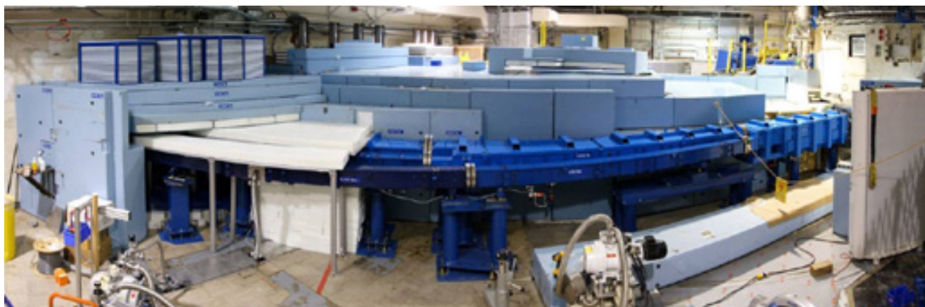
FIGURE 6: A view of the new guides and shields in the latter stages of installation in the confinement building, coming from the reactor on the right and entering D-wing on the left (The apparent curvature is an artifact arising from the fisheye-lens camera)
