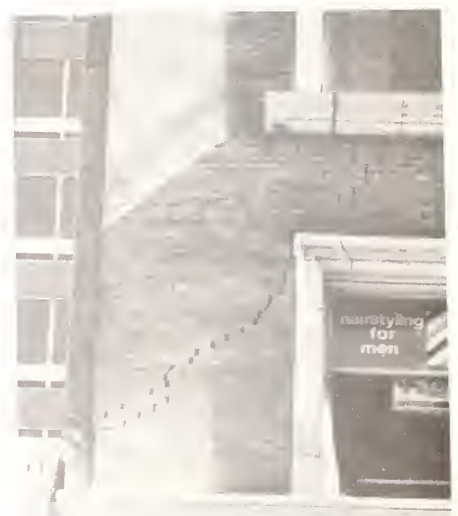
Fig. 28 Pounding Damage
