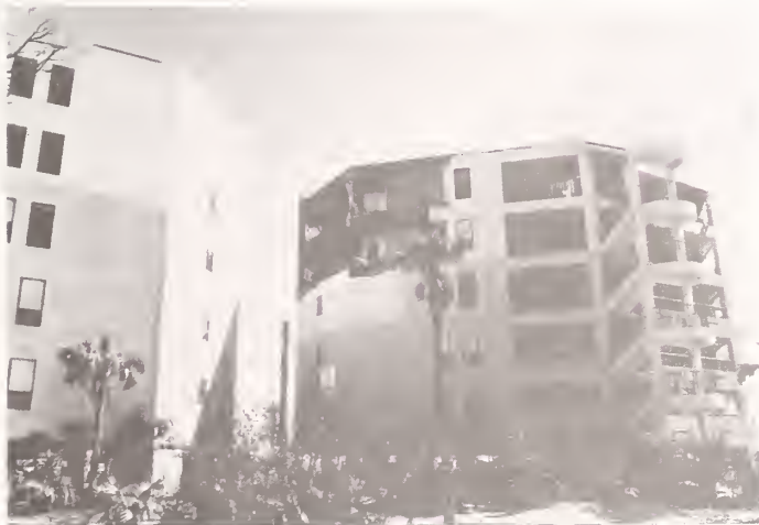
Figure 7. Cladding Failure, Isle of Palms
