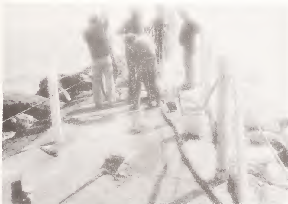
Figure 6. Sealing of the south jetty at Port Everglades, Florida.
