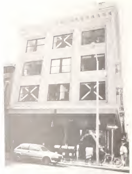
Fig. 26 Retrofit URM Building with Steel Braces
