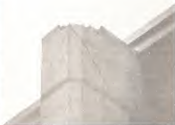
Fig. 10 Damaged Knee Joint in New Freeway
