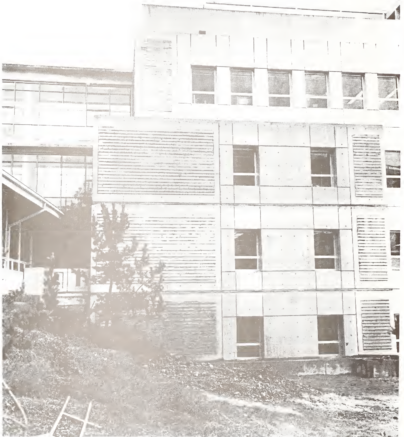
Figure 8. Longitudinal Buttress Uphill End of Building 50B
