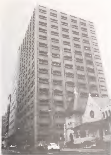
Fig. 21 Lightweight Concrete Shear Walls Failed At Base of Building
