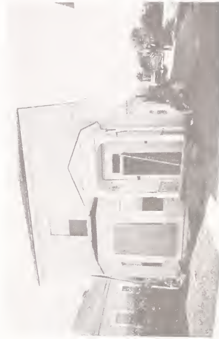
Fig. 13 Damage to House Not Bolted to Foundation
