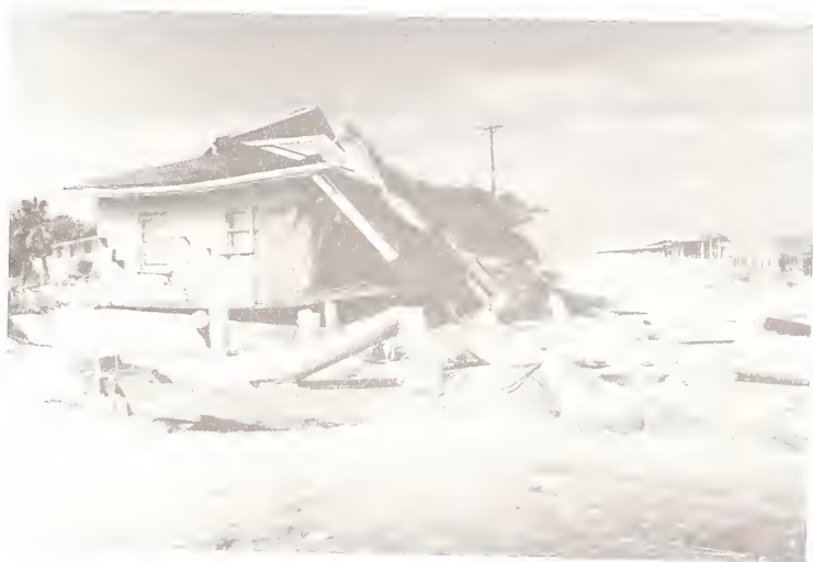
Figure 9. Concrete Pier Failure by Wave Action Near Myrtle Beach
