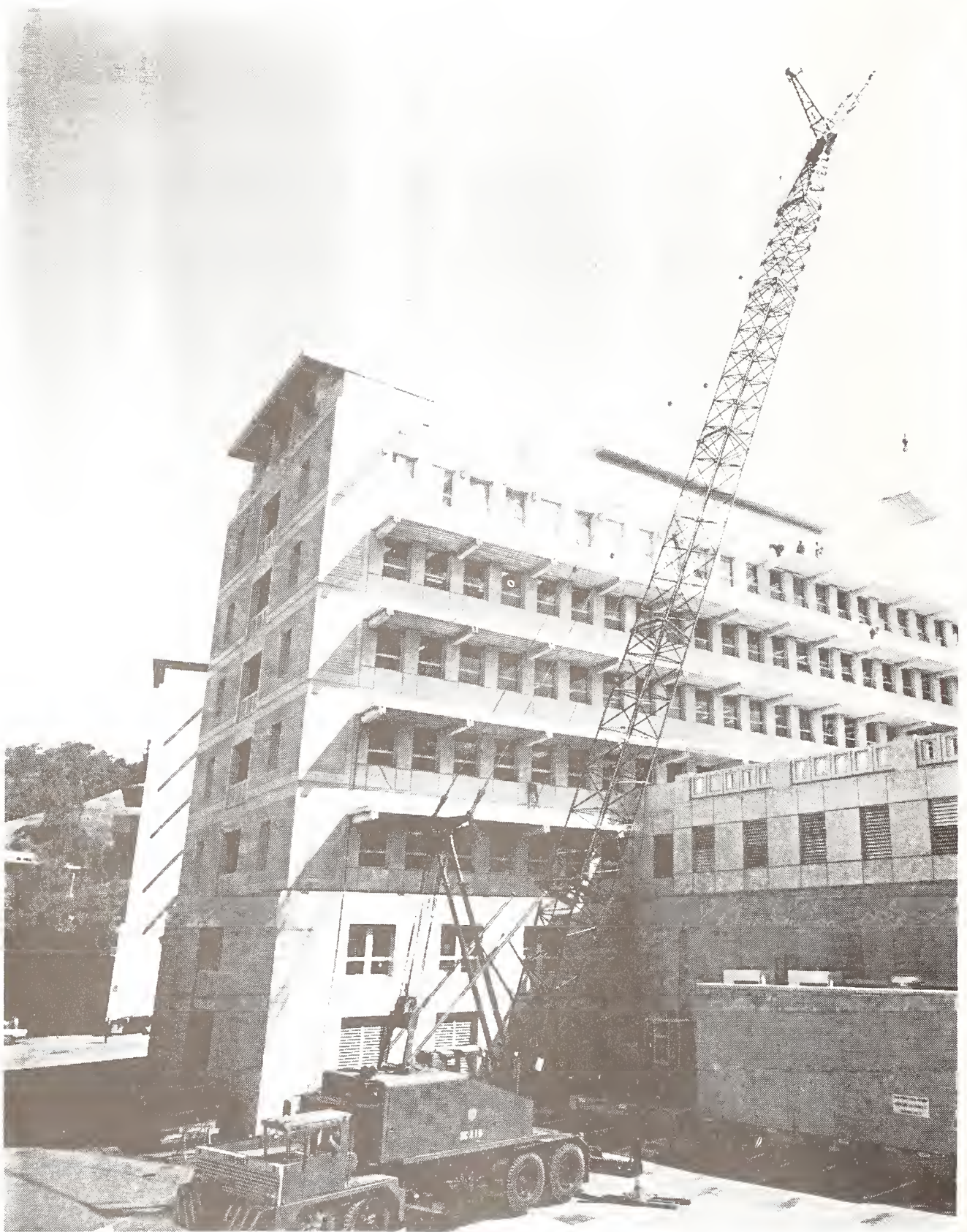
Figure 6. Removal of Concrete Sunshades from Building 50B (About 1972)
