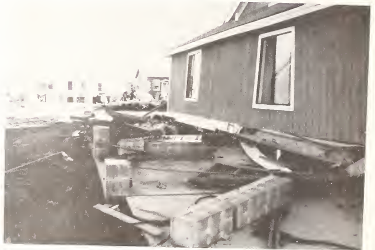
Figure 3. Masonry Pier Failure by Wind Action, Isle of Palms
