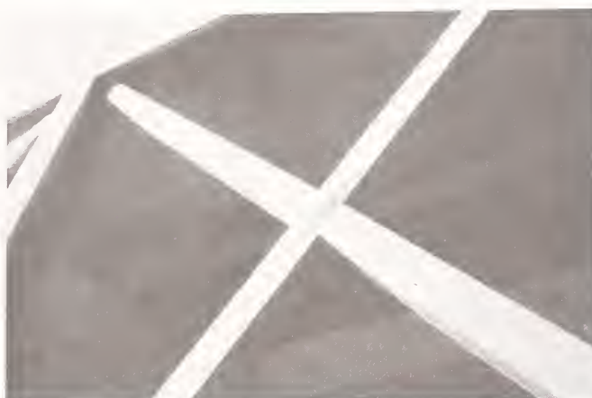
Fig. 23 Buckled Brace Intersection
