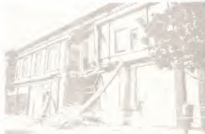
Fig. 20 In-Plane Failure of Masonry Wall
