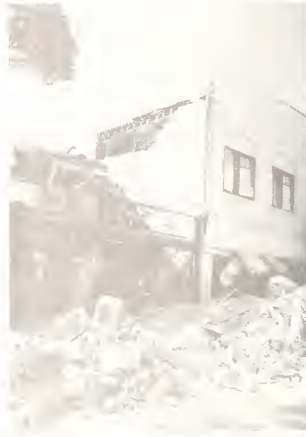
Fig. 19 Collapse of Masonry Wall Onto Adjacent Roof
