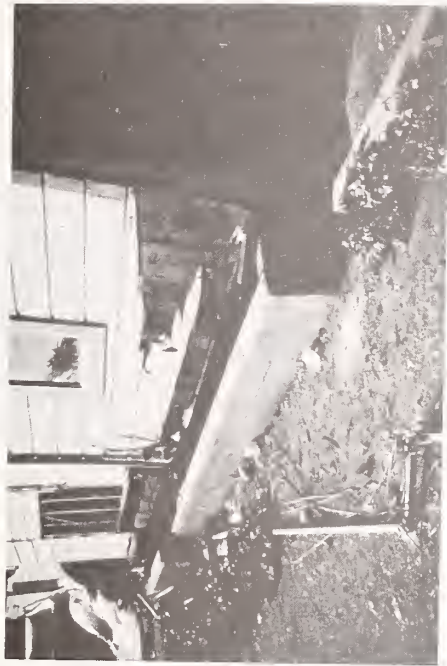
Fig. 13 Damage to House Not Bolted to Foundation
