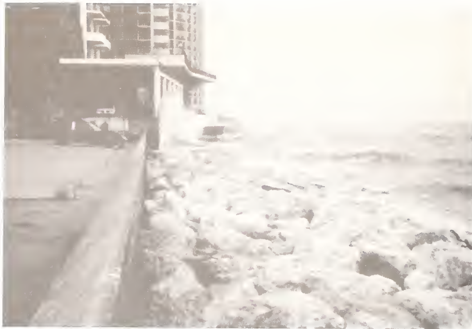
Figure 3. Low berm revetment installed at Temple Emanuel to decrease wave runup and overtopping.
