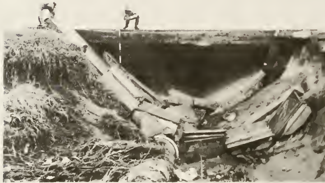
Fig. 3 Damage behind the stair-type revetment in Kotohama Coast
