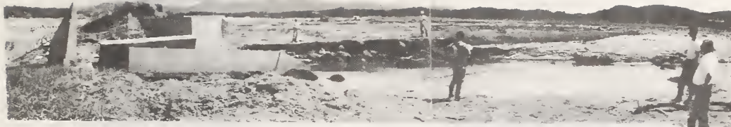
Fig. 14 Scouring behind the dike of the Tako River
