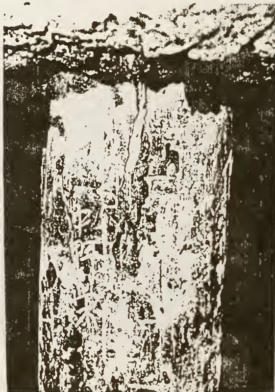
Photo 18 Hair Cracks due to Cutting Work of Pile Head (PHC Pile)
