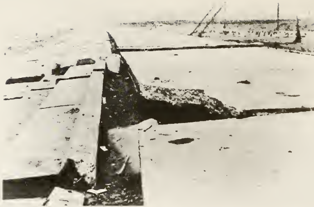
Fig. 2 Damaged stair-type revetment of Ochiai Coast in Noshiro Port
