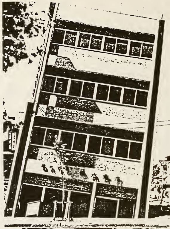
Photo 1 Overturning of Building due to Liquefaction (Niigata earthquake 1964)
