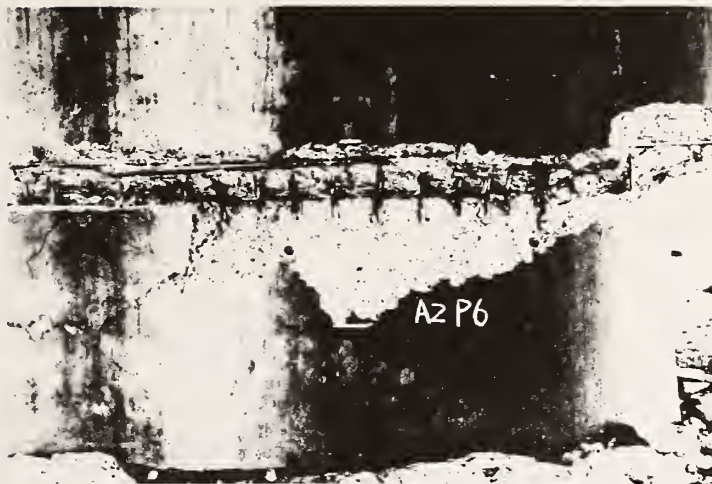
Photo 1 Damage of Pier 6 in the Sendai Bridge by Miyagi-ken-oki Earthquake of 1978
