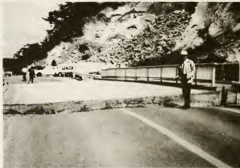
Photo. 1 Example of settlement of approaching embankment to bridge (settlement = 50 cm, height of embankment = 10 m)
