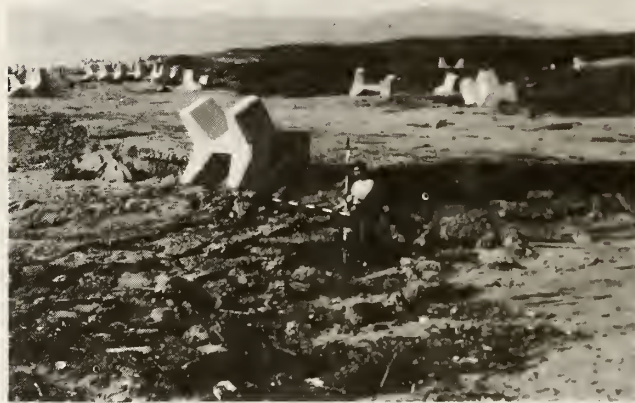
Fig. 6 Scattering of concrete blocks of wave dissipation breakwater in Minehama Coast (1)
