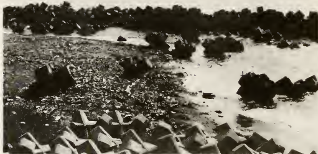
Fig. 5 Scattering of concrete blocks of detached breakwater in Hachimori Coast
