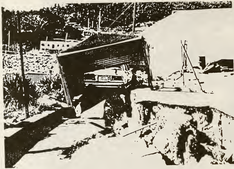
Photo 5 Collapse of Fill Ground (Izu-Ohshima kinkai earthquake 1978)
