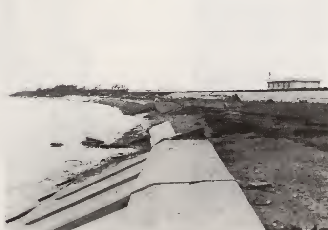
Fig. 16 Damaged revetment of the Yoneshiro River
