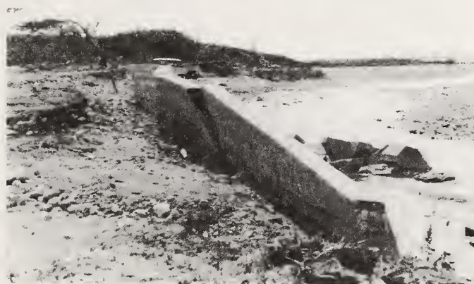
Fig. 9 Damaged revetment of the Mizusawa River (looking down-stream)
