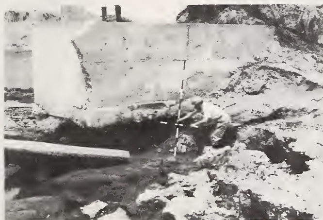
Fig. 15 Scouring under the abutment
