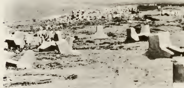
Fig. 7 Scattering of concrete blocks of wave dissipation breakwater in Minehama Coast (2)
