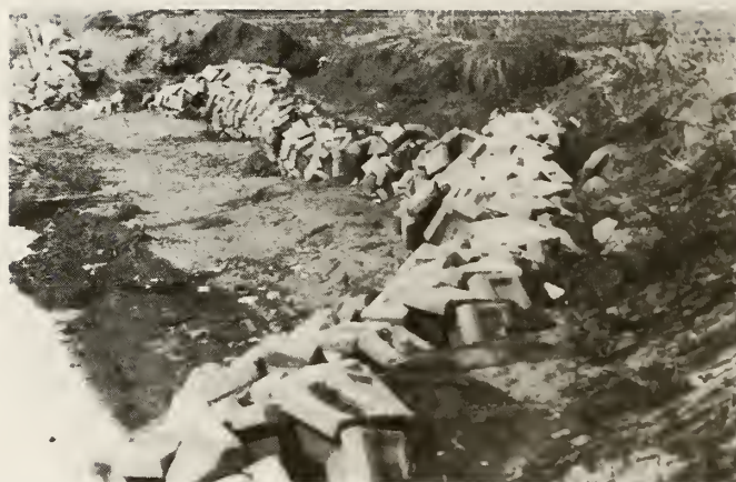
Fig. 11 Damaged blocks and eroded embankment of the river
