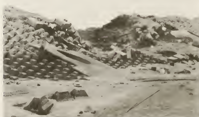
Fig. 13 Situation of the damaged embankment in the Tako River
