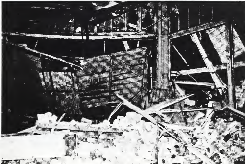
Photo 6 Masonry parapet of a three-story unreinforced masonry building fell, causing the collapse of an adjacent building, Pasadena.
