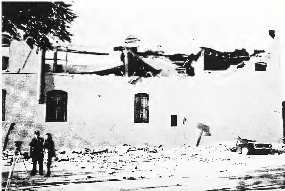
Photo 2 Collapsed unreinforced brick parapet and wall of a building in Uptown, Whittier. Falling bricks crushed cars parked adjacent to the building.
