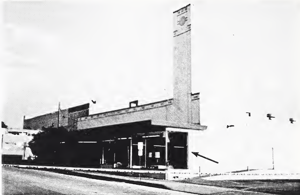
Photo 35 This remodeled masonry building experienced considerable damage to windows. Because large pieces of broken glass were strewn on the sidewalk, the building was cordoned off.
