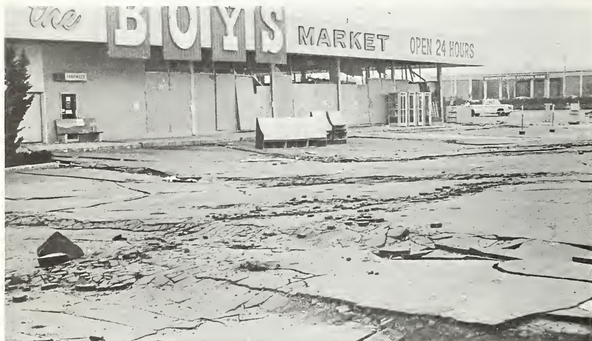
Figure 7.40 Considerable ground movement is evident in the parking lot of the shopping center at the corner of Hubbard Avenue and Glenoaks Boulevard.
