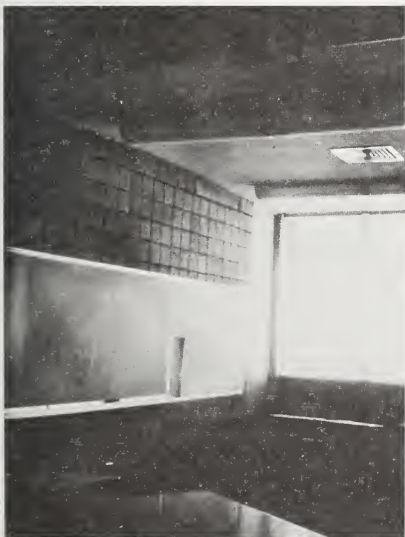
Figure 6.45 Displacement of concrete block at top of transverse partition, Los Angeles County Juvenile Facility.
