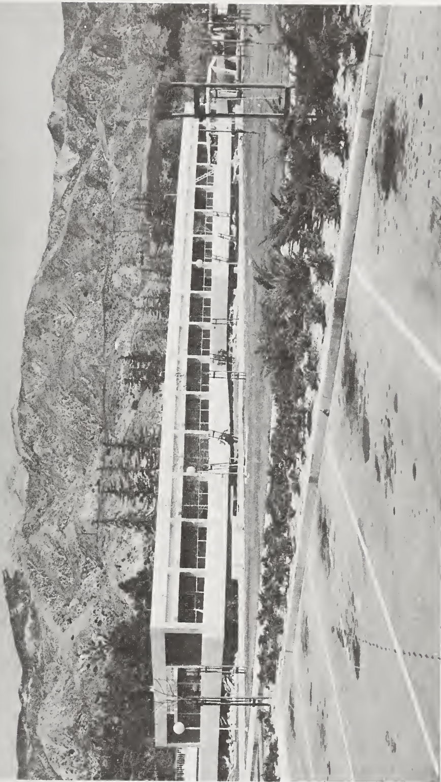
Figure 5.10 South and west elevations of the Psychiatric Unit. The ground story of this building was totally collapsed. What appears to be the ground floor was the first floor of this building.
