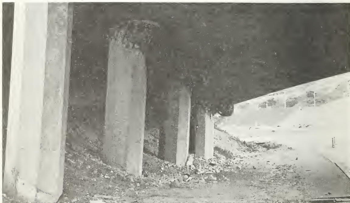
Figure 7.23 Spiral column failures in bent 2 at the west end of the Northwest Connector Overcrossing.
