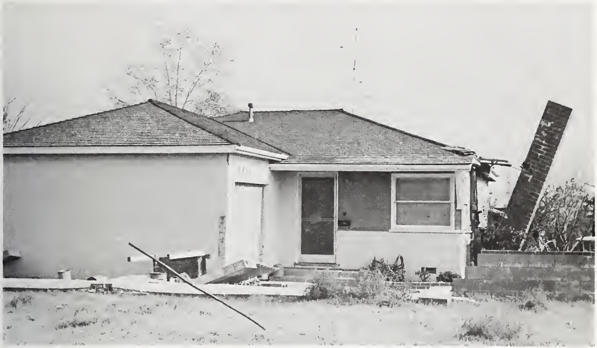
Figure 5.164 Leaning reinforced brick masonry chimney.
