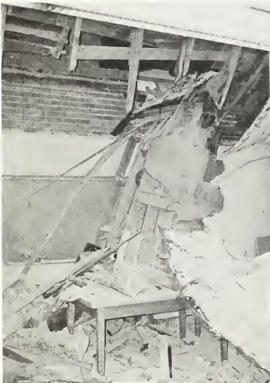
Figure 6.3 A portion of the parapet wall fell through the roof and came to rest on a table, Los Angeles High School.
