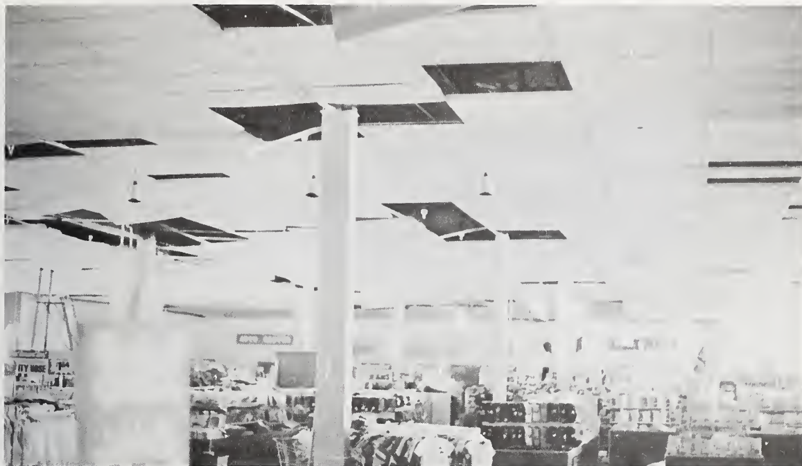
Figure 5.130 Interior view of Grants Department Store showing missing portions of suspended ceiling. Most of the merchandise which had been thrown to the floor had been picked up when this photograph was taken.
