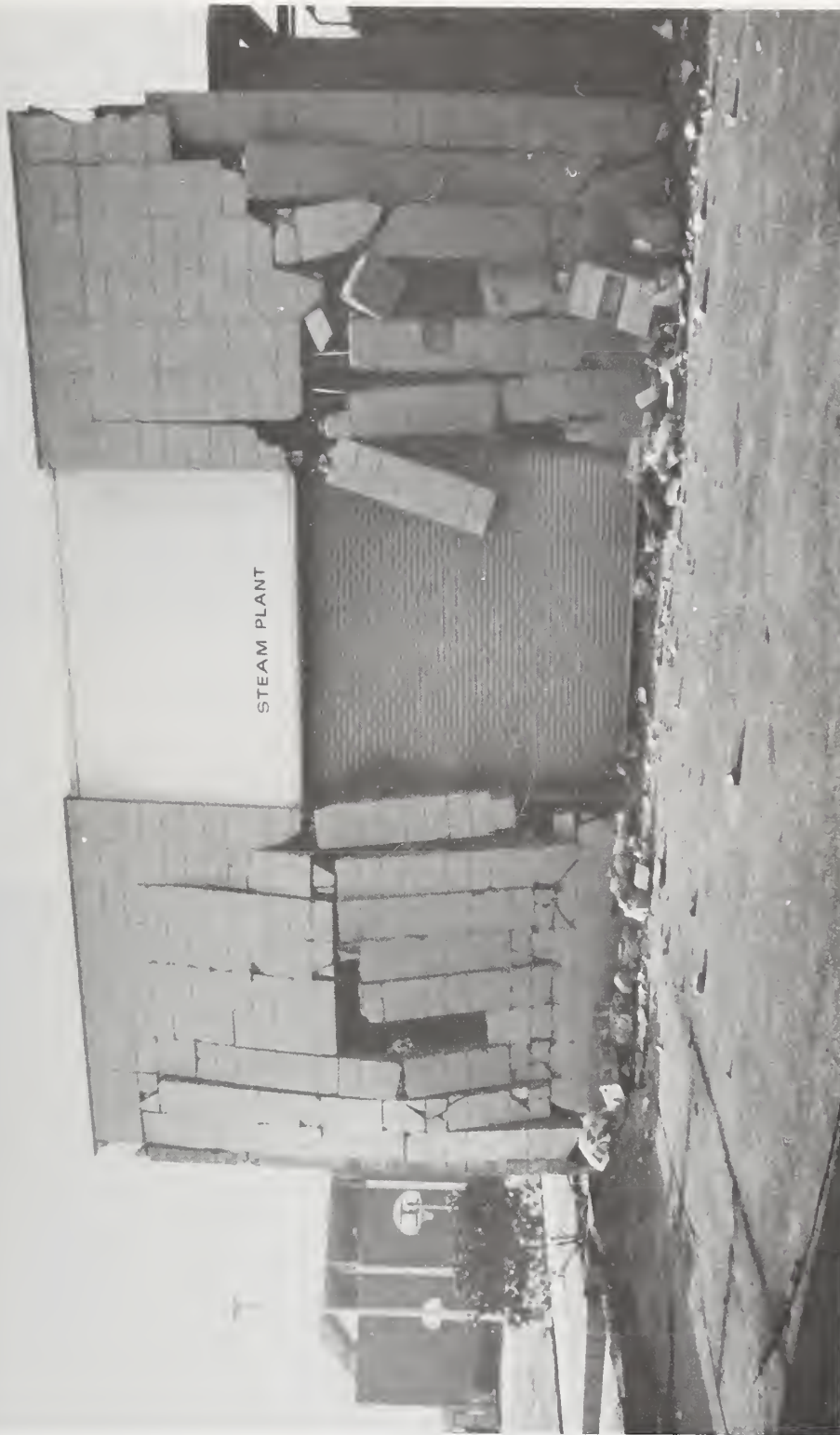
Figure 6.52 Damage to concrete block wall, Los Angeles County Juvenile Facility. Note absence of horizontal reinforcement. Only reinforced vertical cells are filled with grout.
