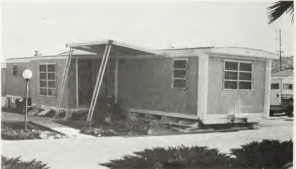
Figure 5.173 Mobile home (Soledad Canyon Road, Newhall) which was damaged when it fell off its small concrete and metal base supports.
