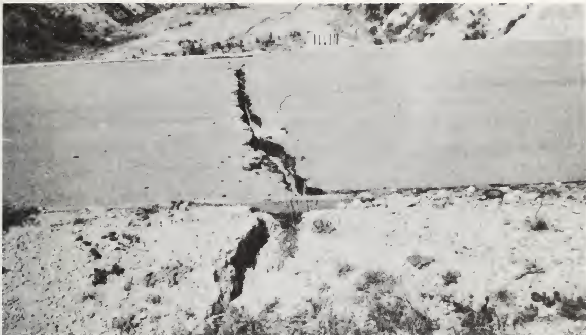
Figure 8.30 Looking northwesterly toward basin showing crack in the pavement and a 2-inch vertical displacement of paved crest of dam (Stetson Debris Basin).
