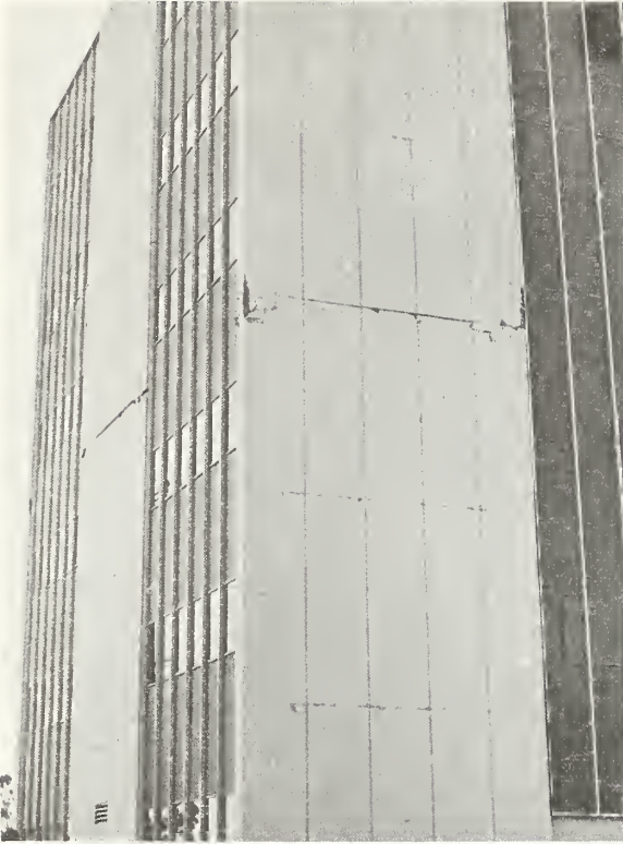
Figure 5.101 South elevation of the Indian Hills Medical Center. Note the horizontal crack and spalling visible on the left shear wall at the fourth-floor level.
