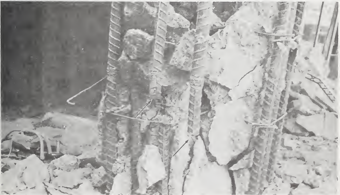
Figure 5.21 Close-up view of the first story column in the northeast corner of Wing B. Note the two fractured main reinforcing bars (arrows) and broken ties.
