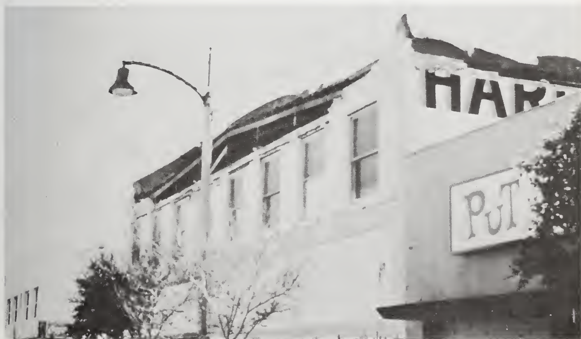
Figure 5.141 Damaged parapet and wall.
