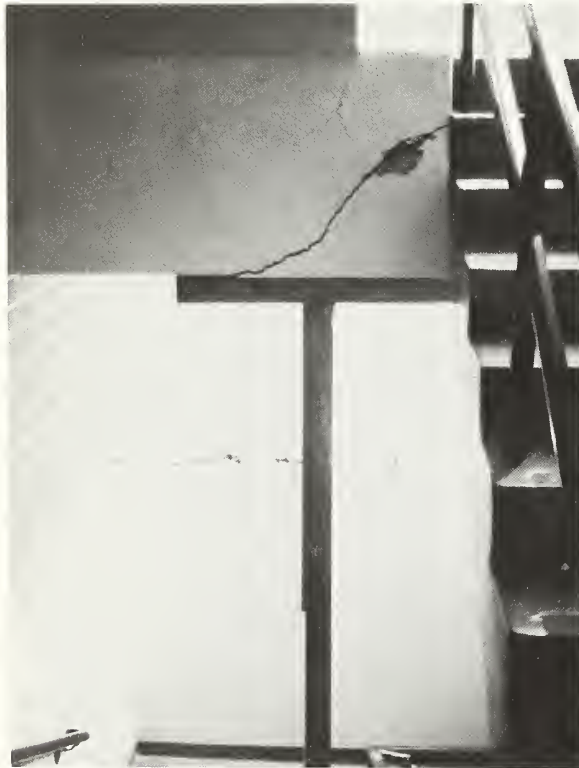
Figure 5.82 Interior view of damaged reinforced concrete shear wall at the east end of the center section of Pacoima Hospital.
