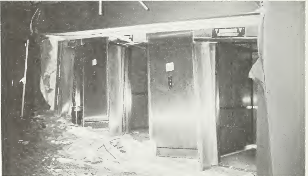
Figure 5.29 Damaged elevators in the Wing A lobby.
