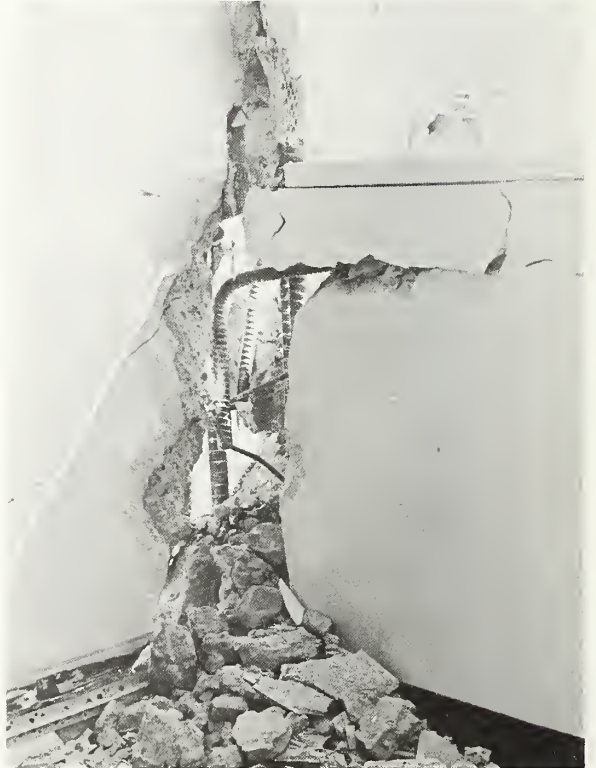
Figure 5.59 Damaged connection between the spandrel and shear wall on the southeast corner of the fourth floor.
