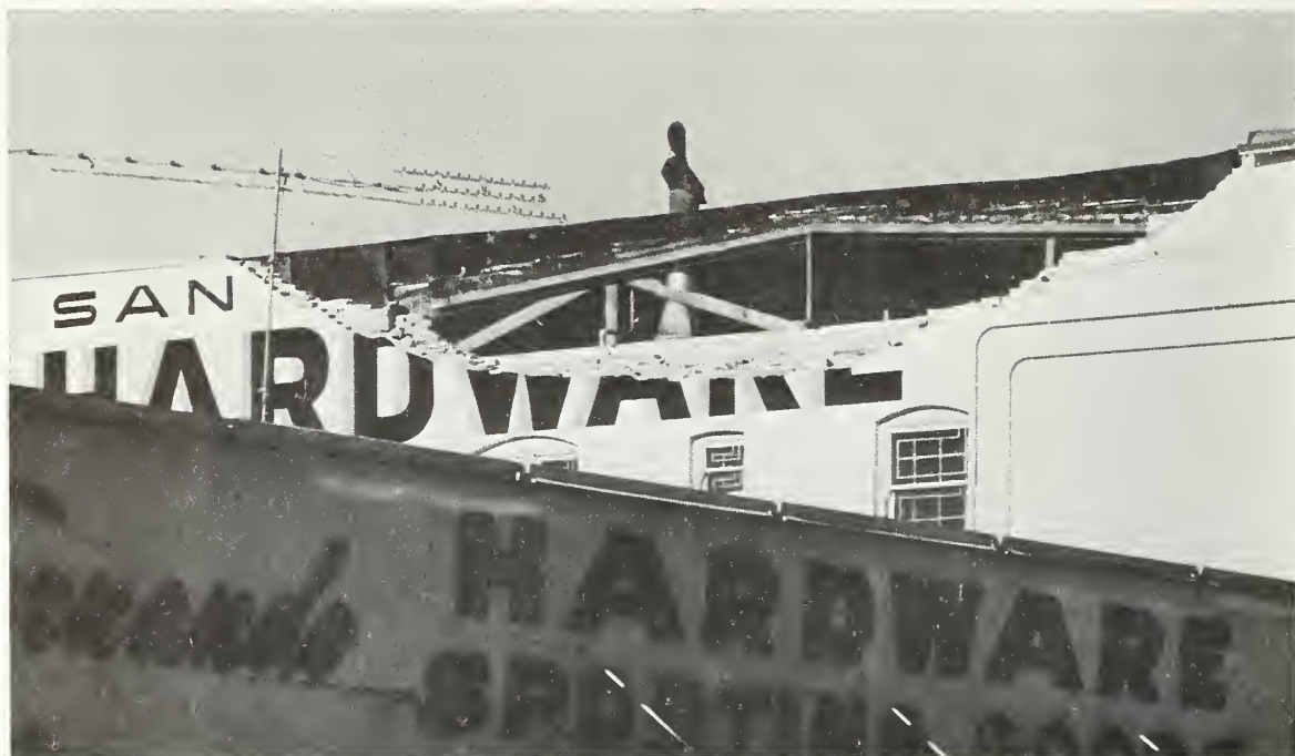
Figure 5.142 Damage to brick masonry parapet wall.
