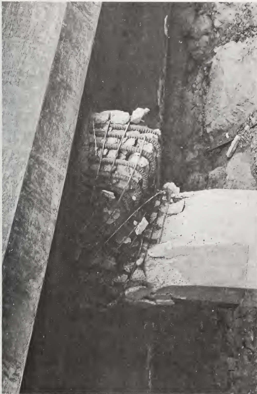
Figure 7.24 Close up of exterior spiral column.
