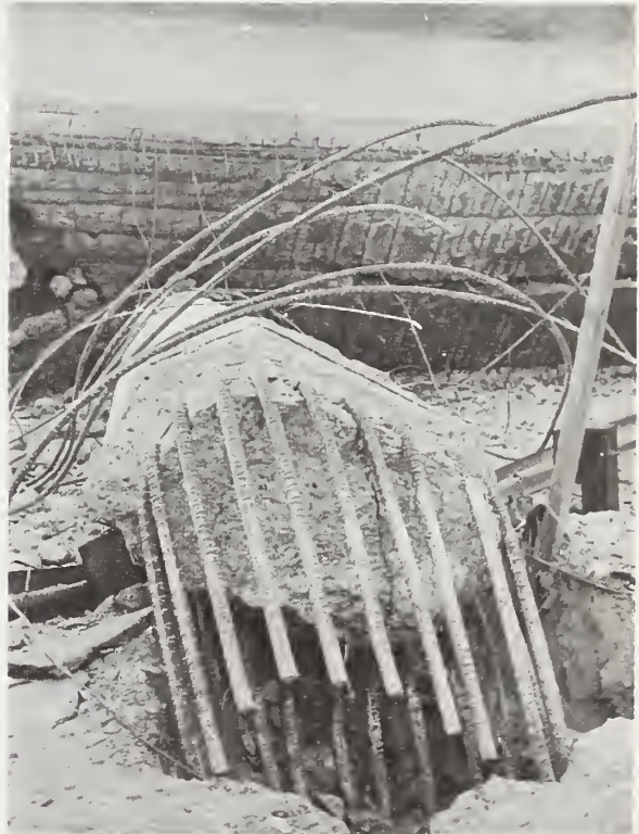
Figure 7.20 Base of the column which pulled out from the 6-ft diameter cast-in-place drilled shaft. Note the stripping of the reinforcement of the bottom of the girder in the background of the picture.
