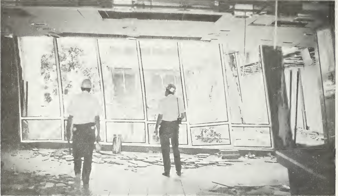
Figure 5.28 Damaged main lobby in Wing A. Note the window mullion distortion. The planted area seen through the window is a court enclosed by the four wings.
