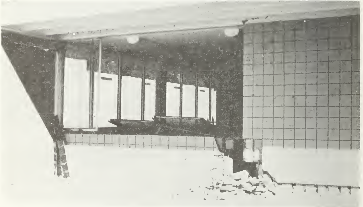
Figure 6.43 Damage to west wall of boys' school, Los Angeles County Juvenile Facility. Window fell inward.
