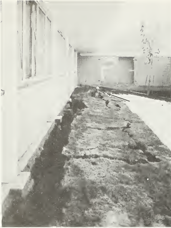
Figure 6.38 Ground crack adjacent to girls' living unit, Los Angeles County Juvenile Facility. Man standing in the crack is 6 ft 0 in tall.
