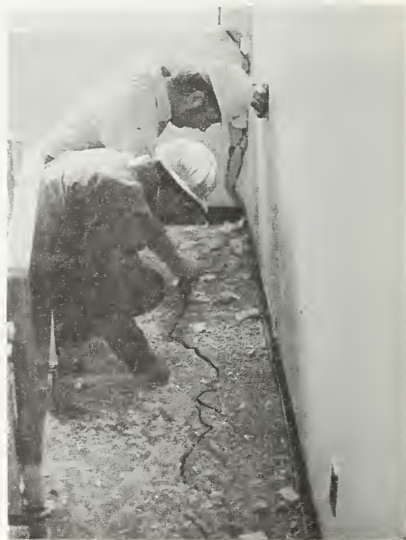
Figure 5.68 Damaged southwest corner room on the third floor. Note floor and spandrel cracking.
