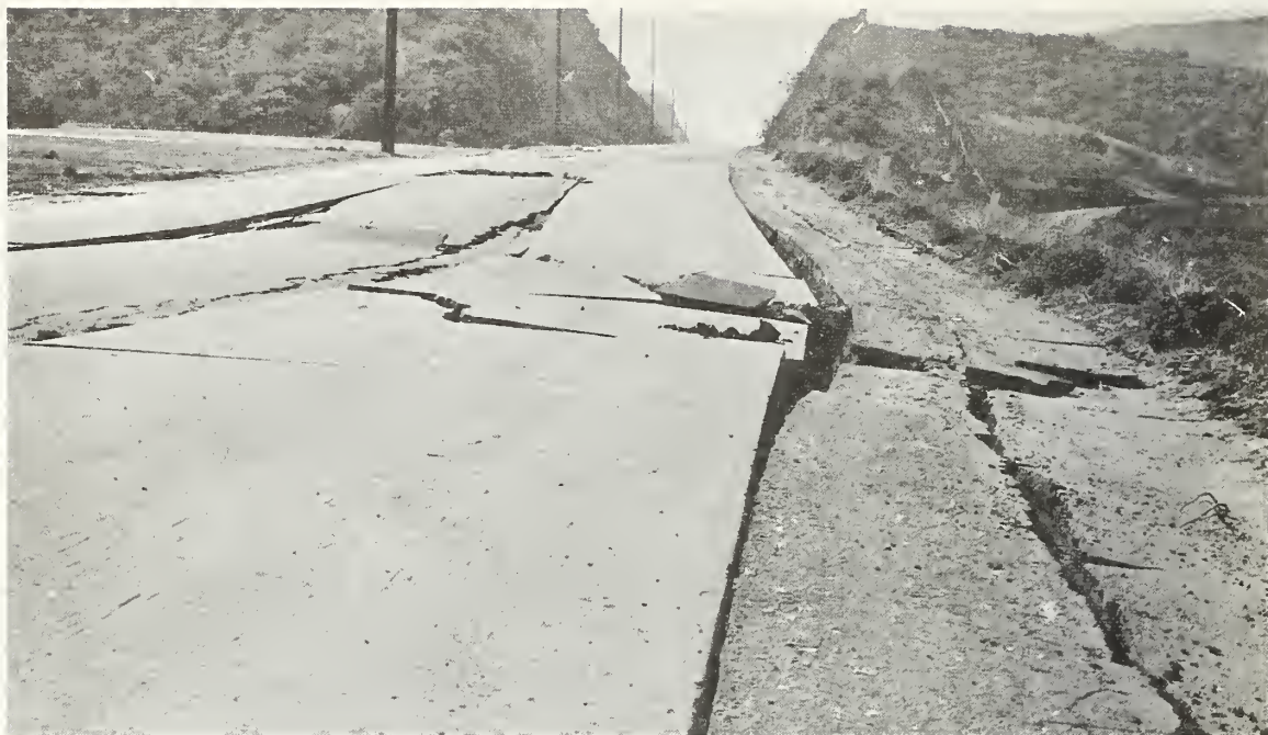
Figure 7.35 Road cave-in and ground cracks along Blucher Avenue along the eastern edge of the lower Van Norman Reservoir.
