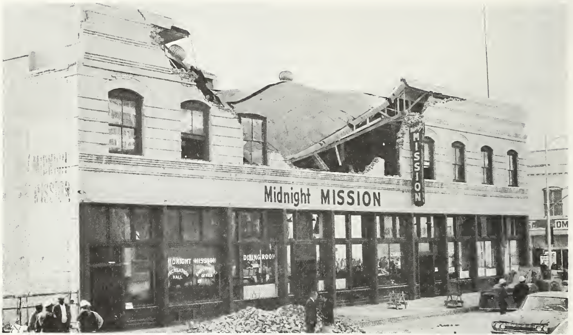
Figure 5.148 Midnight Mission, 396 South Los Angeles Street, in downtown Los Angeles. This building, erected in 1896, provided shelter for about 200 men. One man was killed when he ran out of the front door and was struck by falling masonry. (Los Angeles Times Photo).
