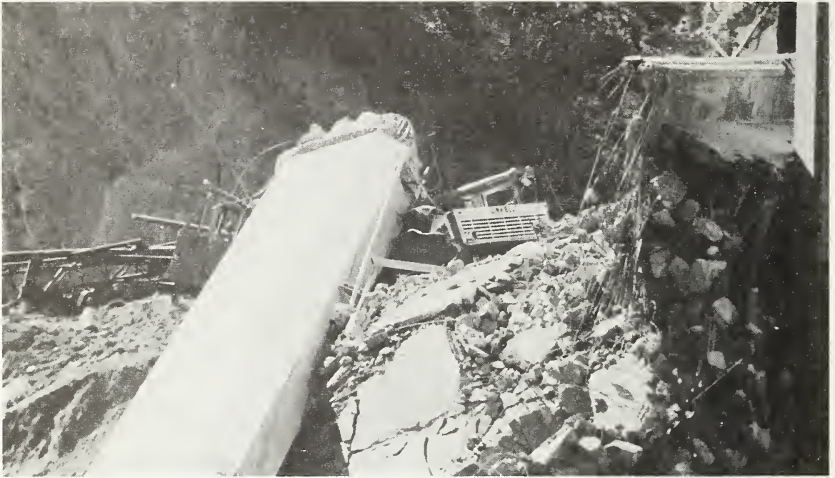
Figure 7.8 The top of Pier 5 and girder debris from the South Connector Overcrossing.
