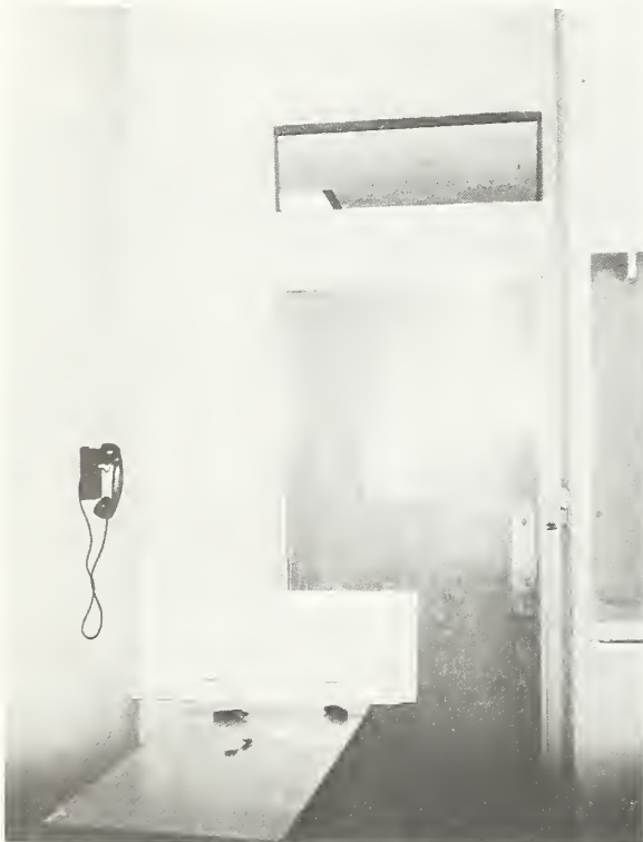
Figure 6.33 Ventilating louvers pulled loose from corridor wall above classroom doors (louver placed on table for photo), Crescenta Valley High School.
