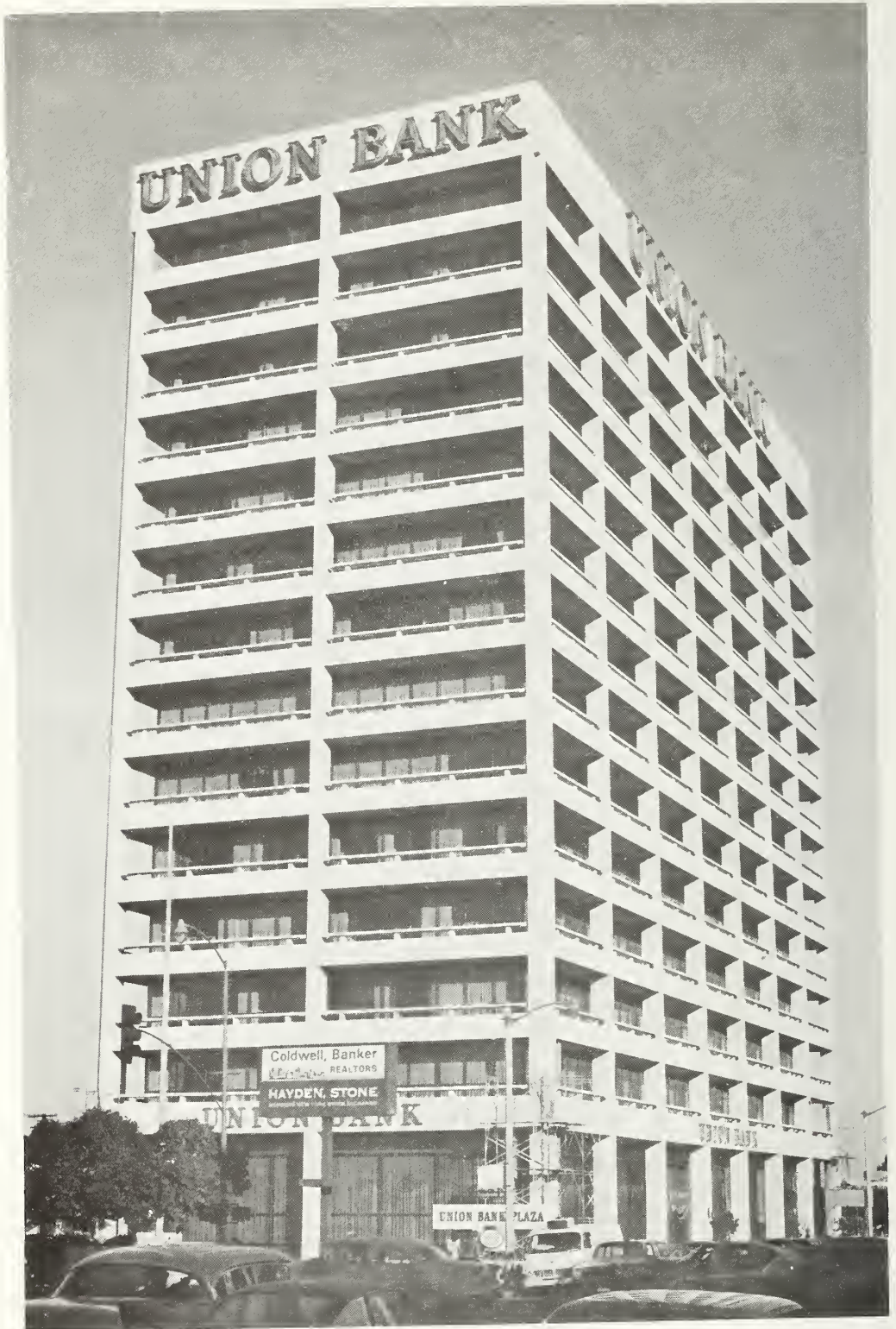
Figure 5.113 The south and west elevations of the thirteen-story Union Bank building. All four exterior corner columns in this reinforced concrete structure were cracked at the second floor level.
