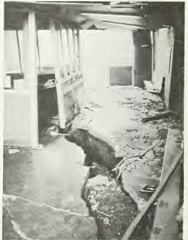
Figure 6.39 Large displacement in floor of girls' living unit, Los Angeles County Juvenile Facility. Structure did not collapse.
