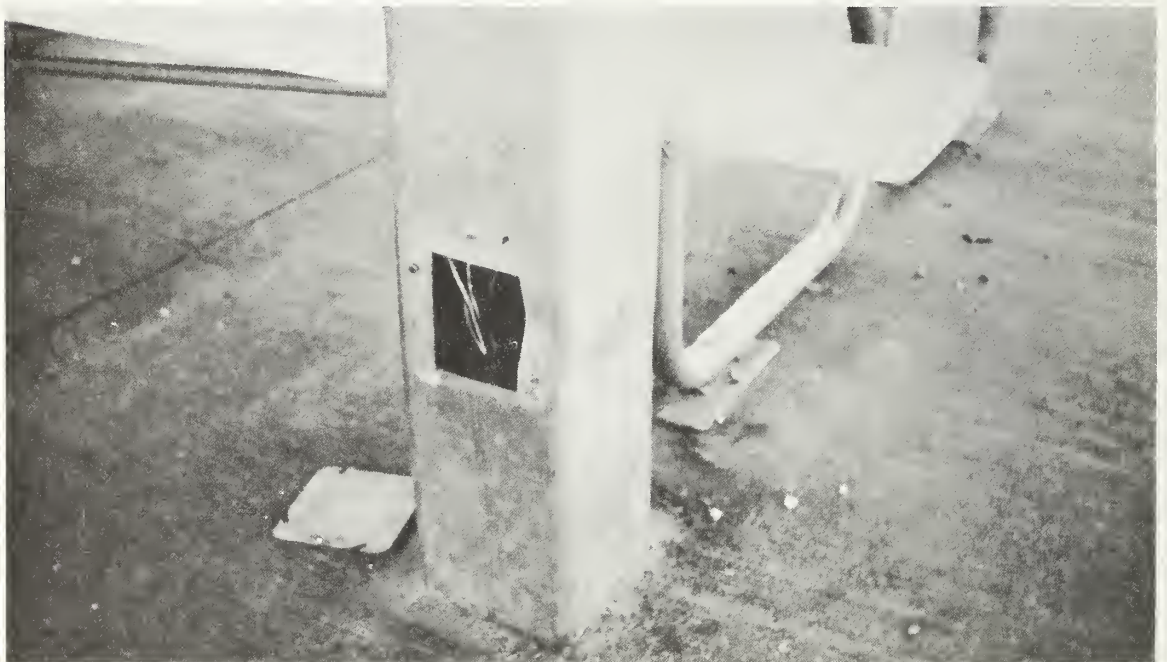
Figure 6.13 Lunch shelter columns were permanently bent at opening for electrical outlet box, Van Gogh Street School.
