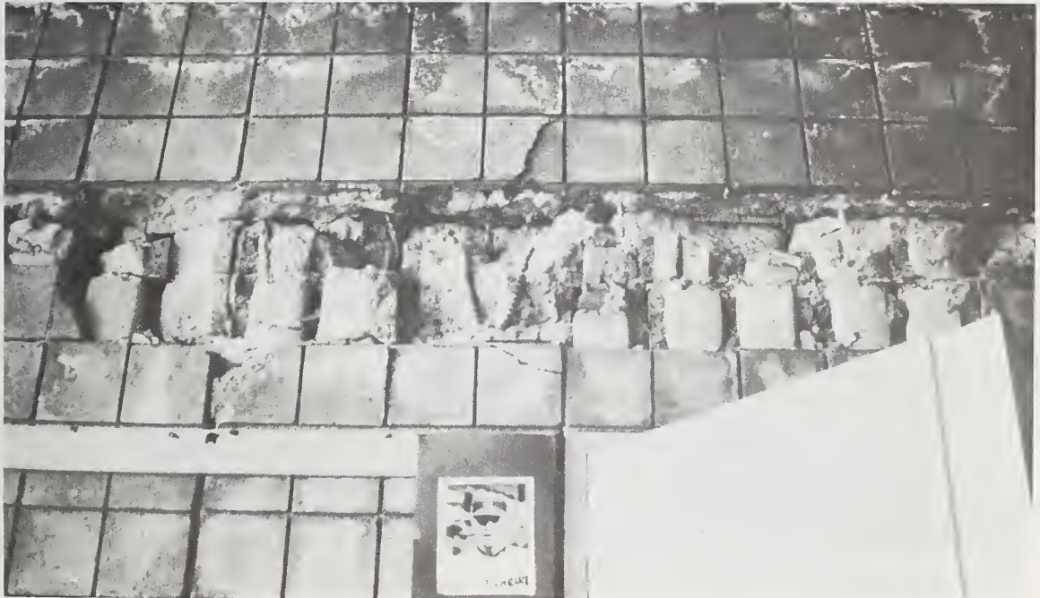
Figure 6.50 Damage to wall at change in roof elevation (interior), Los Angeles County Juvenile Facility.
