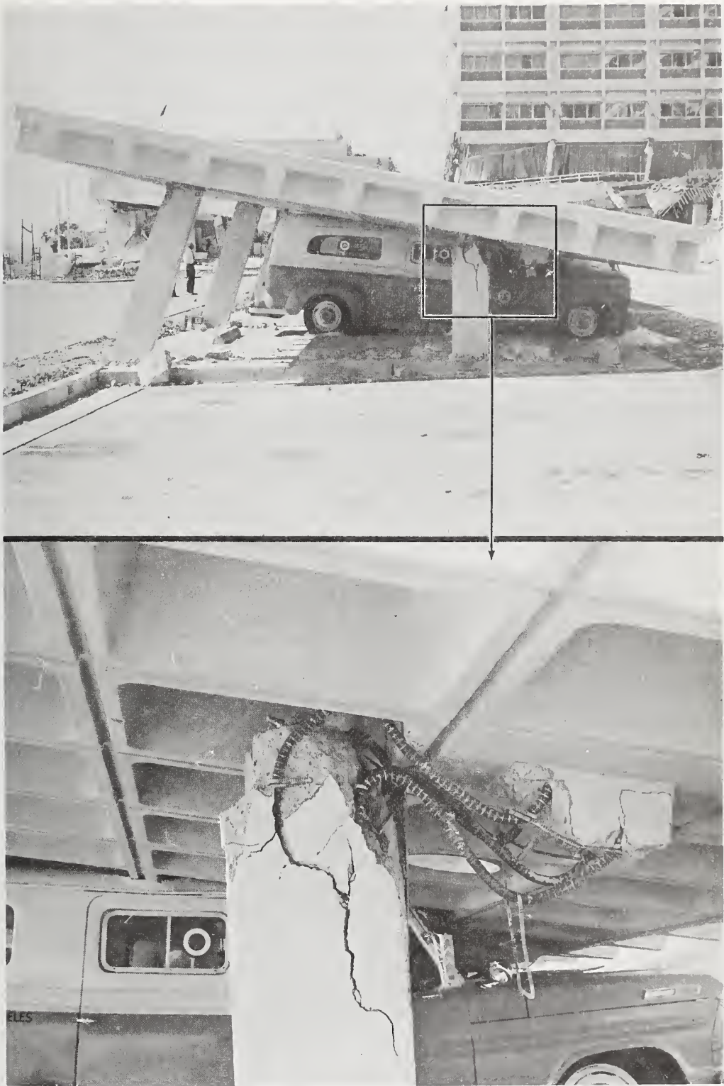
Figure 5.39 Damaged reinforced concrete ambulance port south of Wing D.
