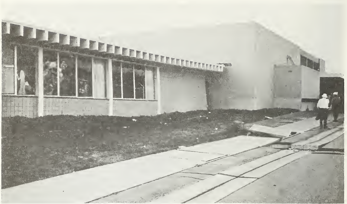
Figure 6.42 East wall of girls' school, Los Angeles County Juvenile Facility. Note distress at right (north) end adjacent to taller (cafeteria) building and ground rupture.
