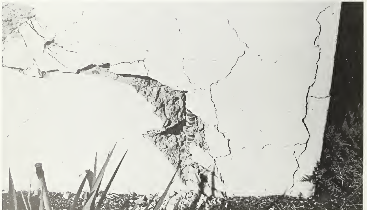
Figure 5.105 Cracking at the base of the southeast corner shear wall. Note the exposed reinforcing bar.
