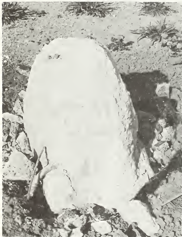
Figure 5.24 Close-up view (looking south) of one of the failed ground-story columns which originally supported the first-floor garden roof in front of Wing D. This is the same column seen in figure 5.23, the third from the right.
