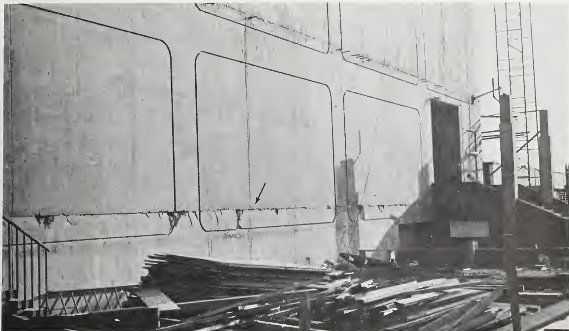
Figure 5.176 Horizontal crack along the construction joint at the base of the structure.
