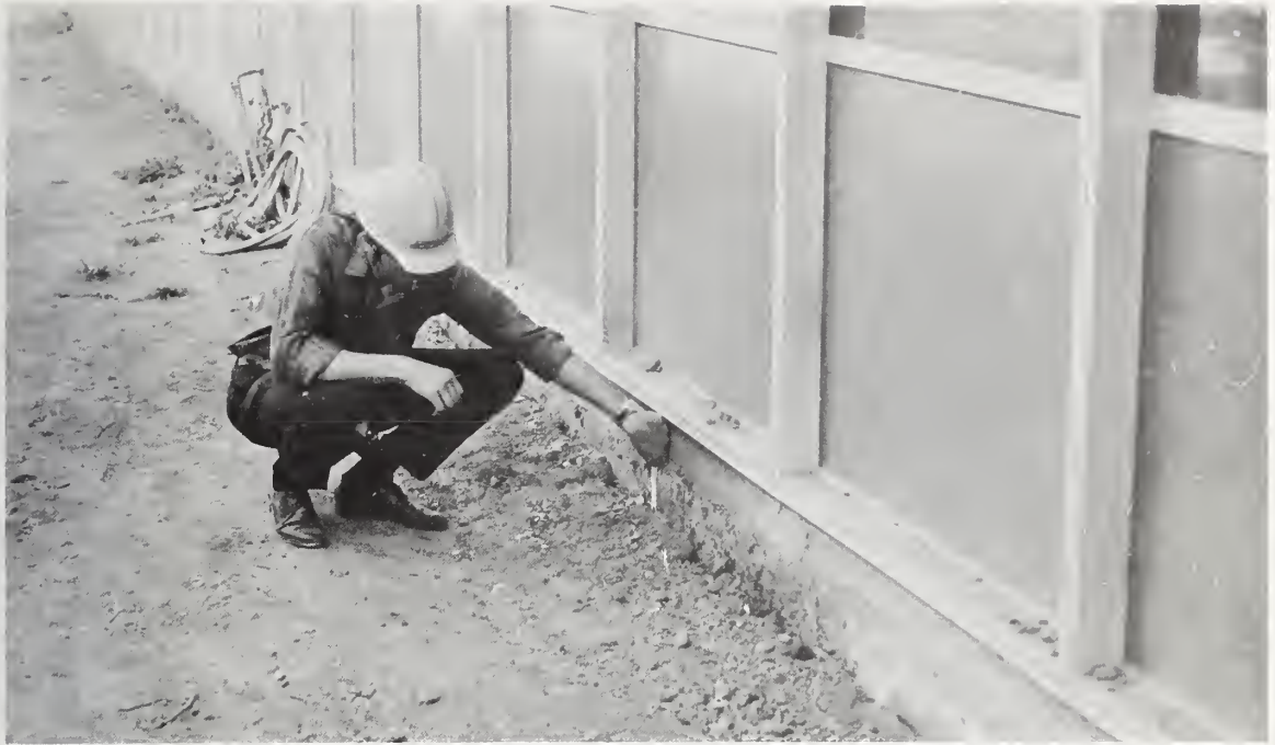
Figure 5.86 Relative movement between north section and ground.
