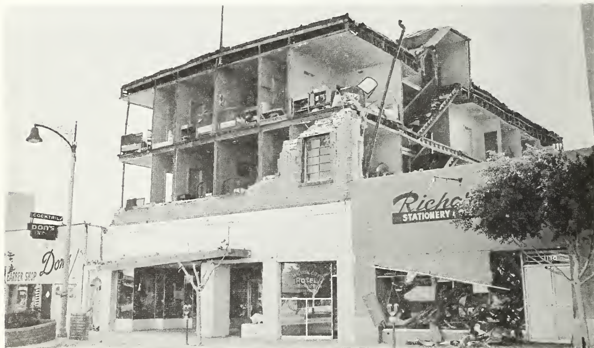
Figure 5.139 Total collapse of brick masonry wall surrounding three-story wood frame building (Mission City Hotel).
