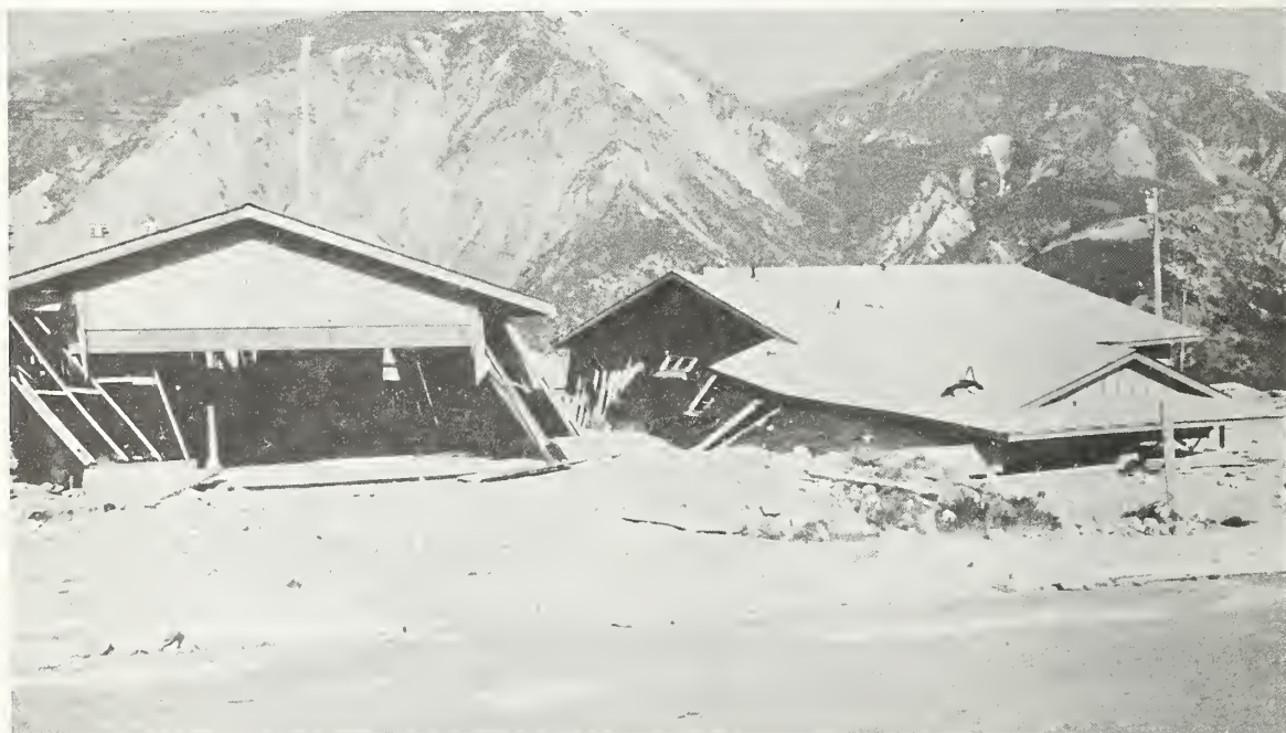
Figure 5.169 Partially collapsed houses under construction.
