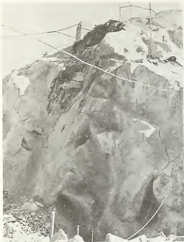
Figure 8.27 Damage to gunite left abutment, Pacoima Dam.
