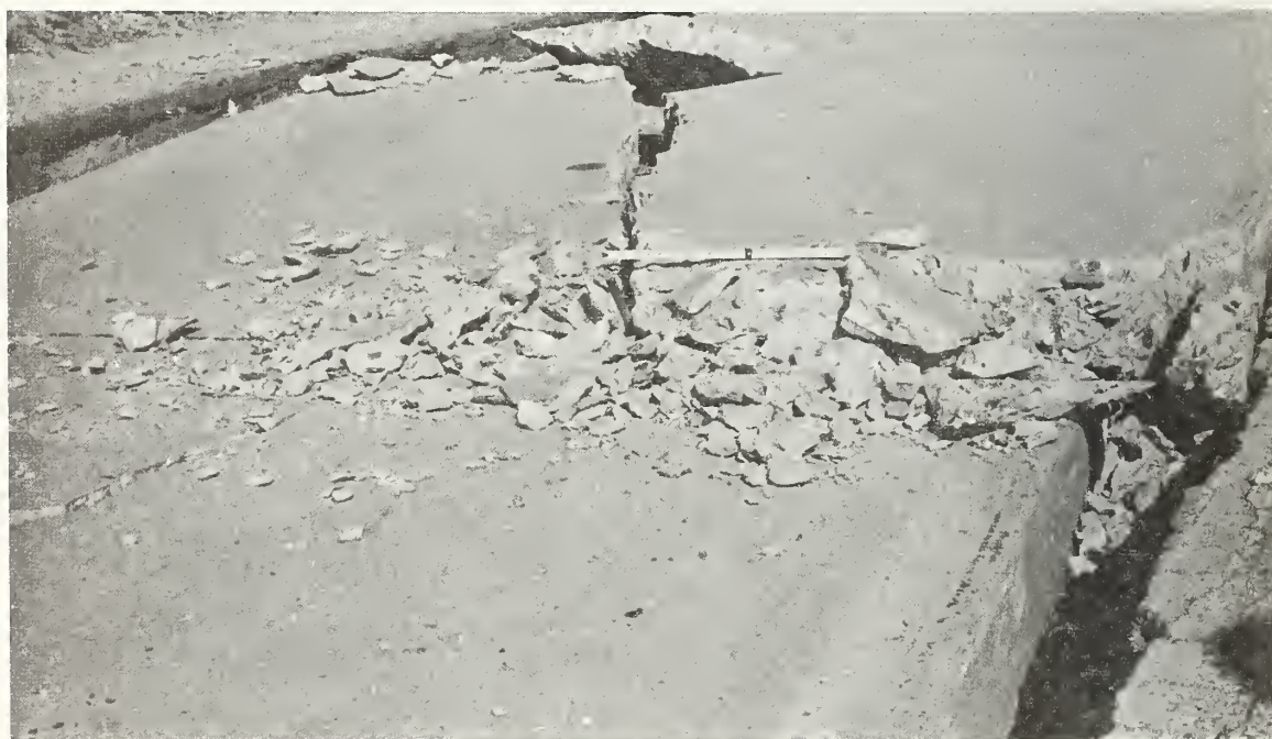
Figure 7.36 Concrete road slabs were crushed by the ground motion in this location.
