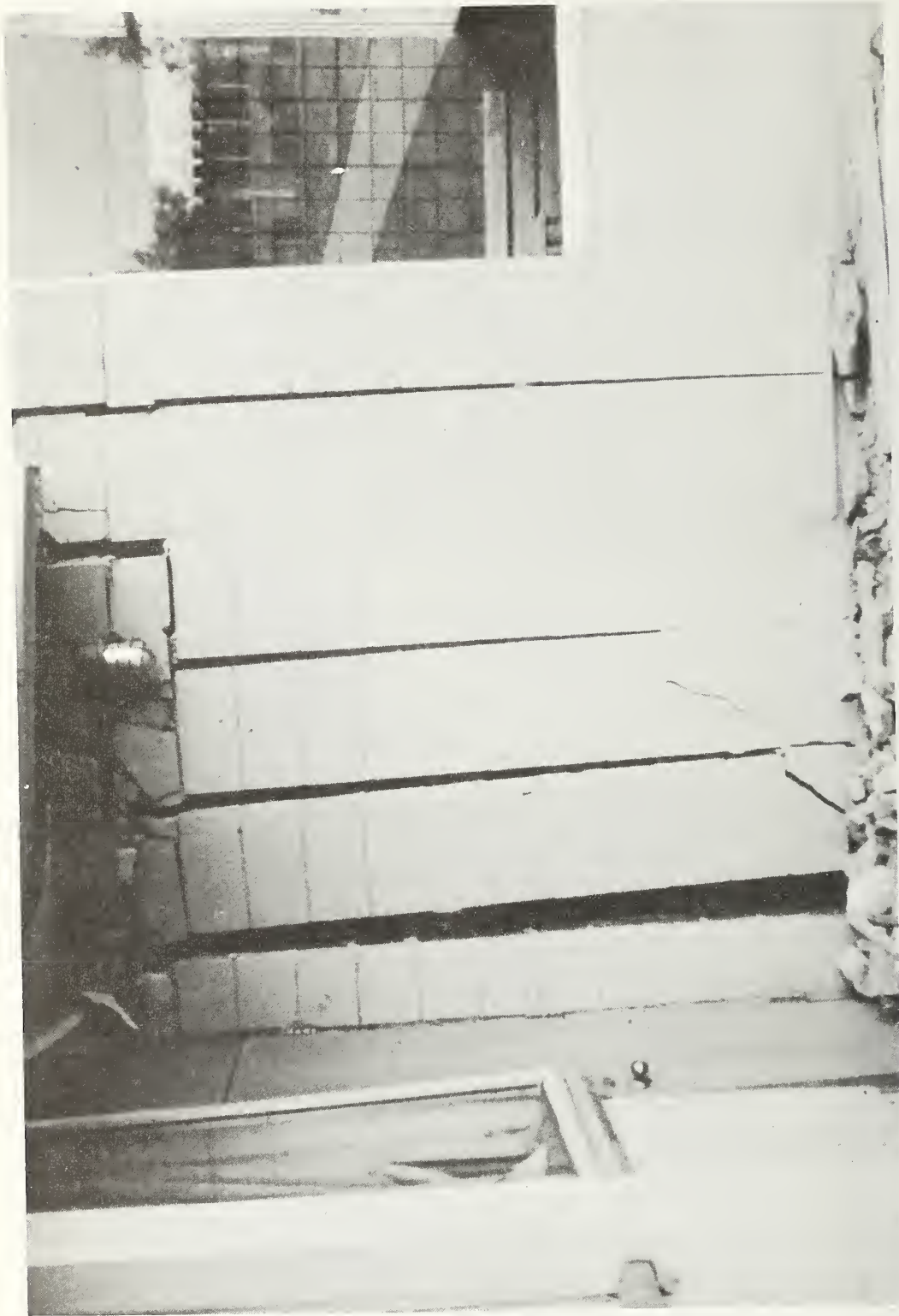
Figure 6.51 Damage to concrete block wall, Los Angeles County Juvenile Facility. Note absence of horizontal reinforcement. Only reinforced vertical cells are filled with grout.
