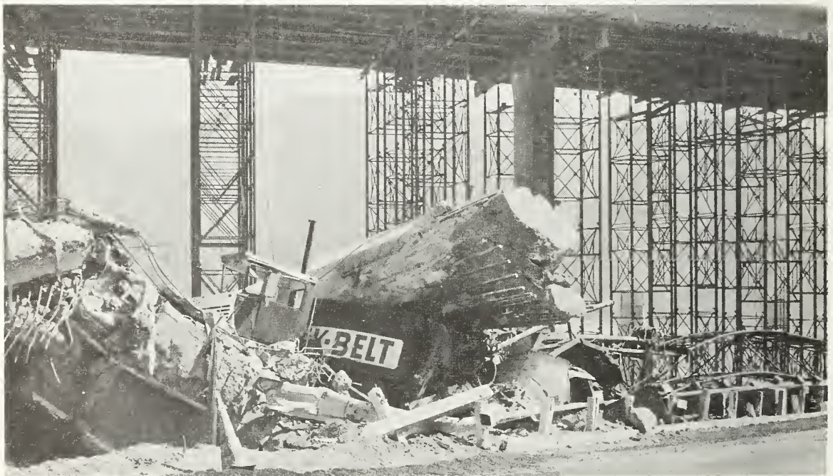
Figure 7.9 The top of Pier 5, which was embedded in the girder diaphragm, resting on the construction crane after collapse.
