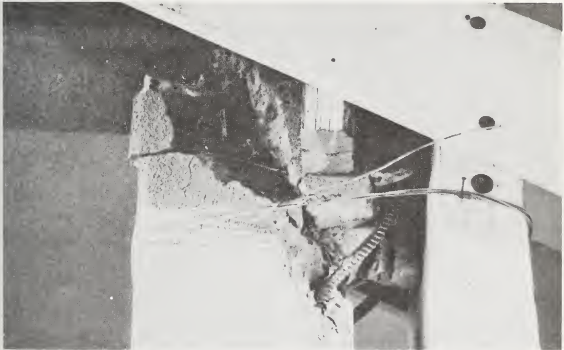
Figure 6.23 Close up of fractured concrete second-story covered arcade column, Patrick Henry Jr. High School.
