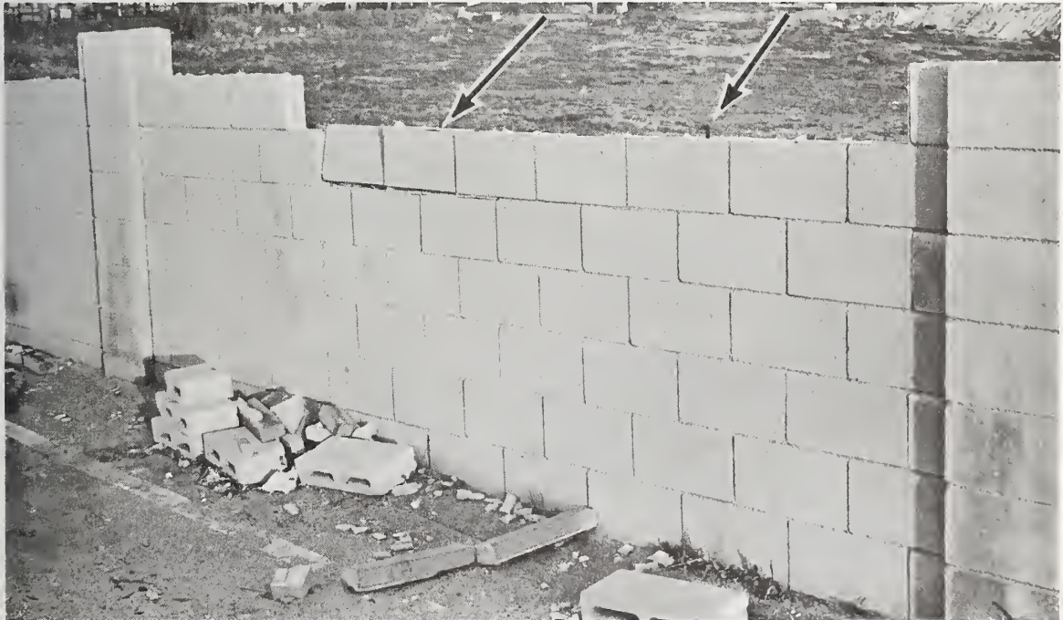
Figure 5.155 Reinforced concrete masonry wall around the Medical Center parking lot. Arrows indicate the location of vertical reinforcement.
