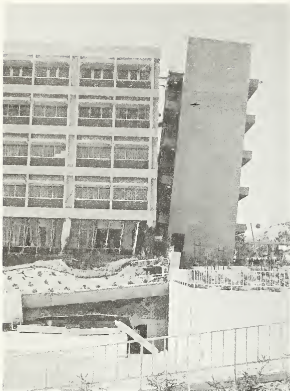
Figure 5.34 Tipped stair tower at the end of Wing C. This is the only stair tower that did not topple. This stair tower is supported directly on the foundation; whereas, the other three towers were supported on the ground-story columns.
