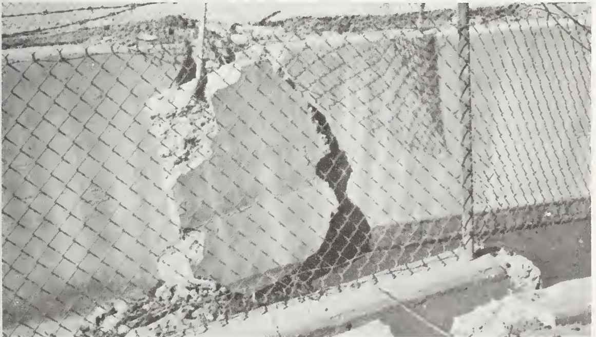
Figure 8.35 Lopez Canyon Channel. A 2-foot displacement of the channel had caused complete failure of the walls and invert, with the upstream portion moving over the downstream portion.
