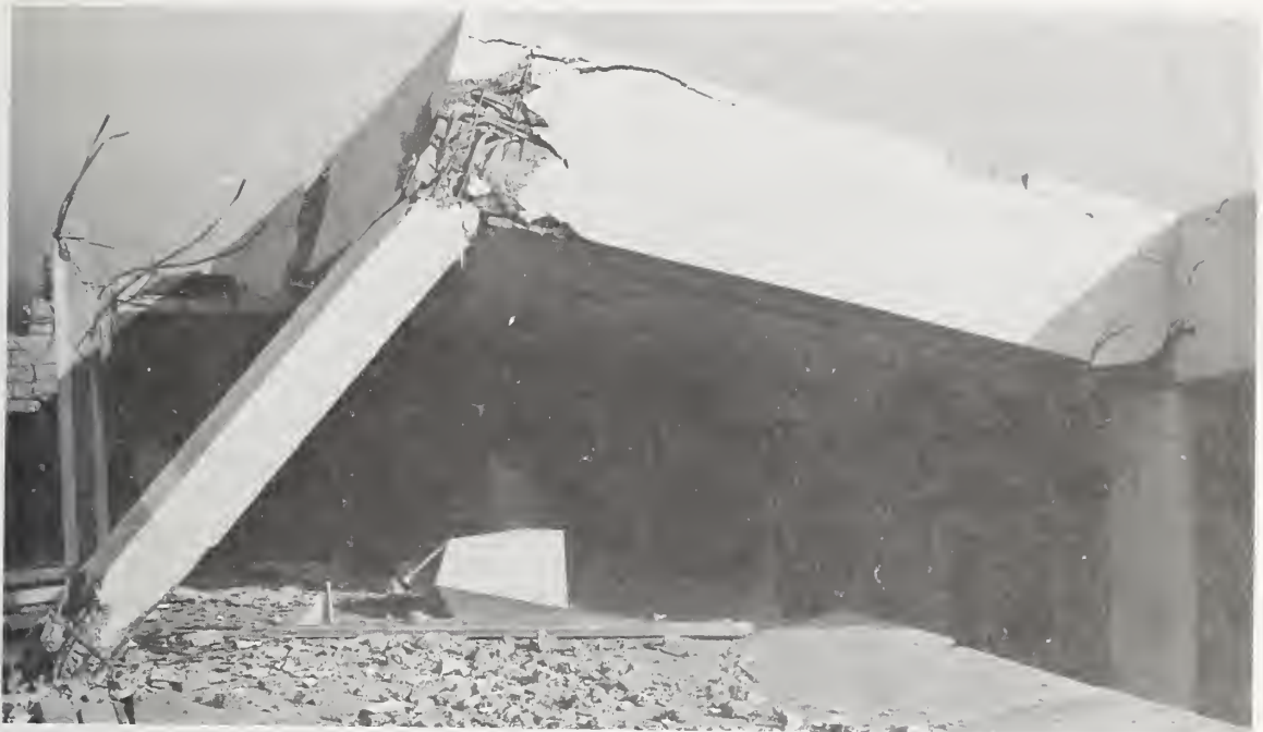
Figure 5.13 Damage to the canopy at the front (north) entrance to the Psychiatric Unit.
