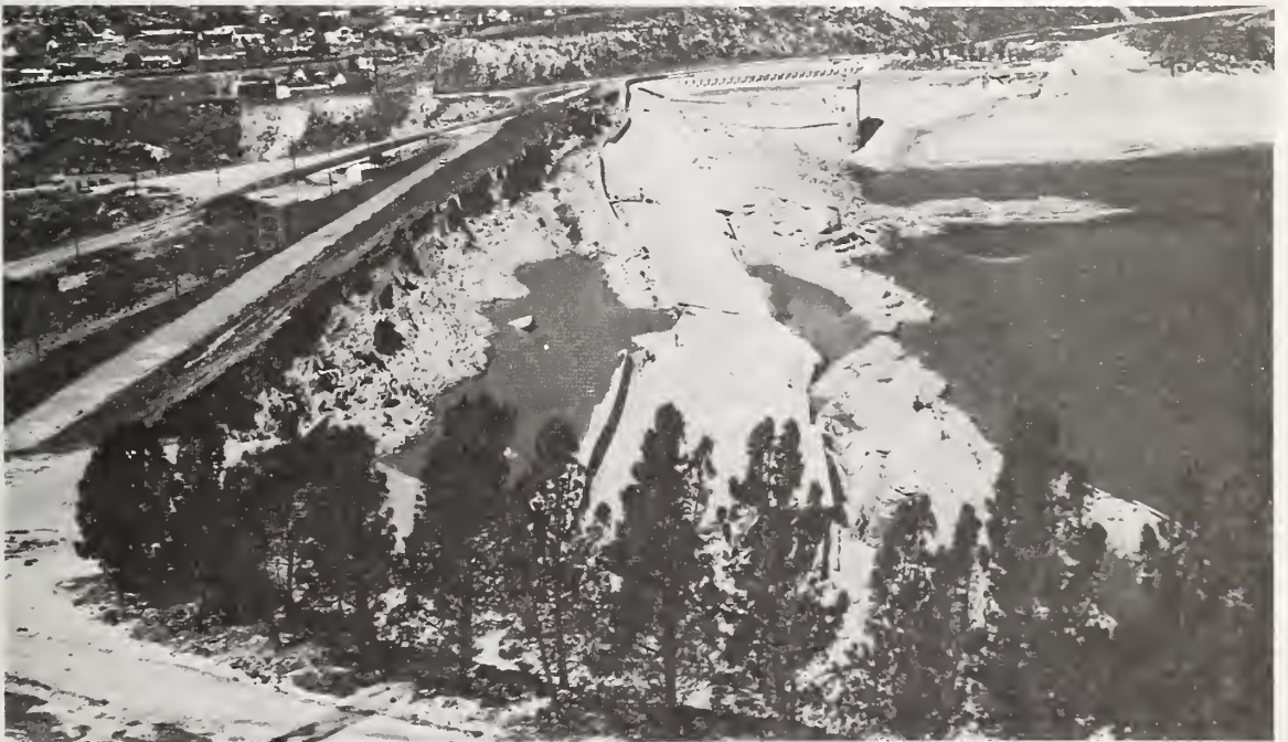
Figure 4.7 Collapsed liner of Lower San Fernando Dam.
