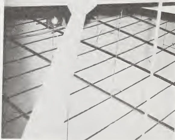
Figure 6.21 Buckled 5 x 3 angle brace, San Fernando High School.
