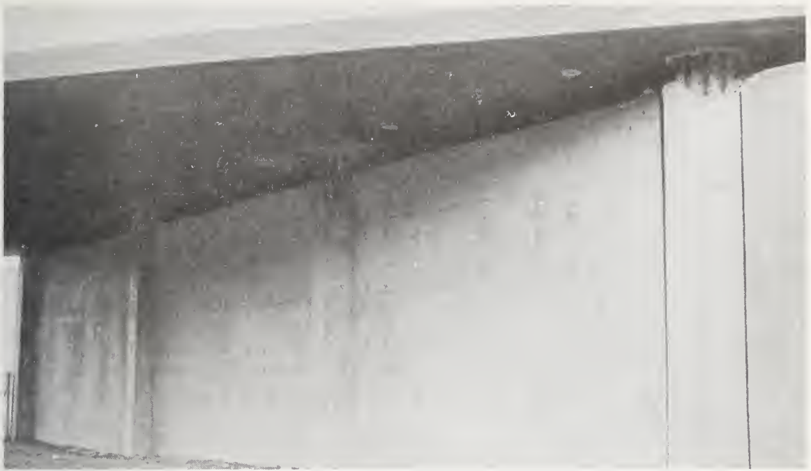
Figure 7.28 Damaged columns in bent 4 with 10-in closure wall which was separated from the columns by 1/2-in filled expansion joints.
