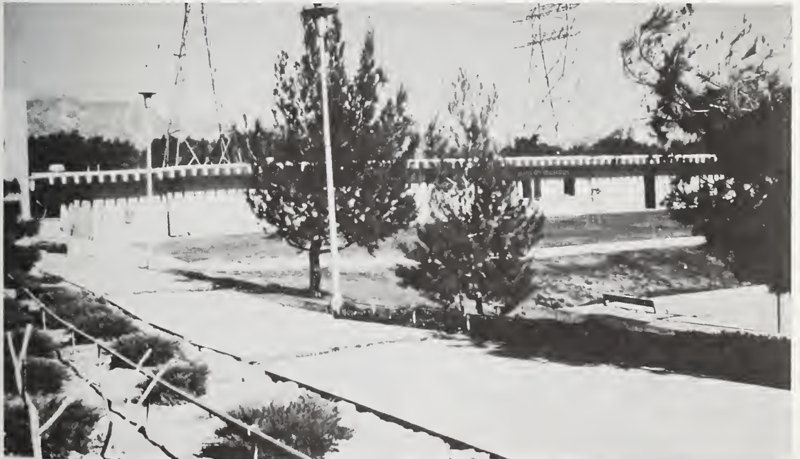
Figure 6.41 West wall of girls' school, Los Angeles County Juvenile Facility. Note displacement at left (north) end of building and severe ground rupture (see figure 6.48).
