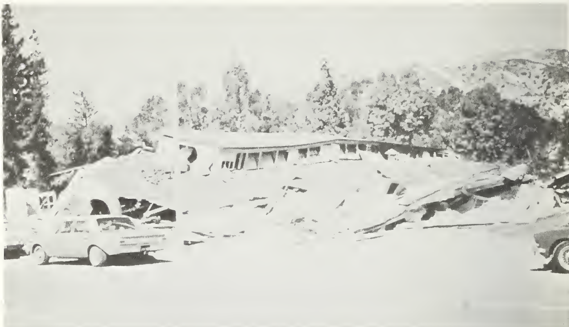
Figure 5.40a Totally collapsed old brick building at the old section of the Olive View Medical Center. The building was not designed to resist earthquake forces.
