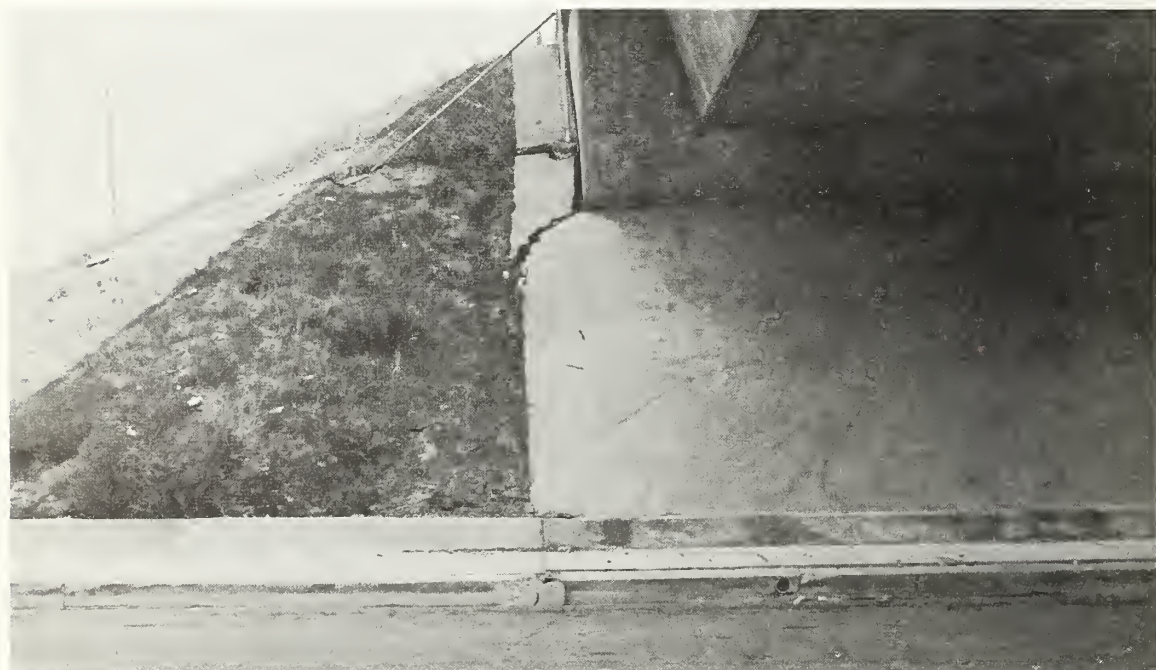
Figure 7.33 Typical damage to wing walls and sloped paving on a single span prestressed concrete box girder bridge.
