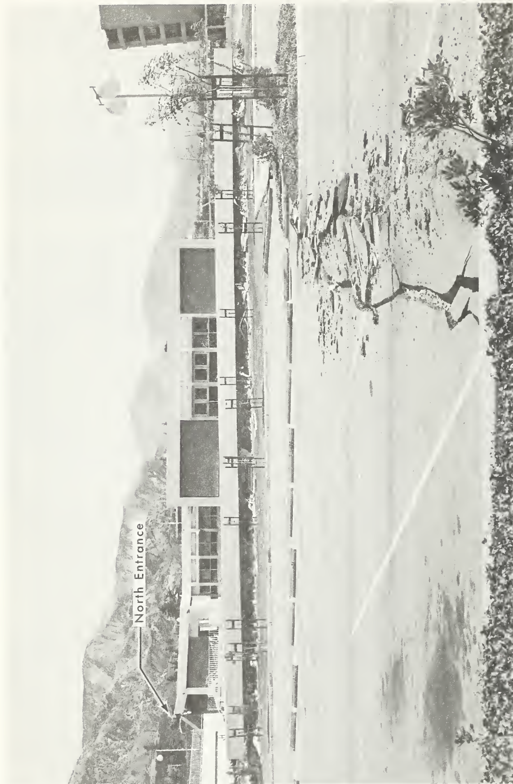
Figure 5.12 West elevation of the Psychiatric Unit. Damage to the surface of the parking lot, just west of this building, indicates severe ground movement.
