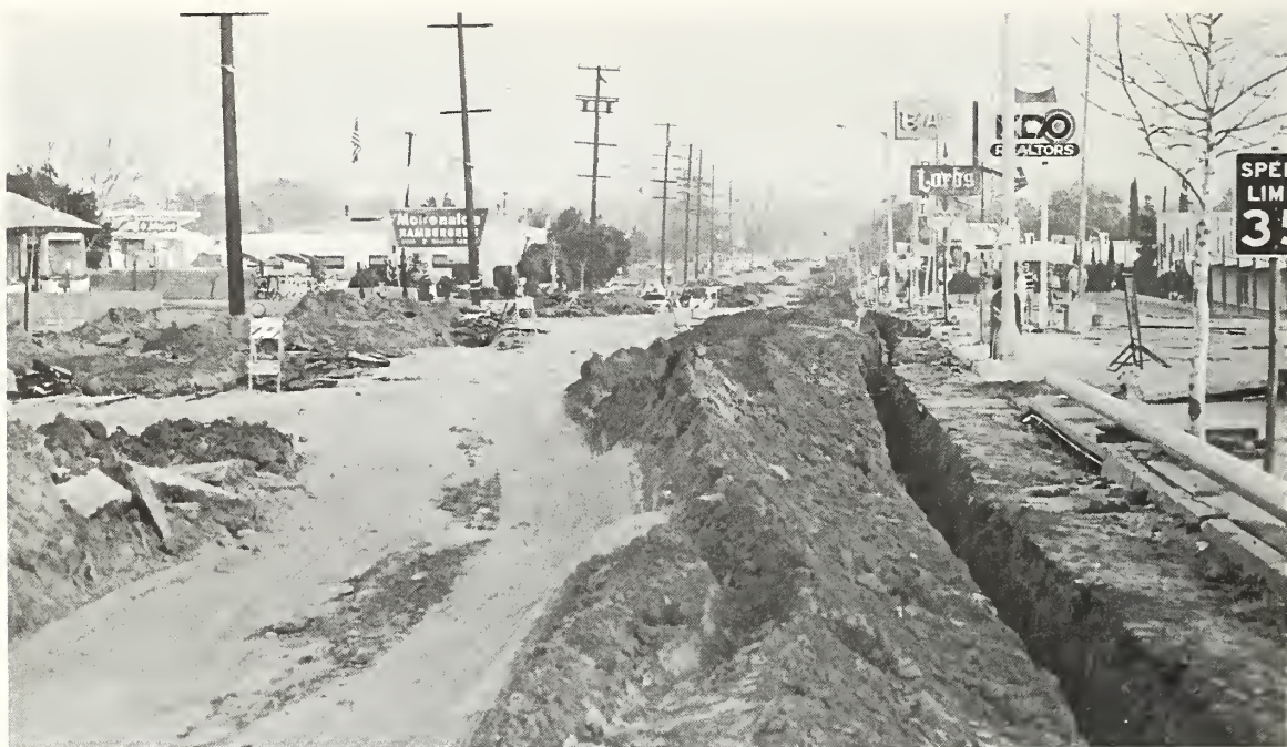
Figure 7.39 Broken gas, water, and sewer lines being repaired near intersection of Hubbard Avenue and Glenoaks Boulevard, San Fernando.
