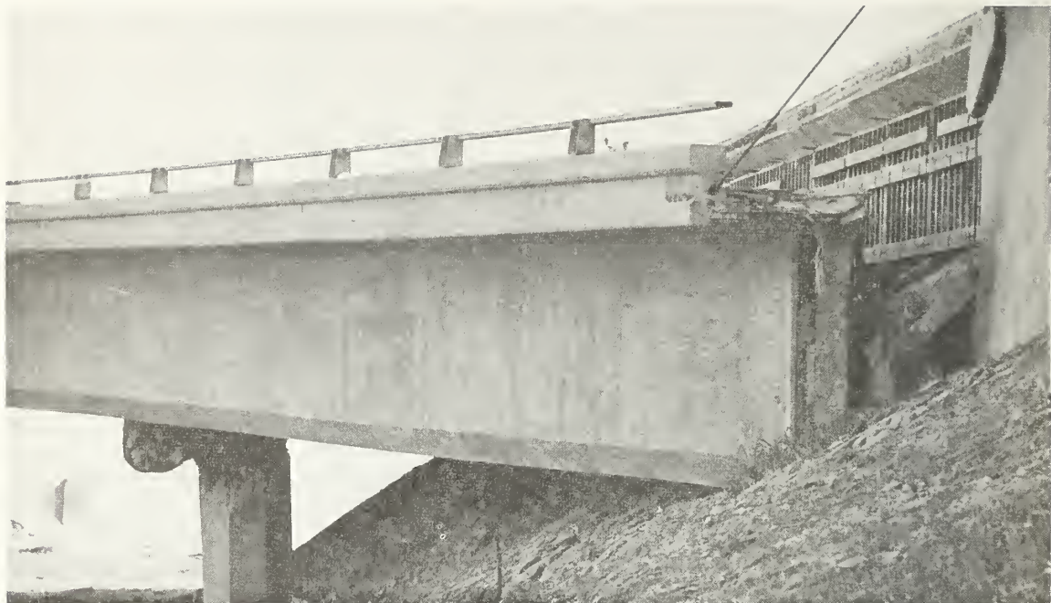
Figure 7.22 Abutment and pier damage at the western end of the Northwest Connector Overcrossing.
