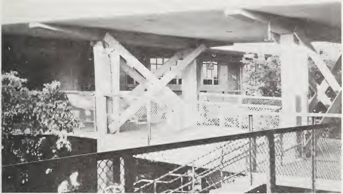
Figure 6.22 Fractured concrete at second-story covered arcade columns, Patrick Henry Jr. High School.
