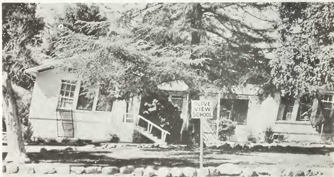
Figure 5.40b Severely damaged pre-1933 wood-frame structure at the old section of the Olive View Medical Center.
