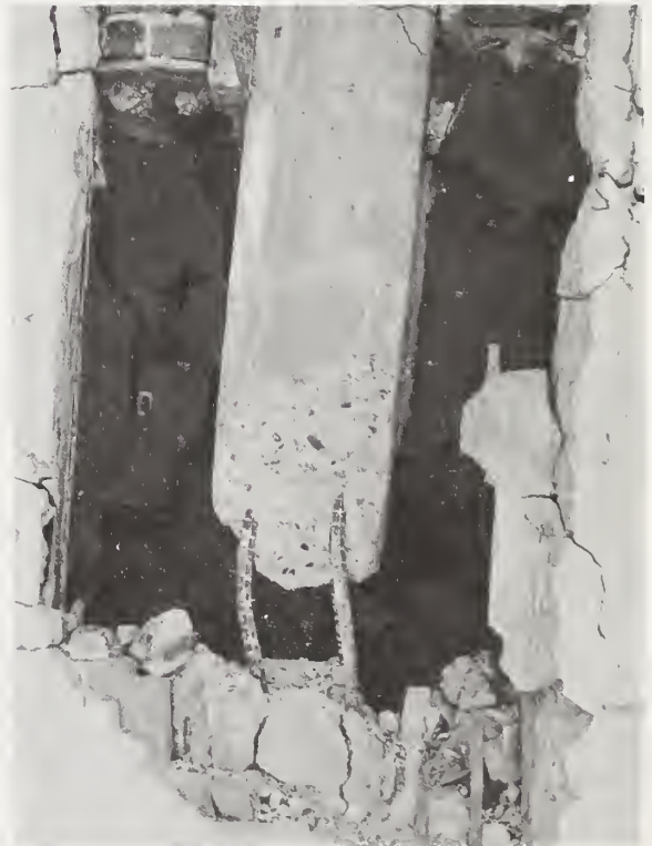
Figure 5.50 Close-up view of one of many damaged columns in Building 6. Note a lack of ties around the exposed square reinforcing bars.
