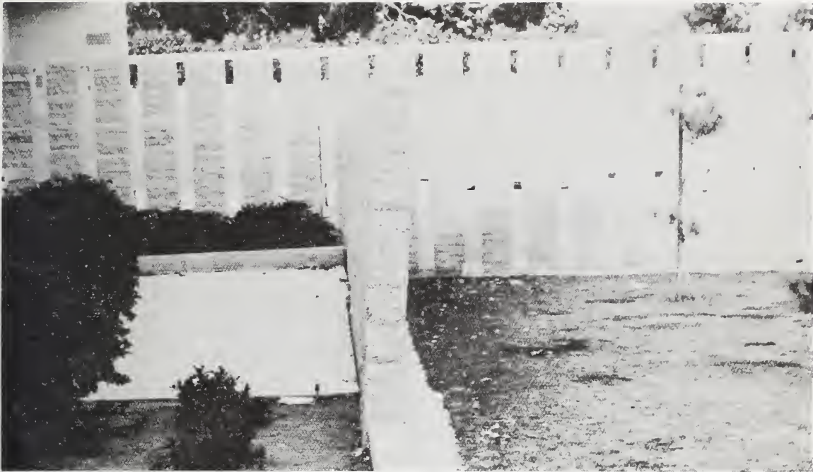
Figure 6.14 Cantilever concrete block garden wall leaned approximately ten degrees, Van Gogh Street School.
