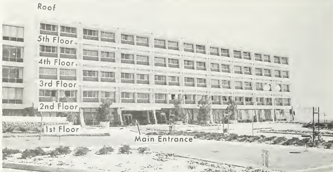
Figure 5.18 West face of Wing A. Note the extensive damage at the first floor and the lateral displacement of the building to the north. Most glass was intact in windows above the third floor.
