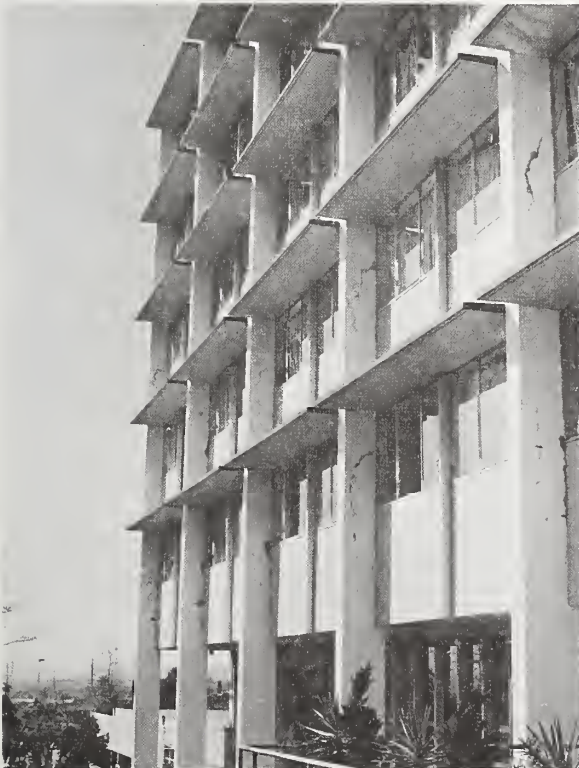
Figure 5.56 Aerial view of Holy Cross Hospital. This 209-bed, reinforced concrete structure was badly damaged and has been evacuated.
