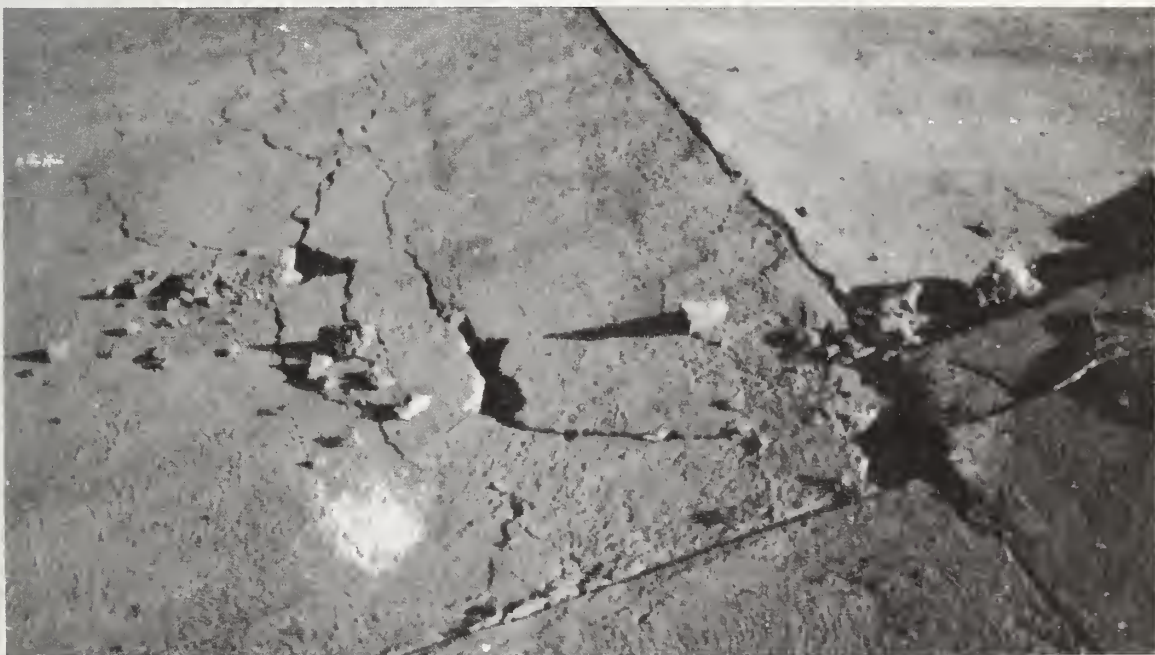
Figure 8.31 Looking easterly showing damage to facing slab; Stetson Debris Basin.
