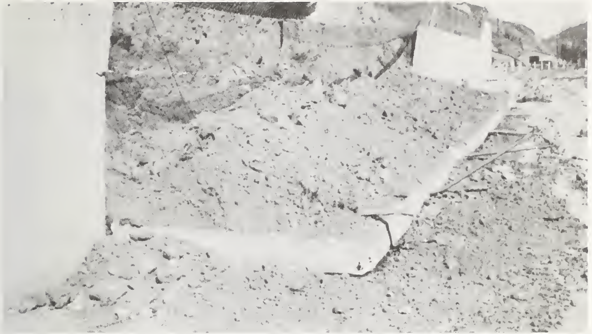
Figure 8.34 Lopez Canyon Channel. A 50-foot section of the wall has failed on the right bank. The 50-foot section adjacent upstream also shows severe structural damage.
