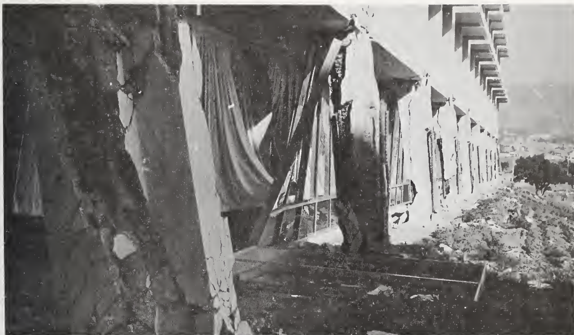
Figure 5.26 South row of first story columns, in Wing D; note the lack of ties on the corner bars which have broken out of the columns.
