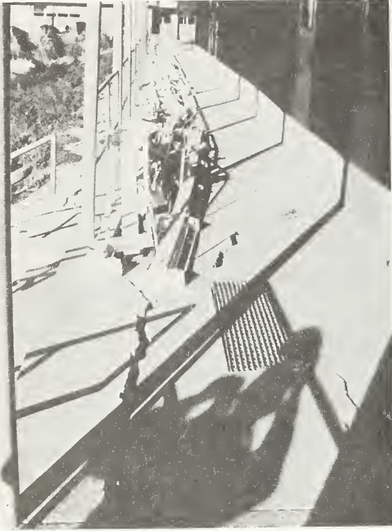
Figure 6.59 Arcade pipe columns were displaced at base where slab on grade pulled apart, Camp Karl Holton. (Damaged lighting fixtures were removed from buildings and stored on walkway.)
