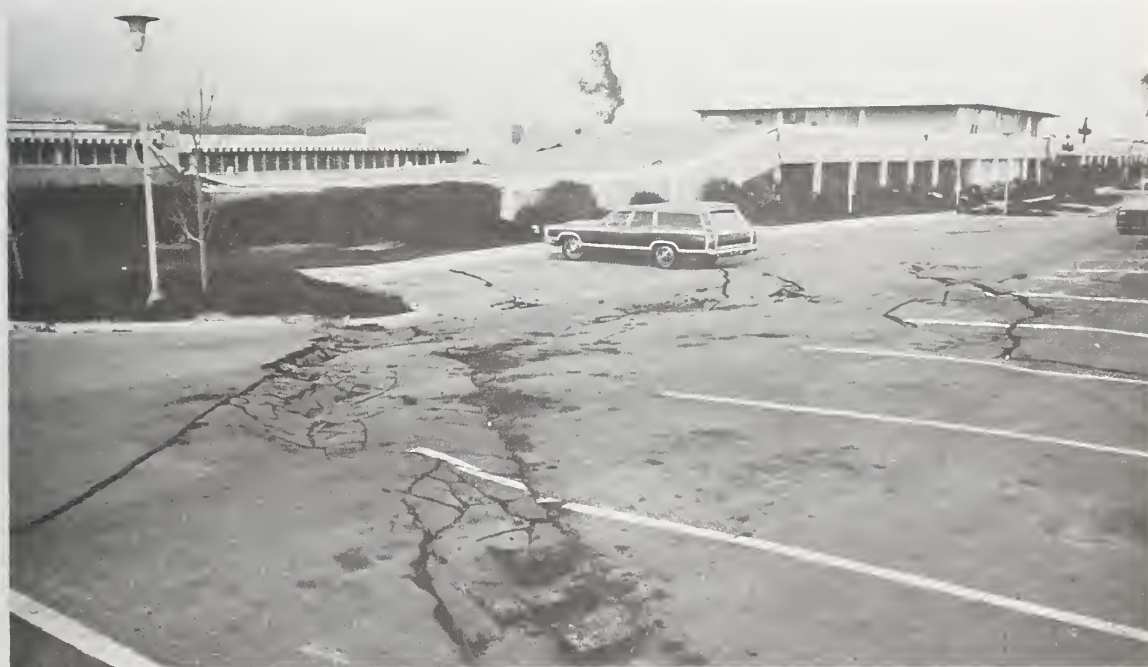
Figure 6.37 A portion of the Administration Wing collapsed at the Los Angeles County Juvenile Facility. Note the distortion of the ground surface.
