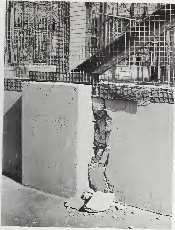
Figure 8.12 Concrete spalling at one of the joints between a column pedestal and an enclosure wall surrounding the electrical transformer yard.
