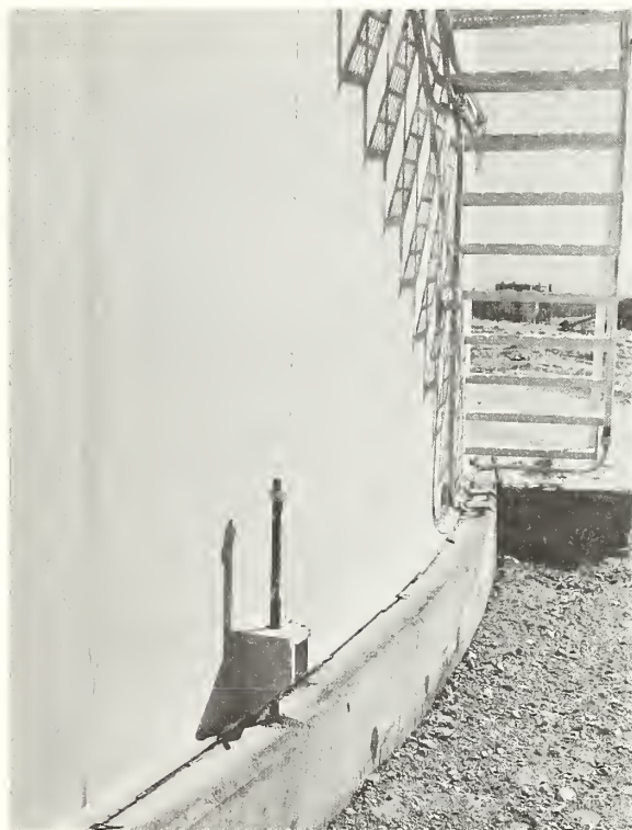
Figure 8.6 Vertical Movement of tank pulled one-inch diameter anchor bolt out of concrete base.
