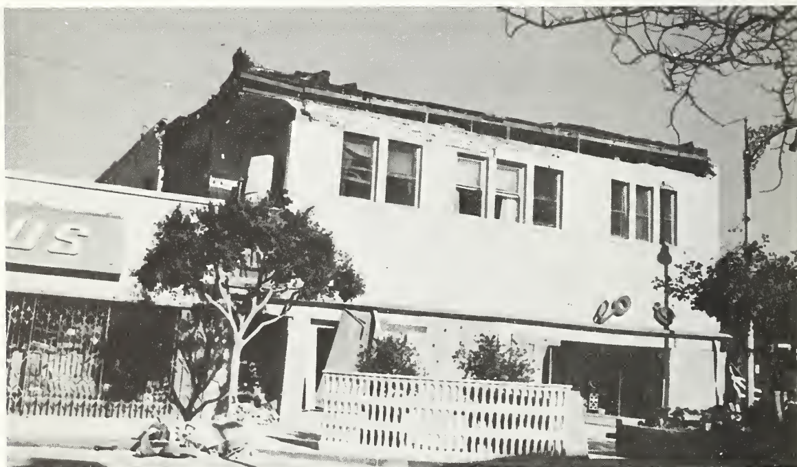
Figure 5.143 Collapsed wall and parapet.
