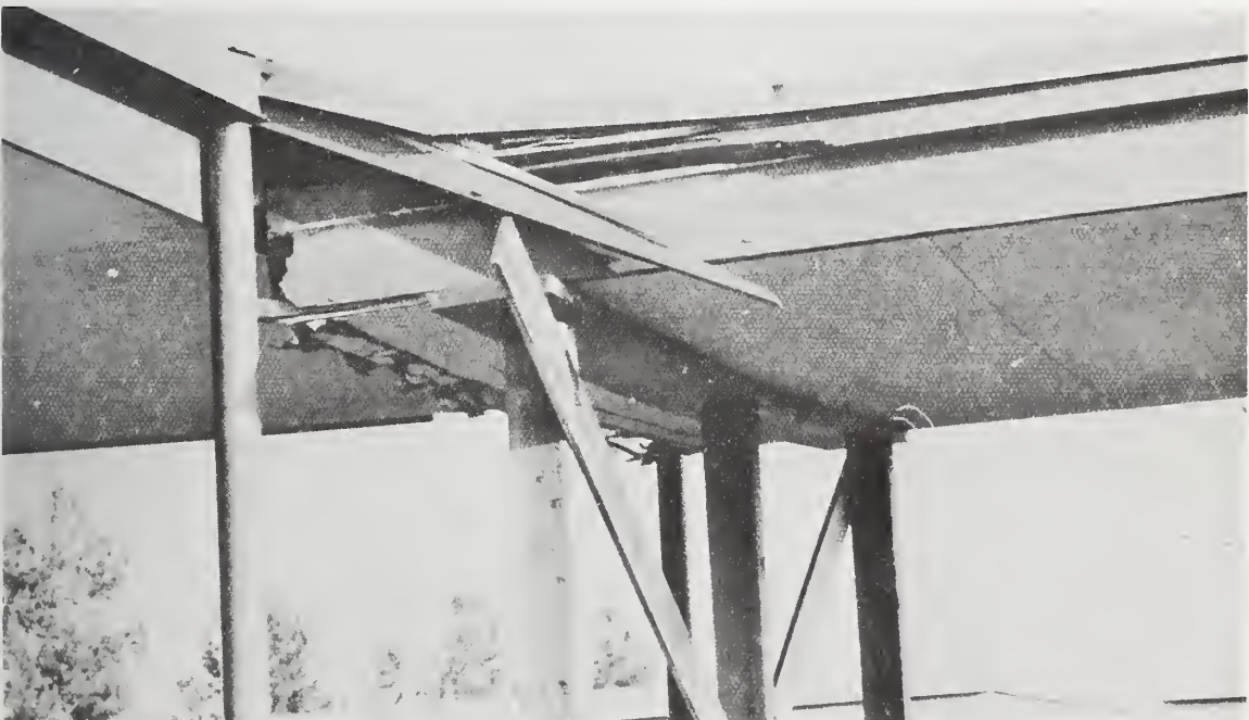
Figure 6.15 Arcades pulled loose from each other at Sylmar High School.
