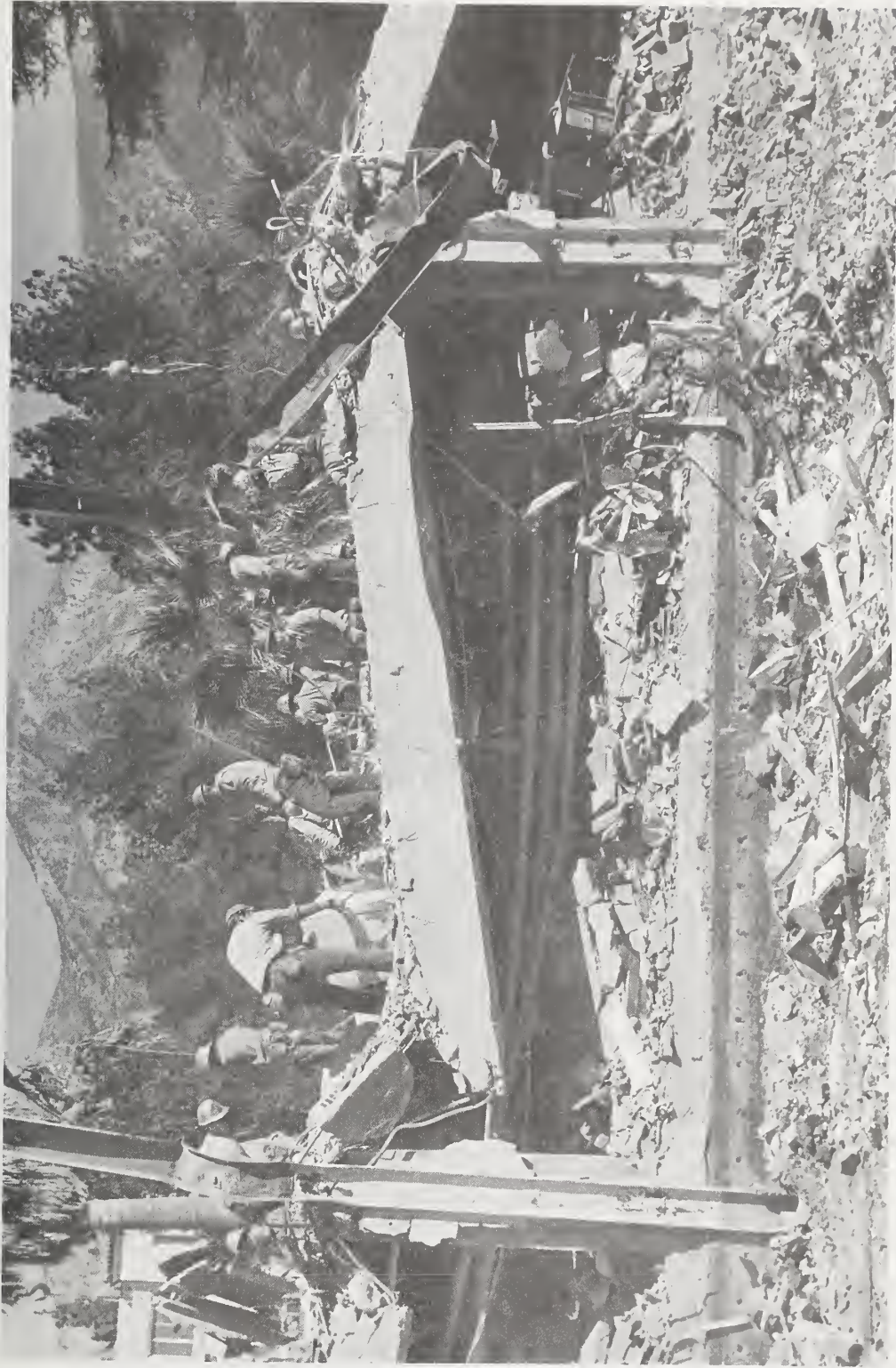
Figure 5.42 Rescue and clean-up operations. This collapsed building was constructed in 1925 and is a reinforced concrete frame structure infilled with unreinforced clay tile walls. (Los Angeles Times Photo).
