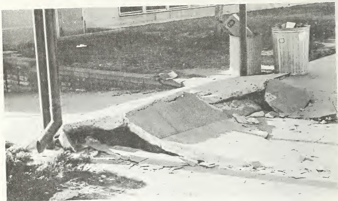
Figure 6.18 Slabs on grade were extensively cracked and buckled, Sylmar High School.
