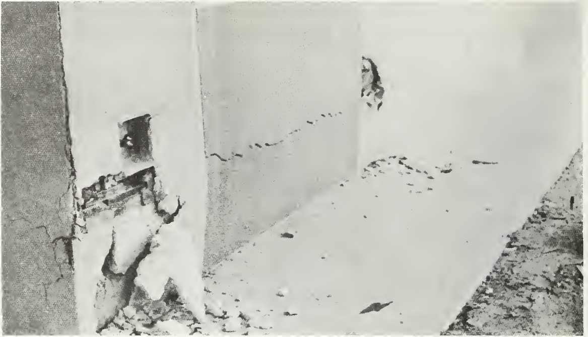
Figure 6.12 Displaced bearing wall, Van Gogh Street School.
