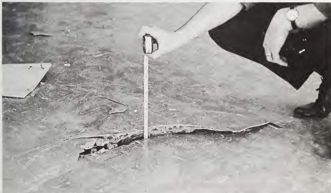
Figure 5.66 Floor cracking at the west end of the third floor. The floor is concrete pan-joist construction with a 3-in. slab.
