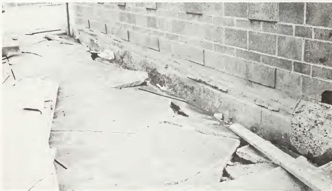
Figure 6.58 Approximately 6 inches of vertical displacement between masonry classroom building and the portable classroom building, Camp Karl Holton.
