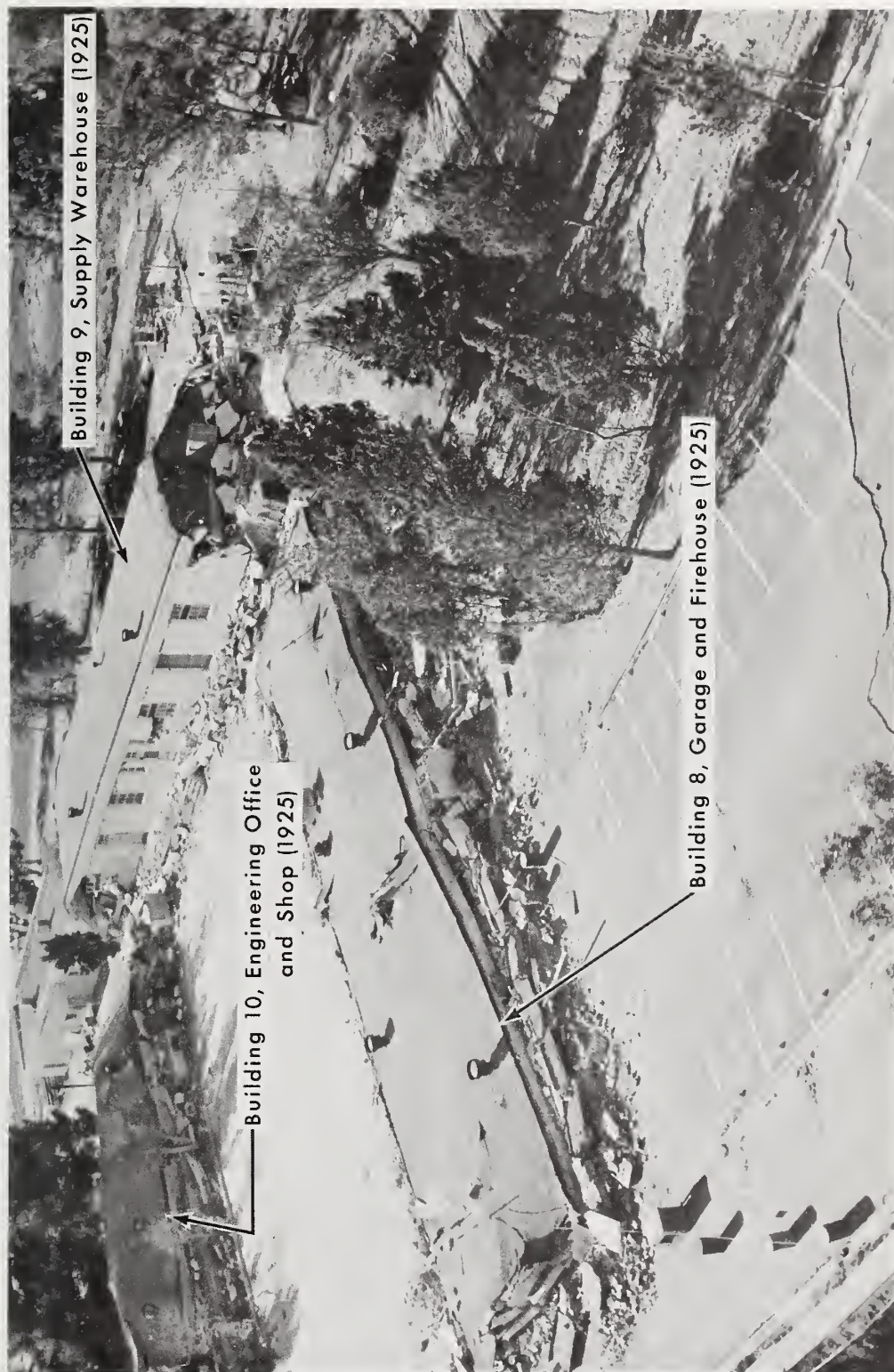
Figure 5.45 Collapsed one-story buildings (No. 8 and 10) located at the east end of the hospital complex. Note that two structures oriented in one direction collapsed; whereas, the building (No. 9) oriented 90 degrees to them is damaged but still standing.
