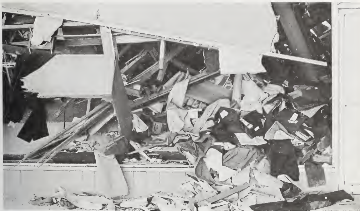
Figure 5.140 The wall of the building shown in figure 5.139 fell through the roof of this building.
