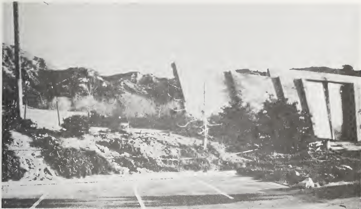
Figure 6.55 A portion of perimeter security wall has fallen; some is severely tilted, Camp Karl Holton.
