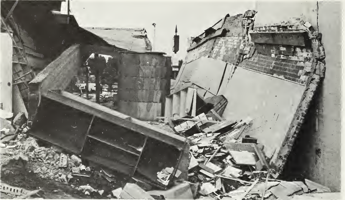
Figure 5.134 Collapsed side wall shown in figure 5.133 as viewed from the rear of the store.
