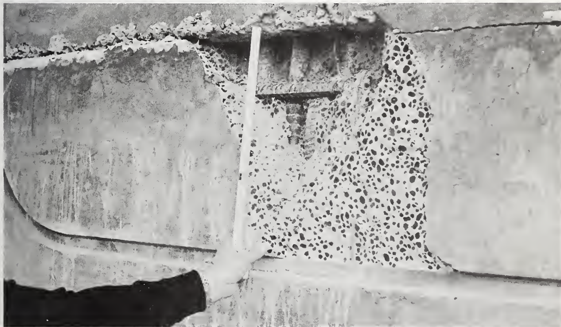
Figure 5.177 Damage to the exterior surface of the concrete wall along the construction joint.
