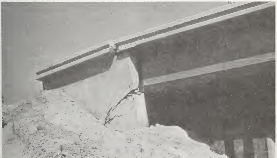
Figure 7.29 Typical abutment damage.
