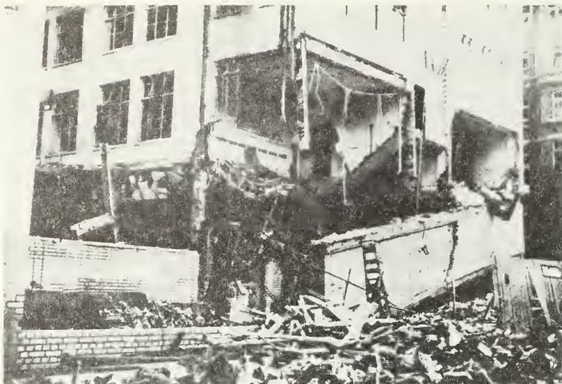
Figure 2 Detail of a Seven-Story-Steel-Framed Building After a Wartime (World War II) Bomb.
