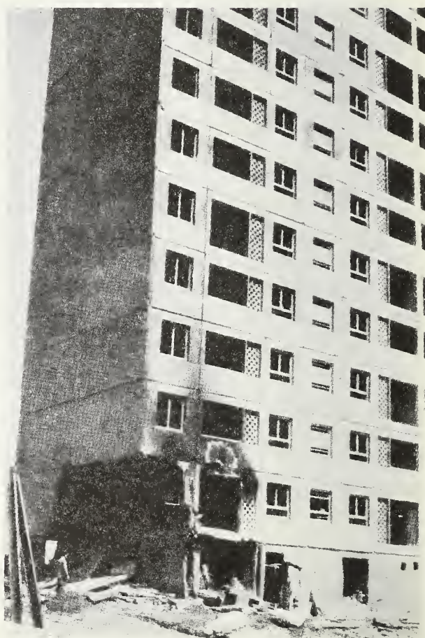
Figure 3 Concrete Panel Building in Algeria Damaged by an Explosion.
