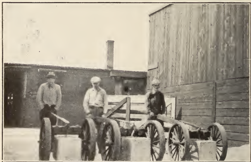
FIG. 5.—Moving 1,000-pound test weights with special carts
