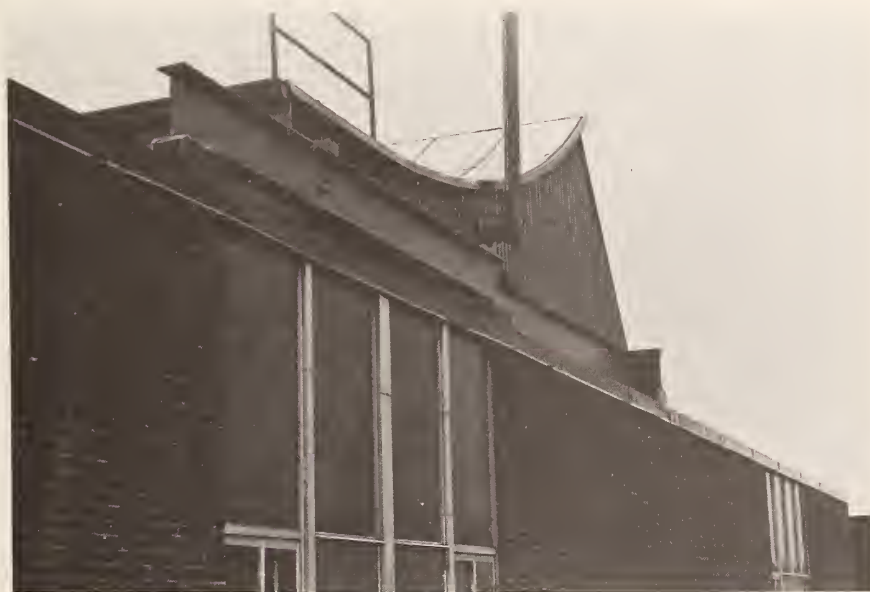
Figure C.6 Large Wooden Reflector Frame Supported by Exterior Walls and Columns of the Building
