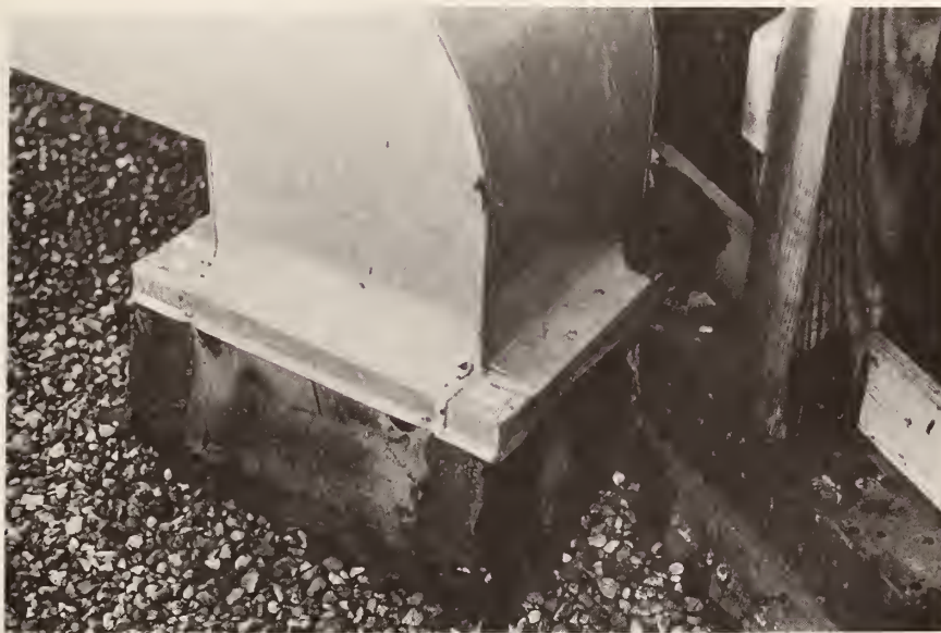
Figure 22. Modification of a Curb Supporting a Ventilator
