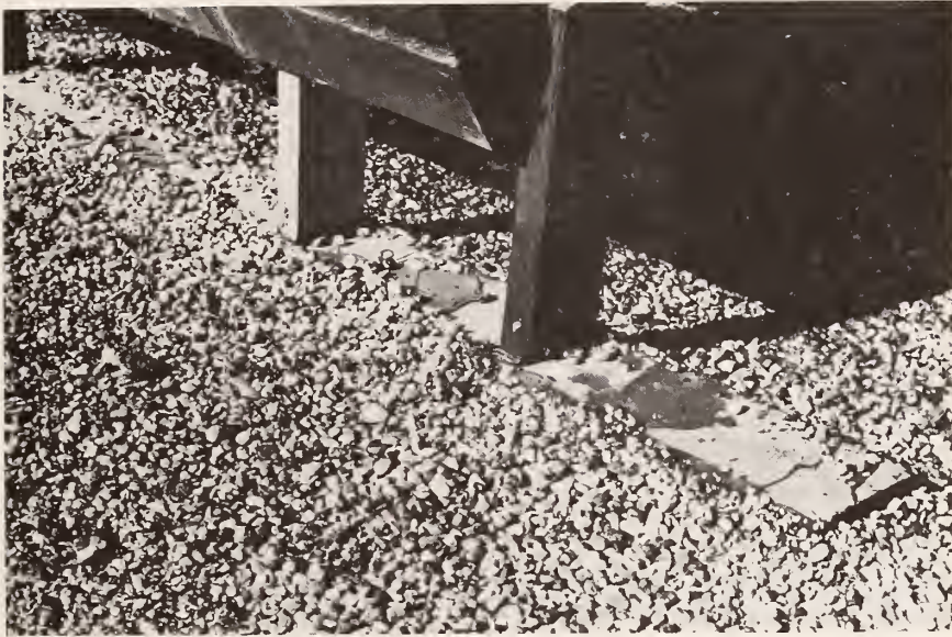
Figure C.13 Sleeper Which Had Sunk into Asphalt Flood Coat and Aggregate Surfacing
