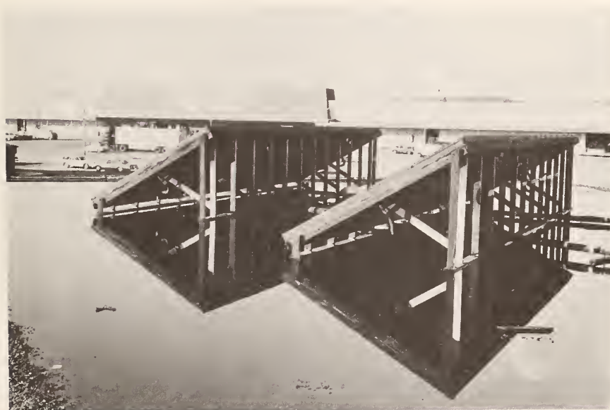
Figure C.2 Ponded Water Over 2 inches (50 mm) Deep Around Collectors
