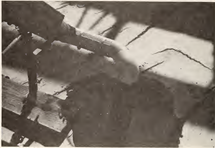
Figure C.15 Excessive Quantity of Asphalt Around Pipe Penetration With Undetermined Type of Flashing
