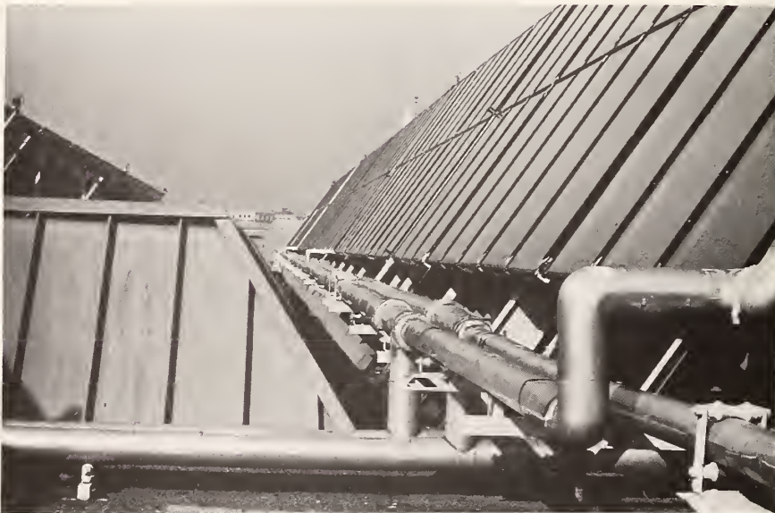
Figure C.20 Inadequate Clearance Between Front of Collector Array and a Mansard Style Roof Projection
