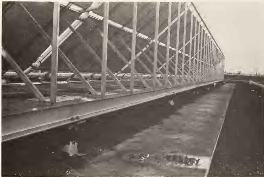
Figure C.31 Coated Felt Walkway on Roofing
