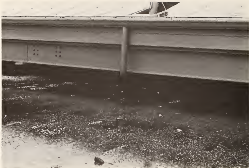
Figure C.3 Ponded Water on Roof Surface Extending Under Large Wooden Platform Supporting Solar Reflectors
