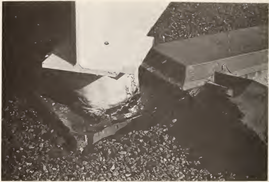
Figure C.23 Penetration of Collector Support Column at the Edge of the Roof
