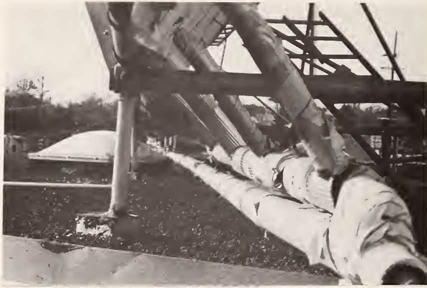
Figure C.19 Piping Located Close to Roof Surface
