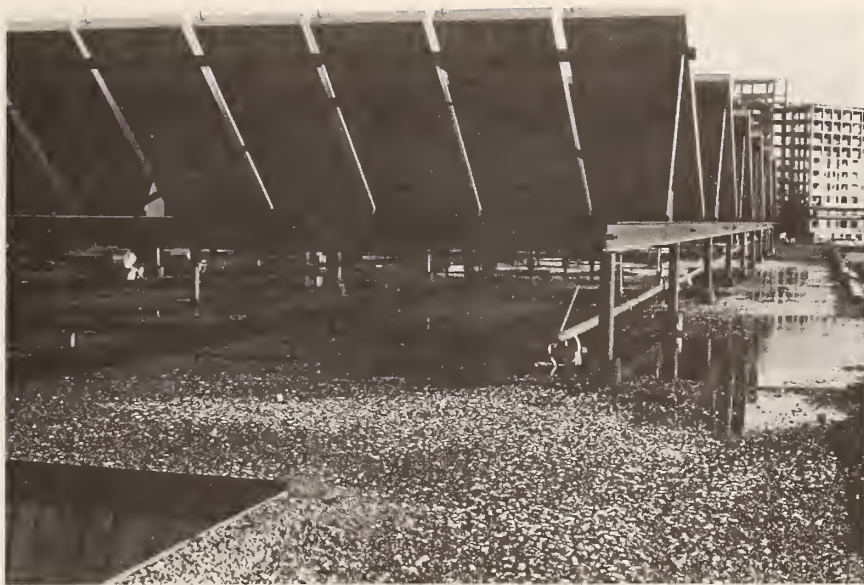
Figure C.1 Ponded Water Under Solar Collectors
