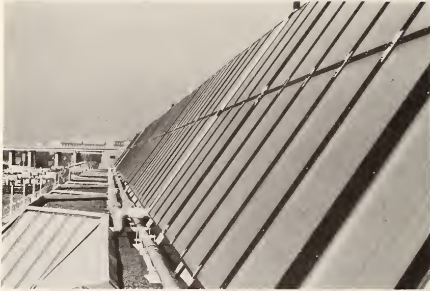
Figure C.27 Collector Array Installed Near Roof Edge
