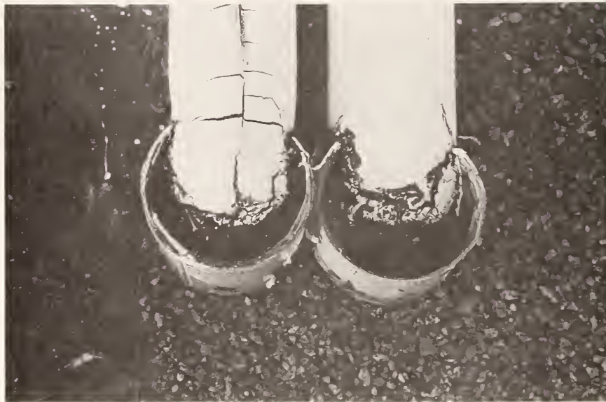
Figure C.16 Pitch Pockets for Pipe Penetrations
