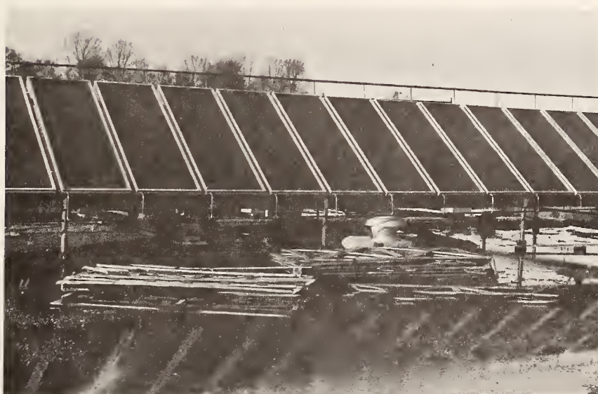
Figure C.34 Debris On Roof from Solar Installation
