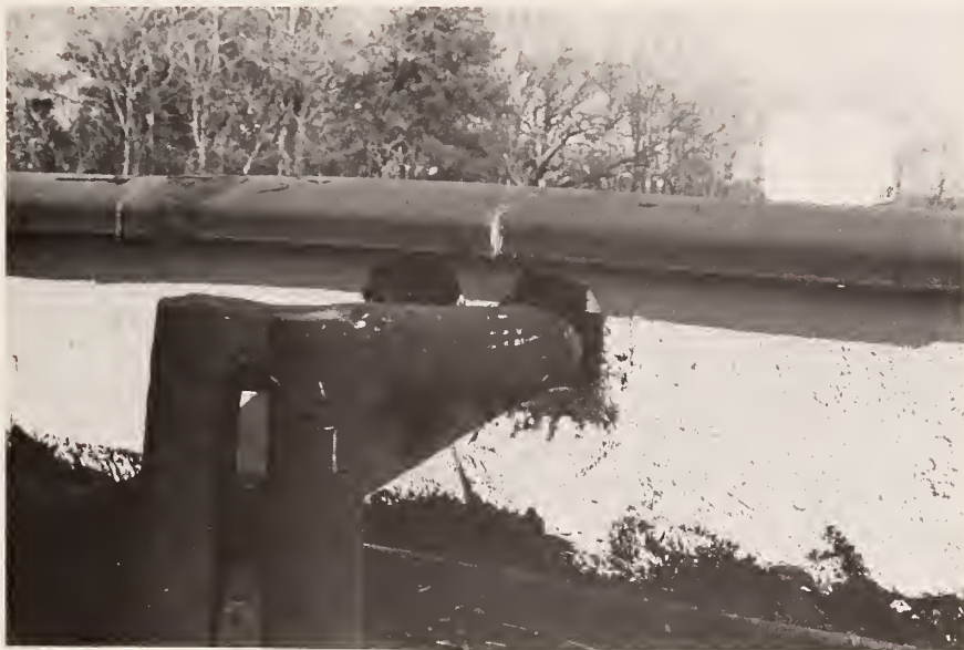
Figure C.29 Fire Wall Penetrated by Solar Piping
