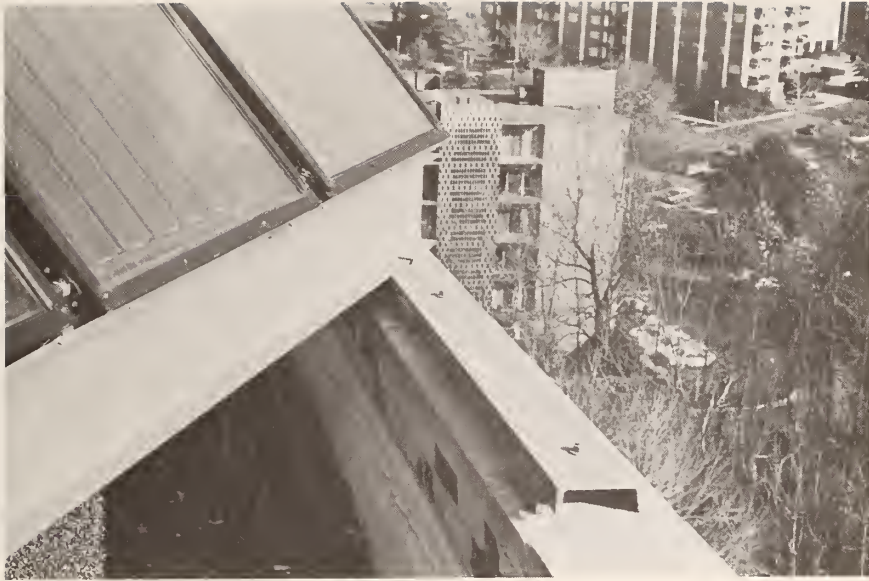
Figure C.9 Attachment of Collector Support Beam Using a Steel Clip Welded to a Channel which is Bolted to a Parapet Wall
