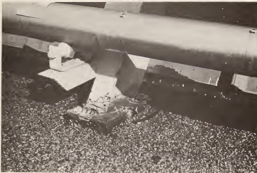
Figure C.25 Pipe Roller Support Attached to Collector Frame
