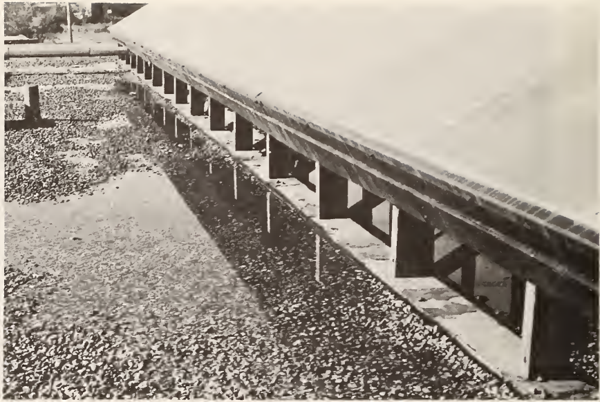
Figure C.11 Wooden Sleeper Mechanically Attached to Roof
