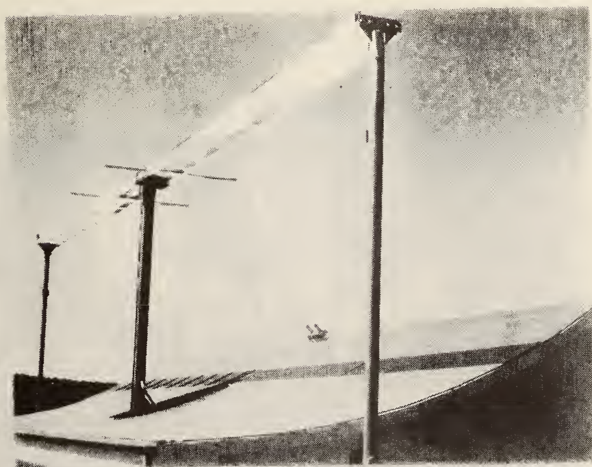
Figure 2-30. Concentrating Collector with Roof Mounted Reflective Surfaces
