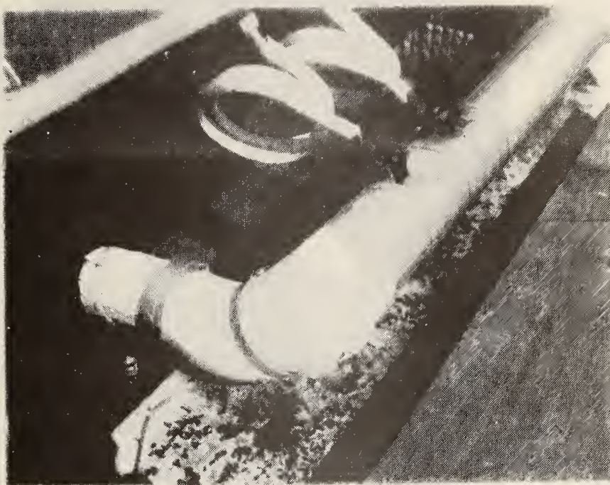
Figure 2-33. Copper Coil Replacement of Flexible Hoses
