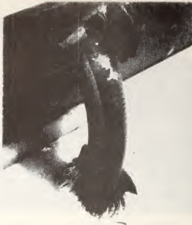
Figure 2-35. Uninsulated Flexible Coupling
