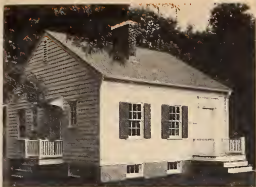
Left: test bungalow constructed at the Bureau for research in heat transfer phenomena in small houses. This bungalow has since been completely enclosed within an insulated enclosure (right) so that the temperature outside of the house can be maintained at any temperature condition encountered throughout the United States.
