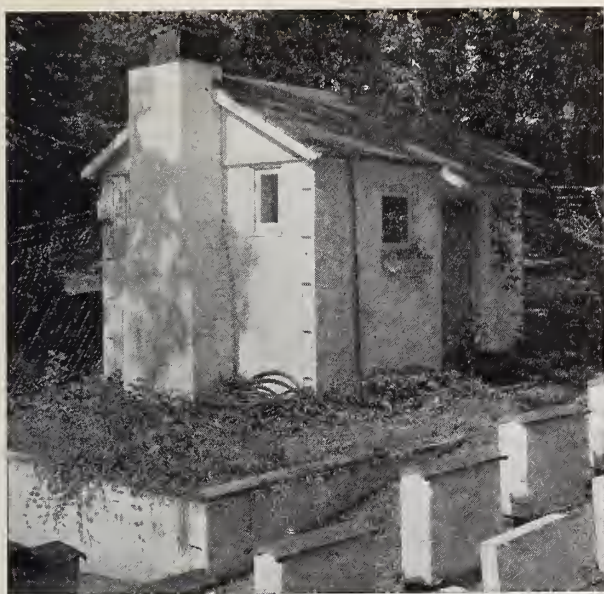
FIGURE 2.—Field office with cinder-concrete block walls and chimney of new common brick.
