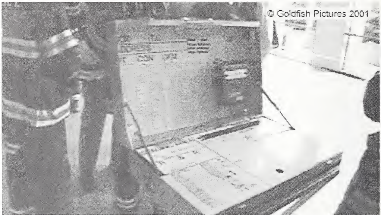
Figure 5–6. Video image of the FDNY Fire Command Board located in the lobby of WTC 1.
