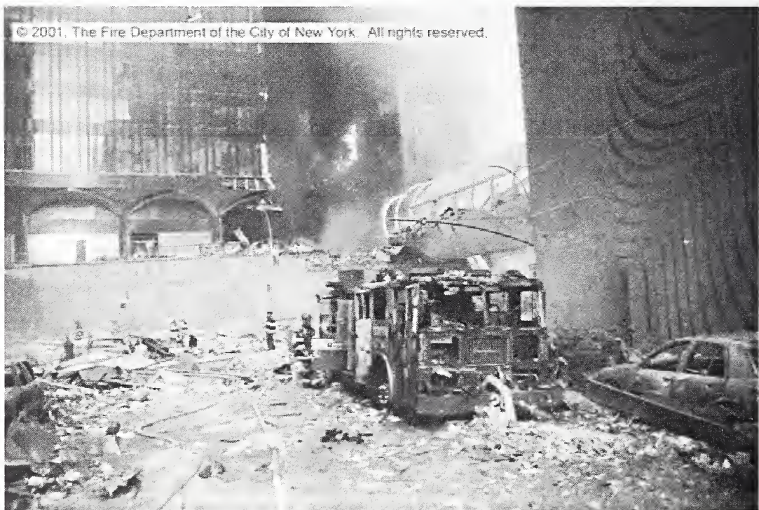
Figure 5–18. Burned out fire apparatus on West Broadway next to WTC 7 following the collapse of WTC 1 and 2.
