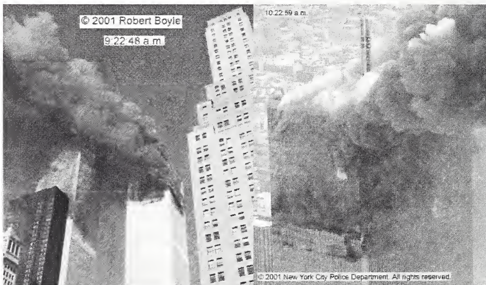
Figure 5–2. Photographs of smoke covering the roofs of the World Trade Center buildings
