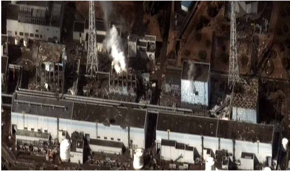
Figure 2 (a). Fukushima Daiichi nuclear disaster, 16 March 2011, showing the four tall damaged reactor buildings with much of the damage caused by hydrogen–air explosions, Fukushima, Japan Source: https://en.wikipedia.org/
