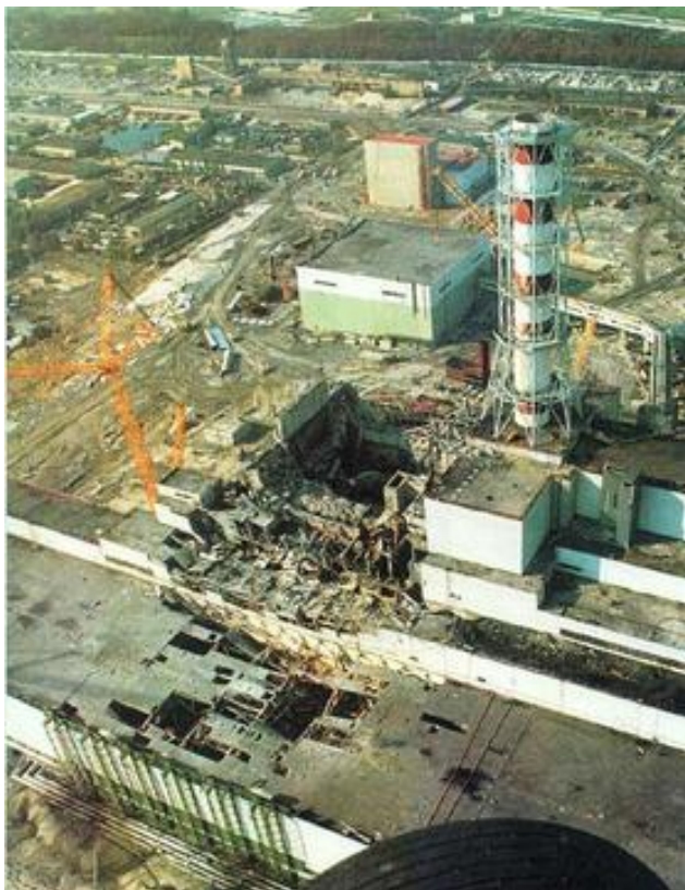
Figure 2 (b). The Chernobyl nuclear reactor after the disaster. Reactor 4 (center). Turbine building (lower left). Reactor 3 (center right), on 26 April 1986, Pripjat, (former Ukrainian SSR, Soviet Union) Source: https://en.wikipedia.org/
