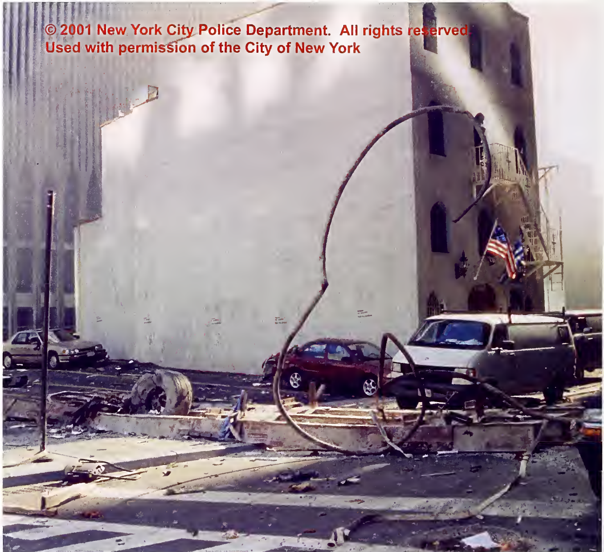
Figure H-14. Photograph showing a full panel section lying in Cedar Street near its intersection with West Street. An aircraft wheel can be seen imbedded in one of the windows. The building behind the panel is Saint Nicholas Greek Orthodox Church and the lower section of WTC 2 can be seen across Liberty Street.
