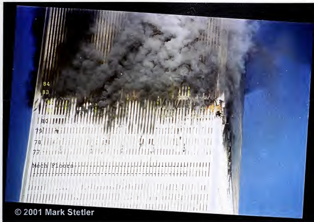
Figure H-6. Photograph taken at 9:26:20 a.m. on September 11, 2001, showing the east face of WTC 2. It has been enhanced, and lettering indicating floors and columns has been added.
