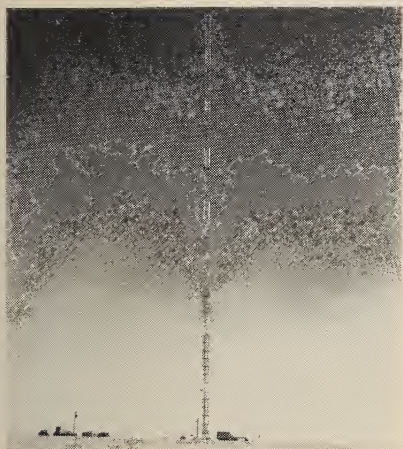
This 500-foot tower at Haswell, Colorado, shown at left is used in studying "tropospheric scatter propagation", the transmission and reception of VHF and UHF signals beyond the line-of-sight. Data for worldwide radio noise predictions are obtained from field recording stations like the one at right located near Boulder, Colorado (p. 108).
