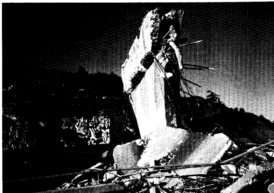
Figure 4.12. Damage at Pier 3 of the SR14/I5 Separation and Overhead, Ramp C, looking to the west (Photo courtesy of EERC).
