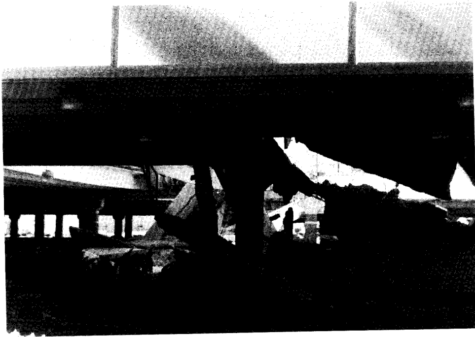
Figure 3.68. In precast parking garages, the support of the double-tees that comprise the floors is a vulnerable link in the system. This garage, at the north end of the Northridge Fashion Center, illustrates a common failure: the double-tees pulled off their supports, leaving the supporting elements essentially intact.
