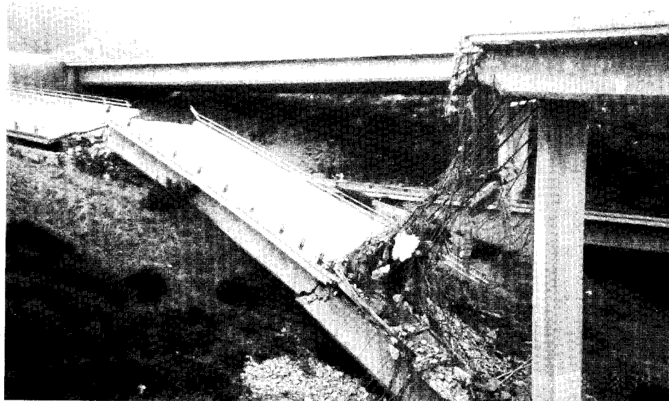
Figure 4.14. Collapsed portion of the SR14/I5 North Connector Overcrossing, looking east. Pier 2 was at the left, near the broken hinge on the ground (Photo courtesy of EERC).
