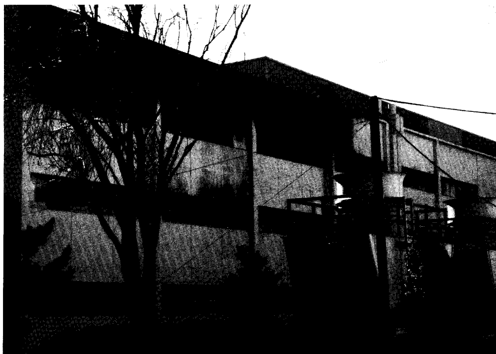
Figure 6.7. University science building damaged by fire.
