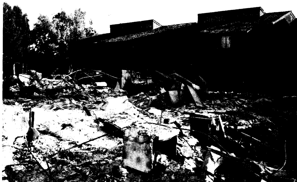
Figure 6.6. Multi-family residential building destroyed by fire.
