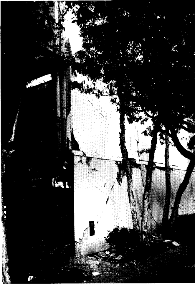
Figure 3.26. The Bay Vista Health Care Center was closed due to damage. Differential movement between the building and its base was indicated by the crack at the foundation line. The corner of the concrete foundation wall spalled, apparently due to crushing. A facade panel over the garage opening was dislodged.
