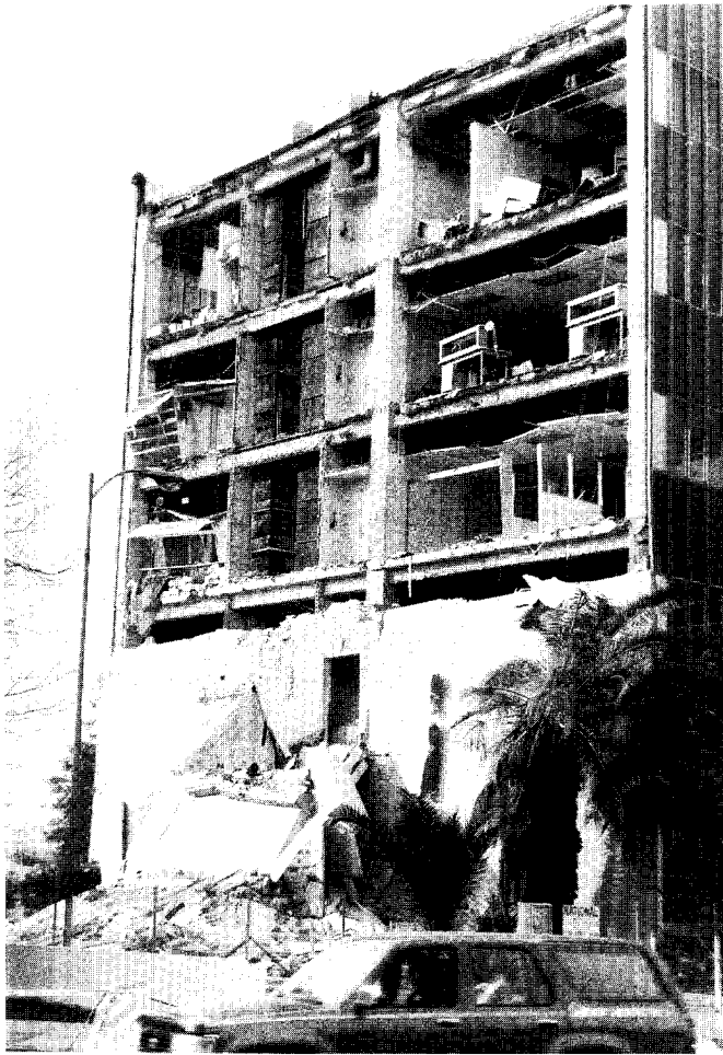
Figure 3.49. The east end wall and stair tower of a five-story apparently steel-framed office building on Sherman Way in Reseda collapsed. The enclosing masonry wall became detached from the structure and slid to the ground, with the upper stories remaining intact. The doorway opening in the wall, shown here resting at about the second story level, originally provided access from the top story to the stair tower.
