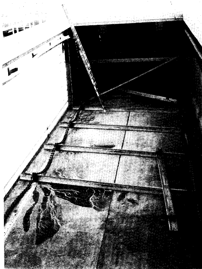
Figure 5.7. A damaged sludge scraper in a clarifier tank at the Tillman Water Reclamation Plant.
