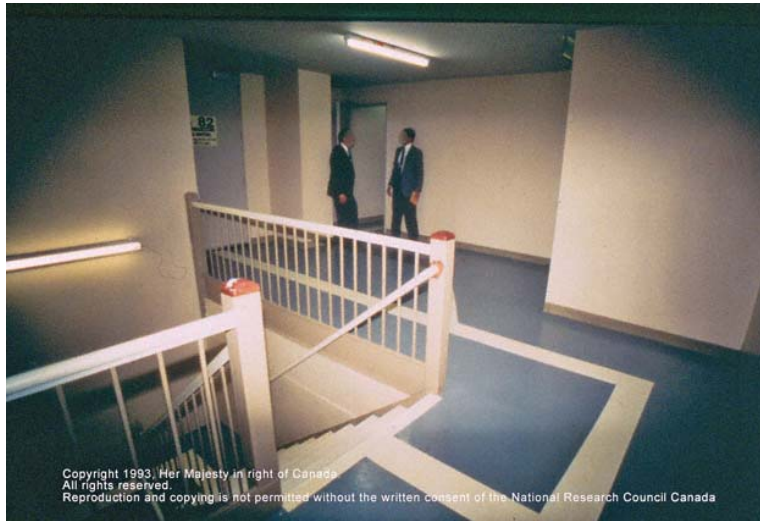
Figure 2-12. Horizontal transfer floors in the WTC towers.
