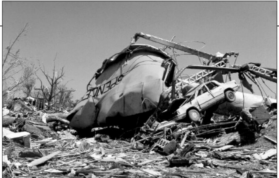
Collapsed steel water tower in Spencer, South Dakota due to the May 30, 1998 Spencer tornado.
