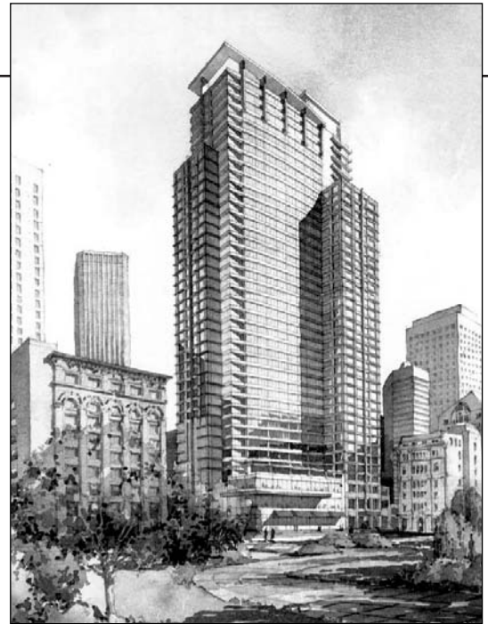
Thirty-nine-story precast concrete building in San Francisco.
