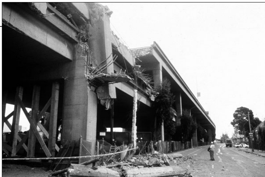
A failure of supporting columns resulted in the collapse of the bi-level I-880 Viaduct during the 1989 Loma Prieta Earthquake in the San Francisco area.
