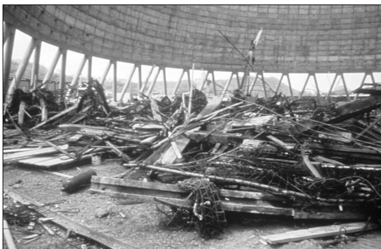
Collapse of a portion of a reinforced concrete hyperbolic cooling tower.
