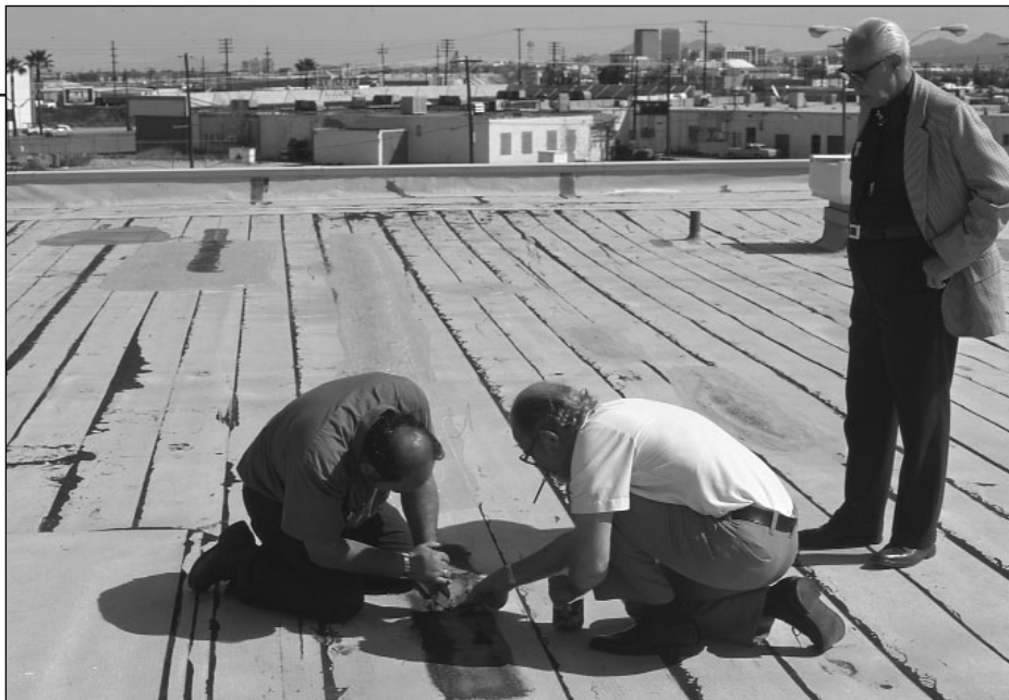
Sampling built-up-roofing membranes for measuring its performance properties.
