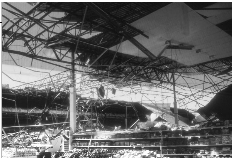
Structural damages to low-rise commercial and residential constructions caused by the 1997 Jarrel, Texas tornado included the partial collapse of the roof of a supermarket. The roof was supported by open-web steel trusses.
