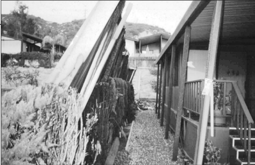
A collapsed carport shields a house from the adjacent structure that burned down completely.
