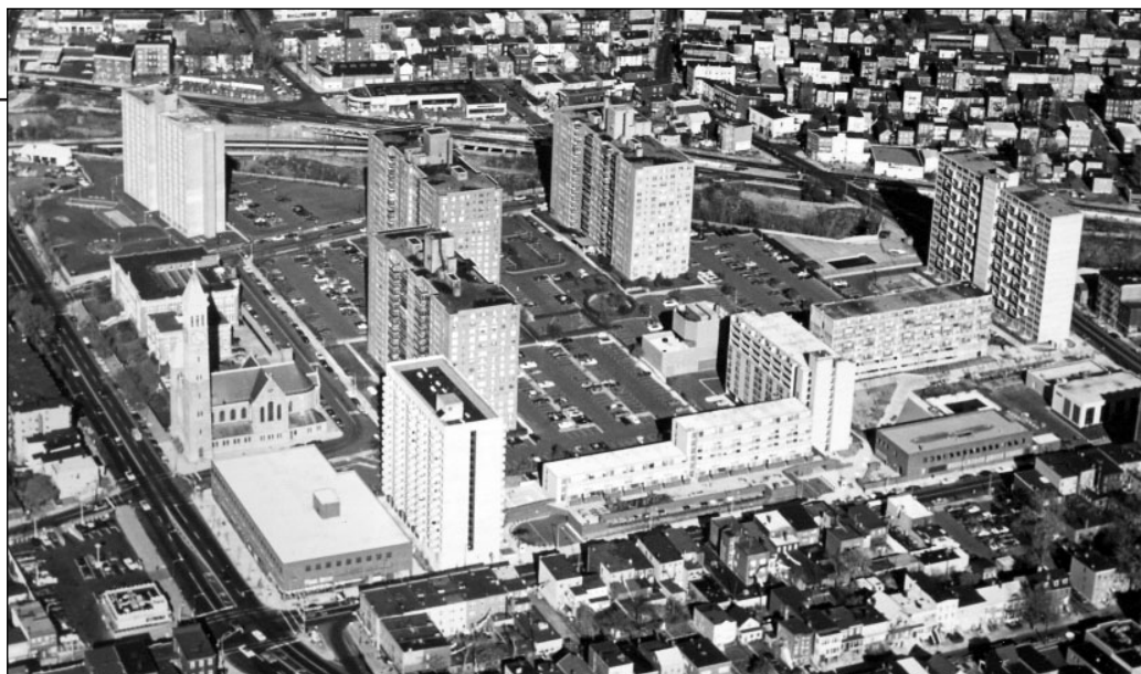
This Jersey City, NJ apartment building site of the mid 1970s featured use of prefabricated modules for medium-rise construction and an on-site energy cogeneration plant. NBS monitored the energy flow from the plant's electricity generated site recovery system including recovering heat from diesel generators that contributed to heating the building units. HUD was interested to know if the cogeneration design was energy efficient and worthy of replication.
