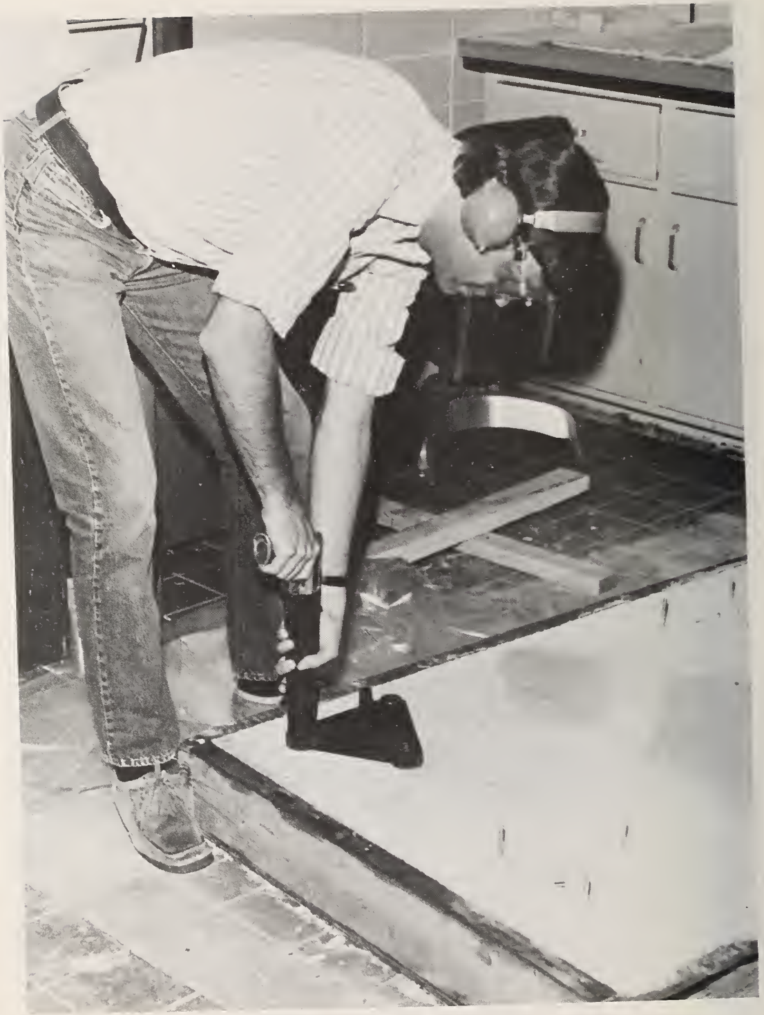
FIGURE 6 Probe Penetration Test
