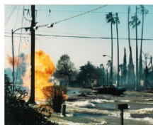
Photo: Balboa Blvd. 1994 Northridge Earthquake, damages to multiple lifelines (road, water, gas, electric power) - cascading failures and hazards
