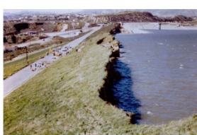
Lower San Fernando Dam – remains of crest after upstream slope failure – LADWP photo
