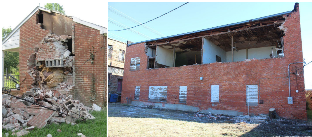
Figure 1-1 Examples of damage from recent moderate earthquakes in the CEUS. (a) Chimney collapse in the 2011 M5.8 Virginia Earthquake (from USGS). (b) Out-of-plane unreinforced masonry wall failure in the 2016 M5.8 Oklahoma Earthquake (from Ezra Jampole).
