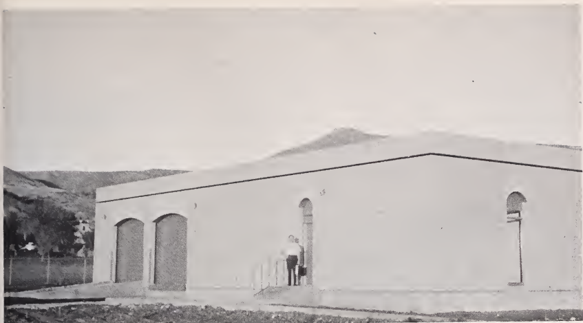
This is Idaho's new State weights and measures laboratory.
