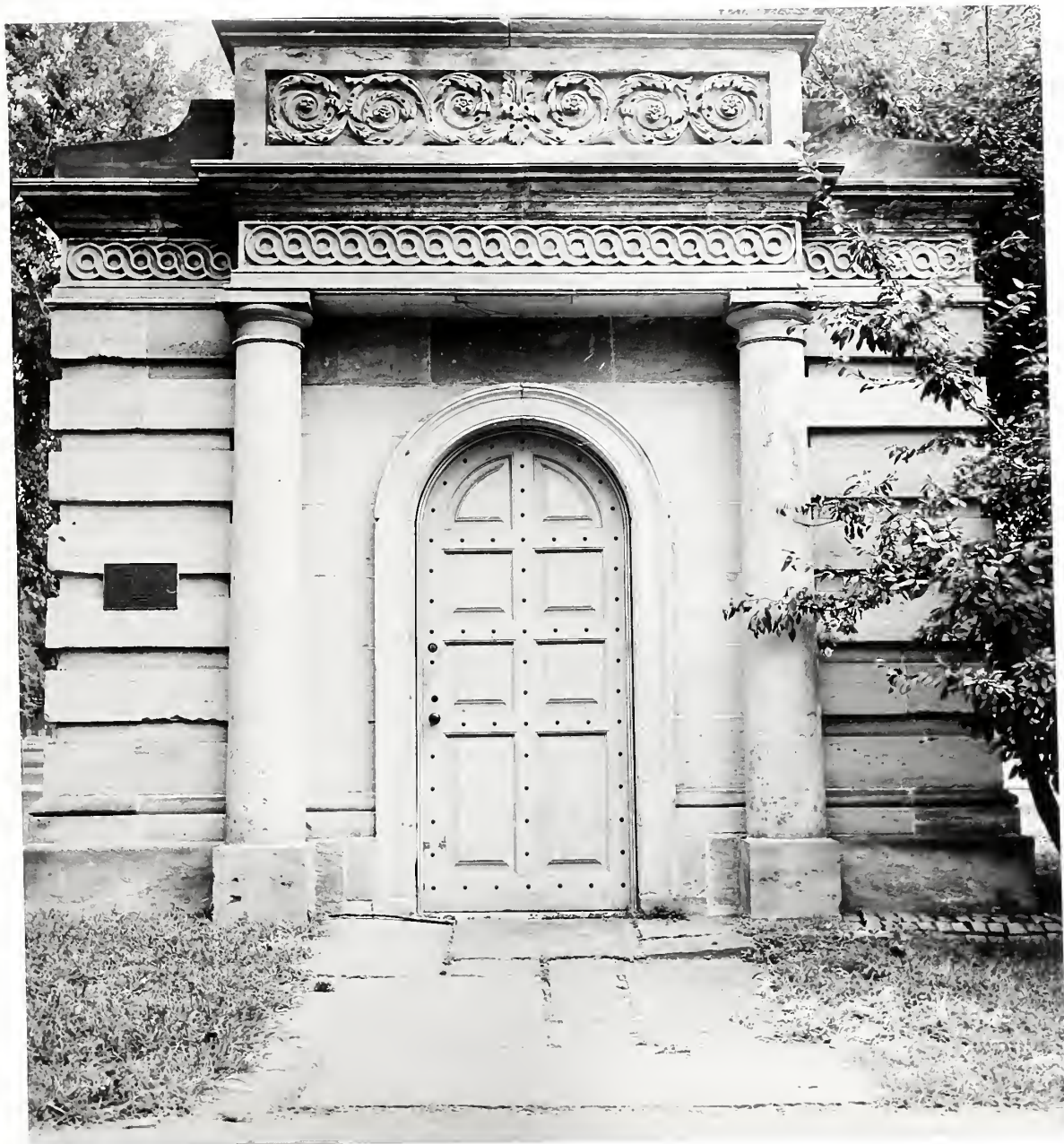
Fig. 7. View of Bulfinch gate house at Constitution Avenue and 17th Street, Washington, D. C. Photograph shows the excellent state of preservation of the unpainted Aquia Creek sandstone after about 125 years of exposure.
