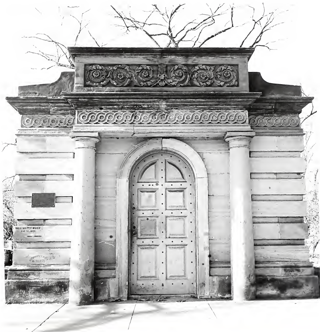
Fig. 8. View of Bulfinch gate house at Constitution Avenue and 15th Street, Washington, D. C. Photograph shows the excellent state of preservation of the unpainted Aquia Creek sandstone after about 125 years of exposure.
