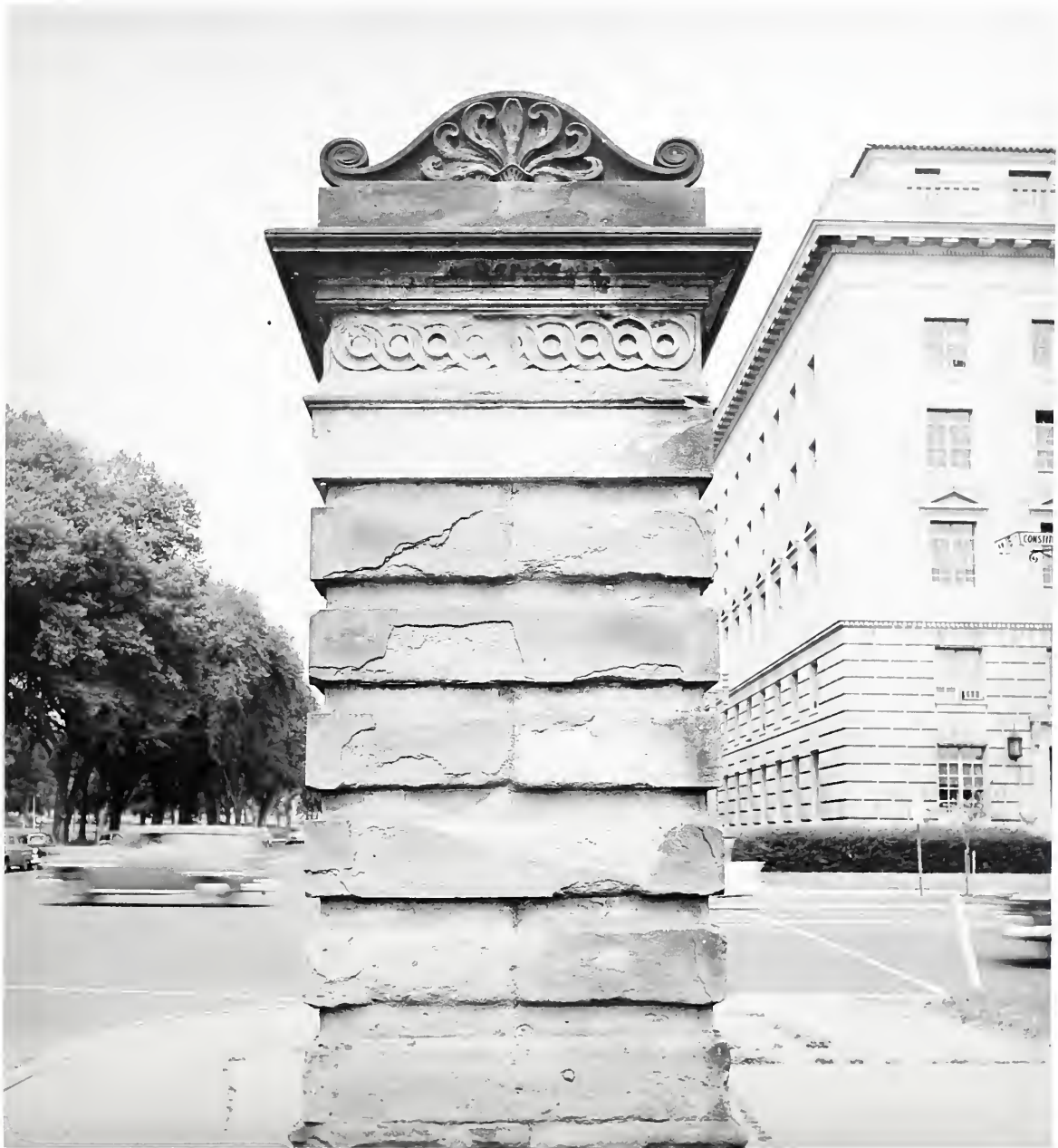
Fig. 10. View of gatepost at the southeast corner of Constitution Avenue and 15th Street, Washington, D. C. illustrating the advanced state of disintegration of unpainted Aquia Creek sandstone after about 125 years of exposure.
