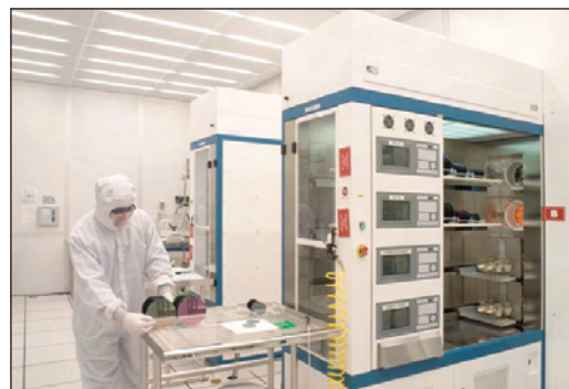
Figure 2. Oxidation and annealing furnaces banks.
