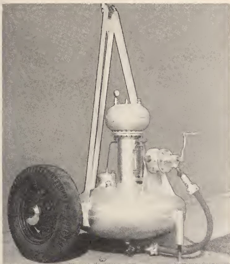
FIGURE 8. Volumetric-type LPG-meter prover—County of Tulare, Calif.
